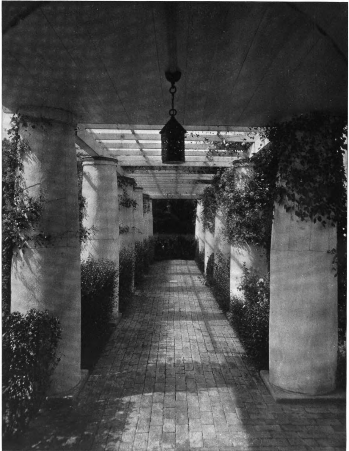
THE PERGOLA FROM THE PORCH
