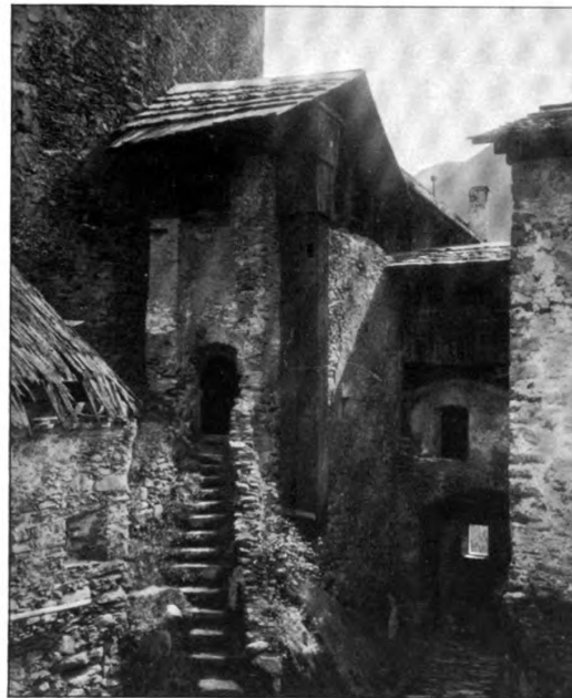
A RUINED STAIRWAY AT TAUFERS
