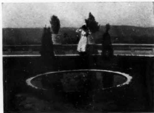
THE PARAPET AT THE WEST
