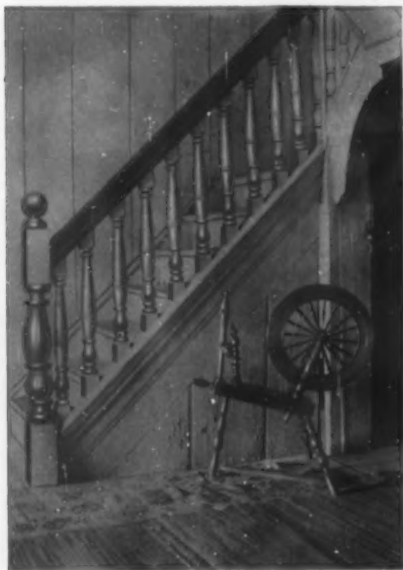
STAIRWAY AND DOOR
