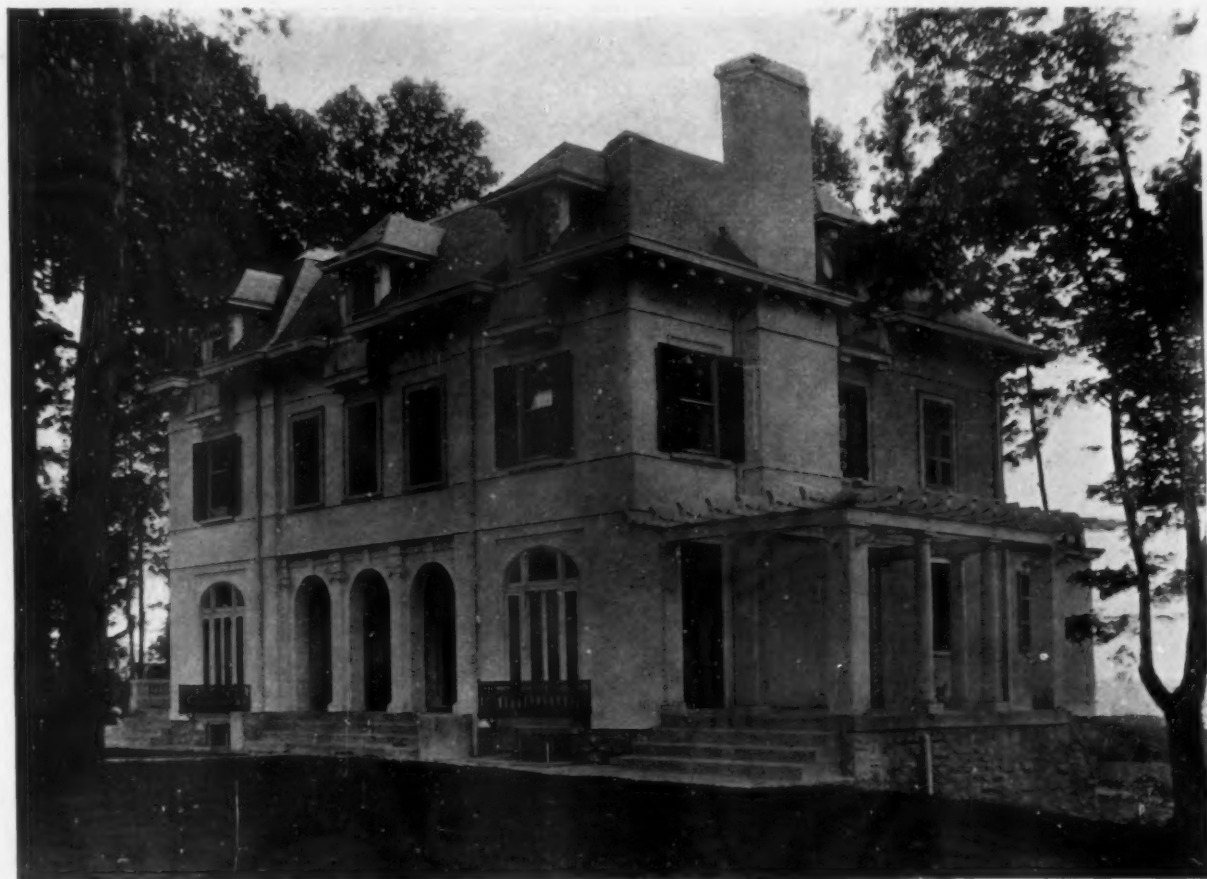
THE RESIDENCE OF A. C. MEYER, ESQ.
