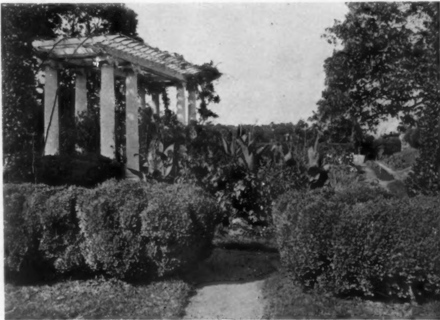
AN APPROACH TO THE PERGOLA
