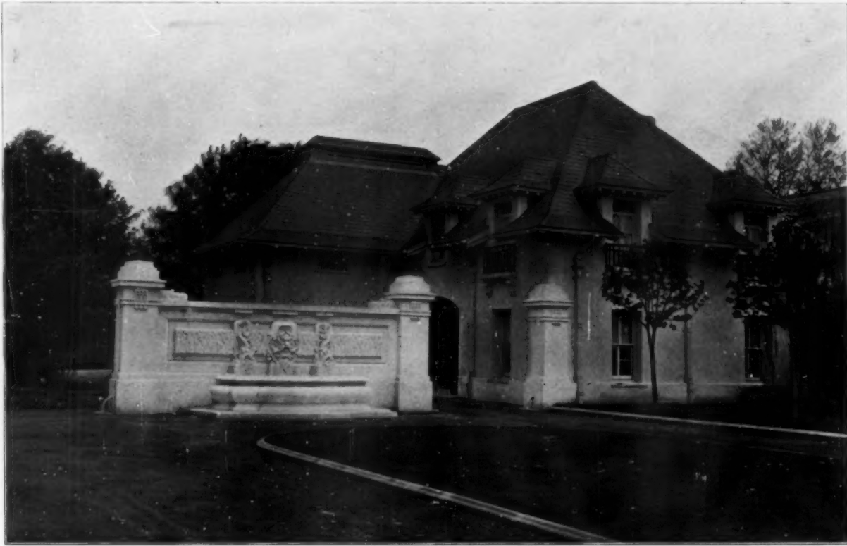
THE ENTRANCE TO THE STABLES FROM THE FORECOURT
