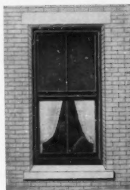
Our sliding sashes can be made to pivot to permit cleaning from inside of building if desired.
