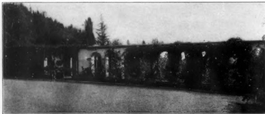
The Colonnade Overlooking the Pool
