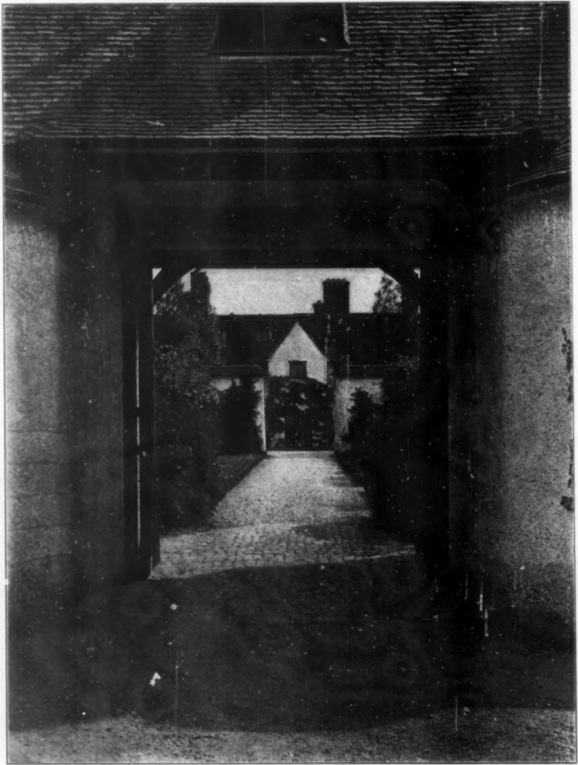
A VIEW THROUGH THE GATE HOUSE BERRYDOWN COURT
