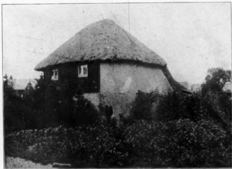
A WEATHER-BOARDED COT AT HERNE BAY, KENT
