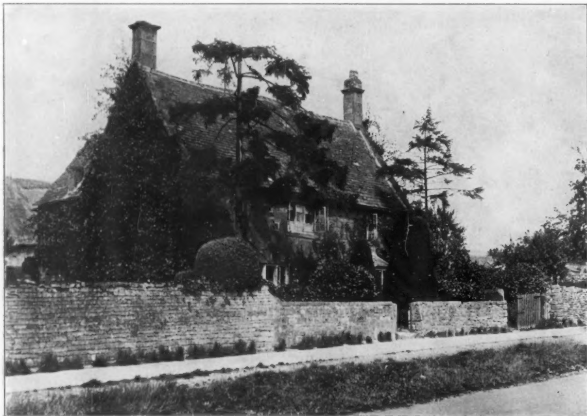
AN OLD HOUSE AT BROADWAY
