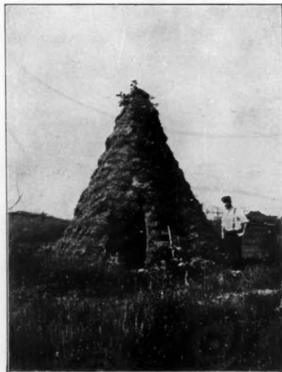
TYPE OF MUD-AND-STRAW HOUSE
