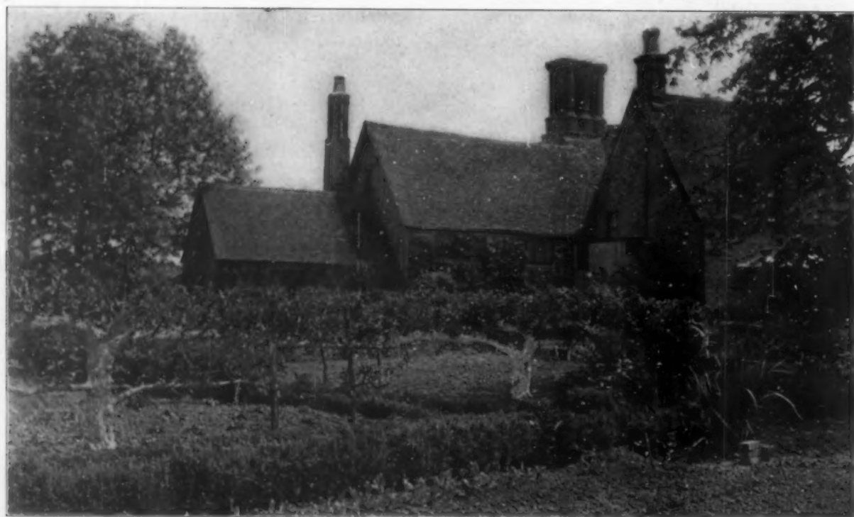
A HADLOW COTTAGE
