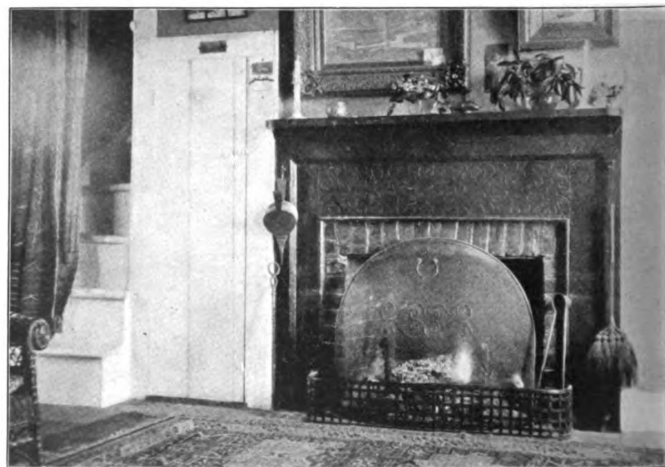
THE LIVING-ROOM FIREPLACE
