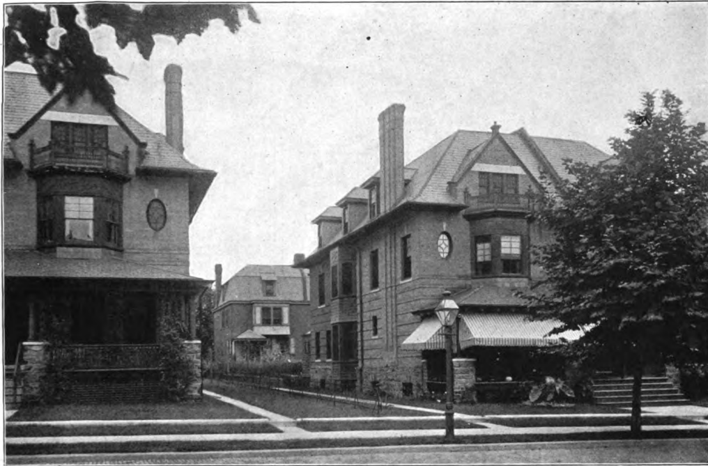
These houses are about thirty feet apart, which is a reasonable minimum distance
