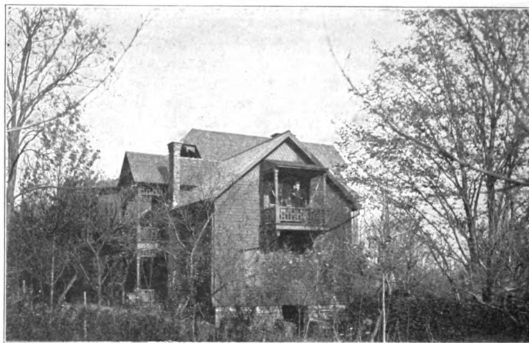
A SECOND STOREY BALCONY
