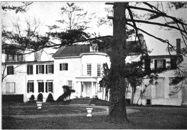
THE ENTRANCE FROM THE WEST
