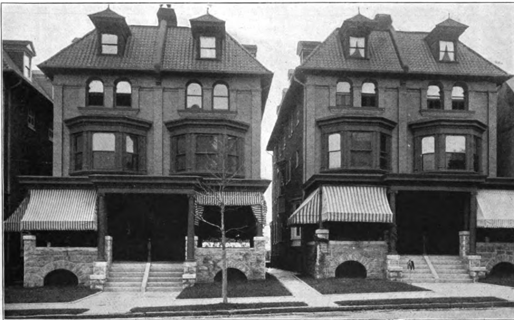
There are fifteen windows in the side wall of each of these houses which are less than eight feet distant from fifteen similar windows placed exactly opposite in the adjoining house
