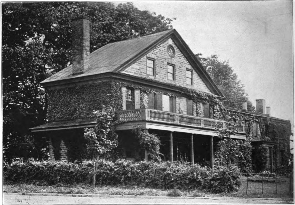
WHITBY HALL FROM THE SOUTHWEST
