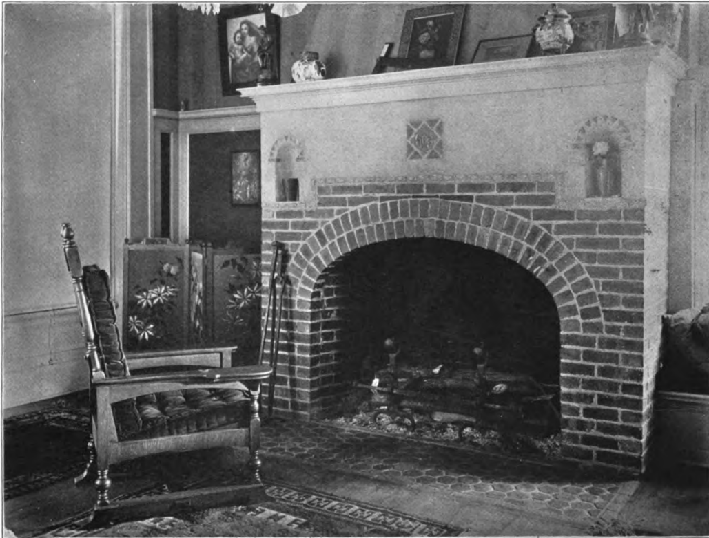
ROUGH BRICK FIREPLACE WITH TILE INLAIS IN PLASTER
