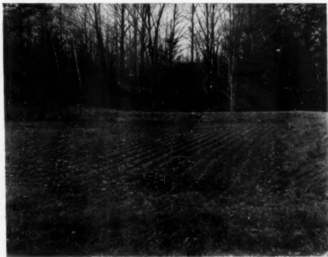
Bed of Sand Five Feet in Depth, formerly Relied upon for Purifying Crude Sewage. Now Employed for Filtering Oxidized Sewage Water
