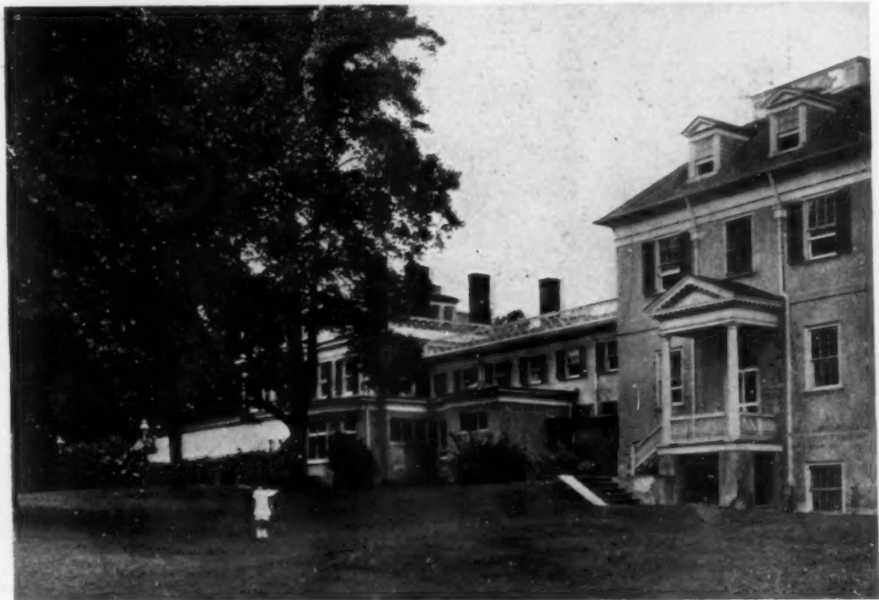
THE CLUB HOUSE FROM THE REAR
