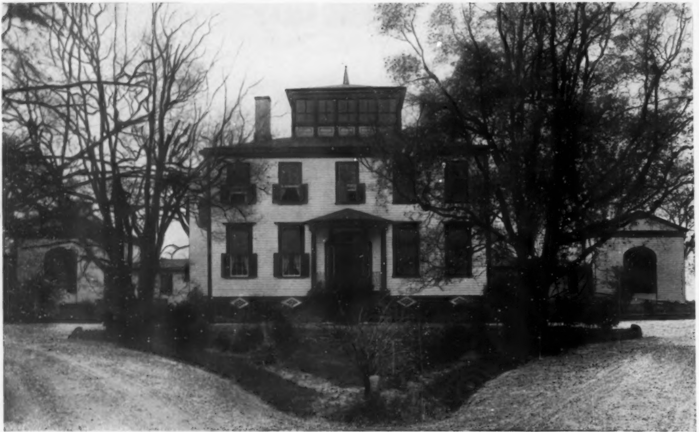
THE NORTH FRONT AND DRIVEWAY—"HAYES"
