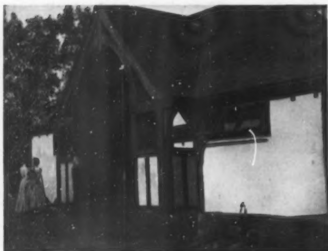
STABLE ENTRANCE, CORNWALL-ON-HUDSON, N. Y. Taylor & Levi, Architects
