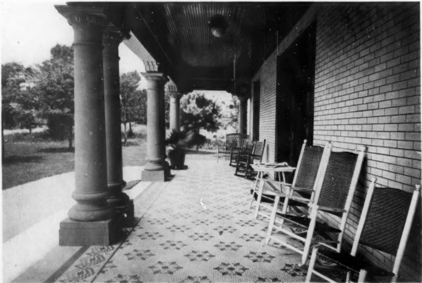
AN ATTRACTIVE PORCH FLOOR OF TILE
