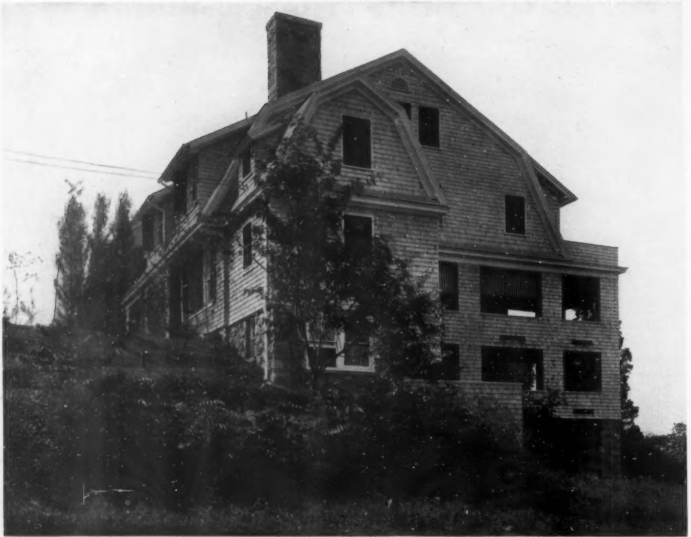
A SIDE VIEW, SHOWING AMOUNT OF SPACE GAINED BY THE CONTOUR OF SITE
