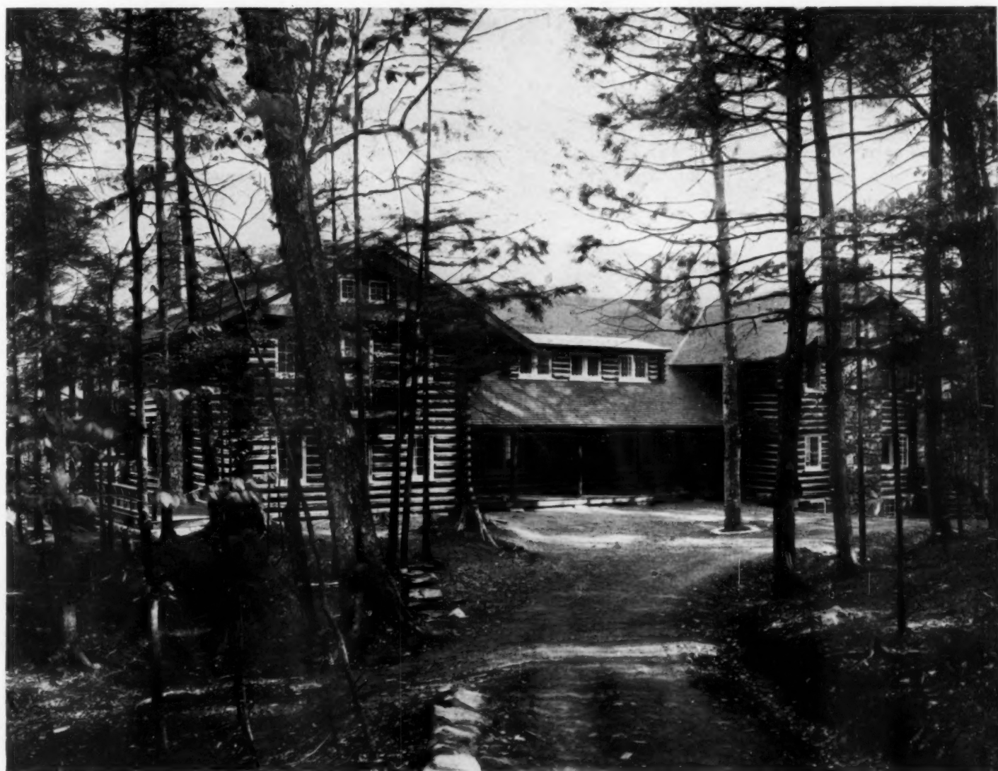
THE LODGE AS SEEN FROM THE REAR APPROACH
