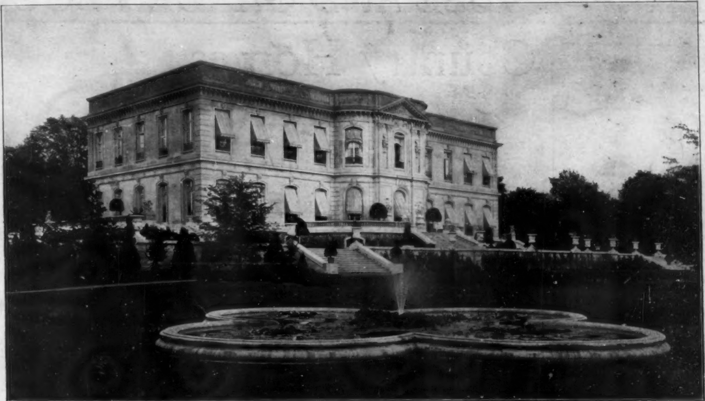
Residence of E. J. Berwind, Newport, R. I. Horace Trumbauer, Arch. Equipped with Loomis-Manning Filters
