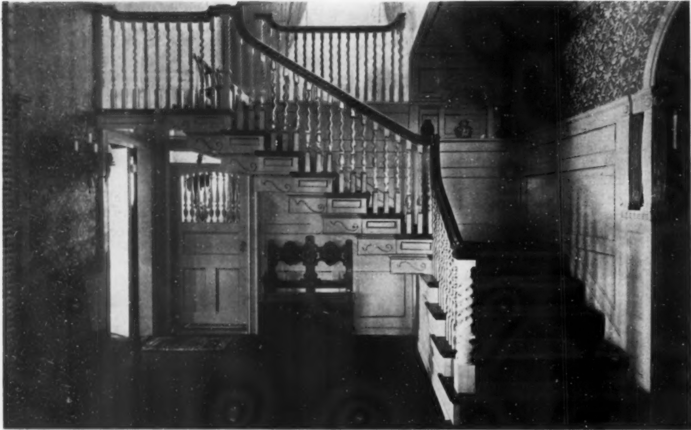
FIRST FLOOR, COLONIAL HALL, NO. 2, SALEM, MASSACHUSETTS
