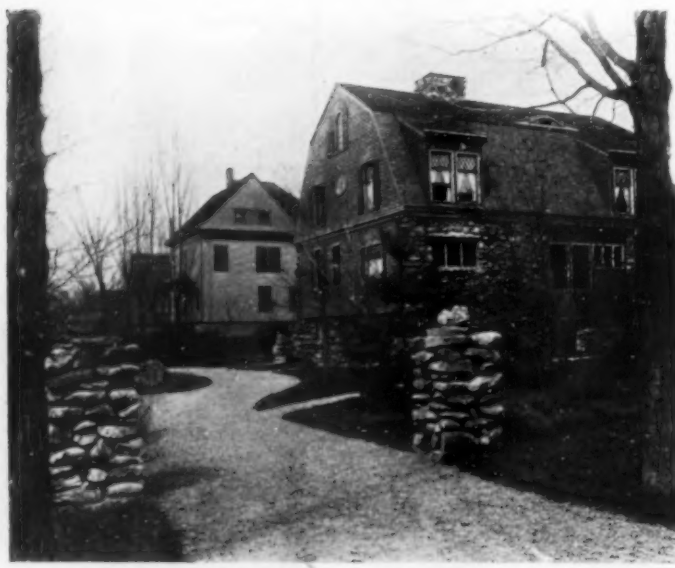
"THE MANSE" FROM THE SOUTH AND WEST
