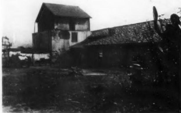
BACK COURT SHOWING OLD STORE HOUSE
