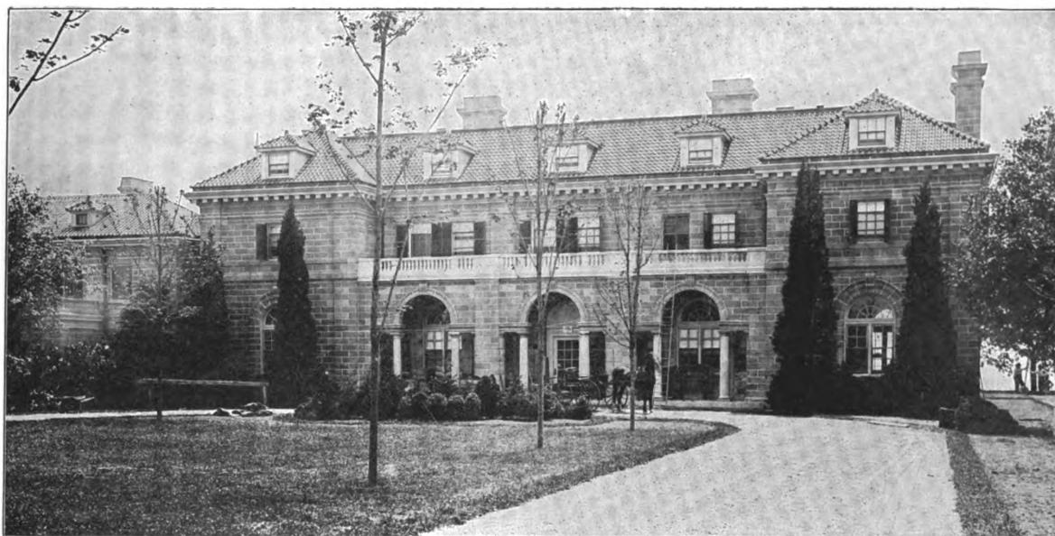
A Residence the Walls and Partitions of which are of the "Two-Piece" Hollow Concrete System
