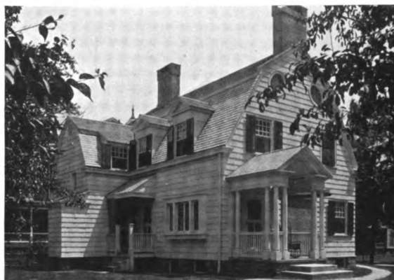
Side and Rear View
