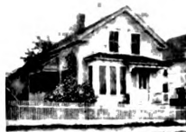
A No. 3015 IDEAL Boiler and 175 ft. of 3/8-in. AMERICAN Radiators, costing the owner $118, were used to Steam heat this cottage.
