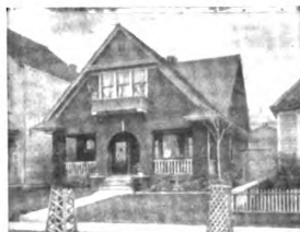
A No. 17-3-W IDEAL Boiler and 300 ft. of 38-in. AMERICAN Radiators, costing the owner $150, were used to Hot-Water heat this cottage.
