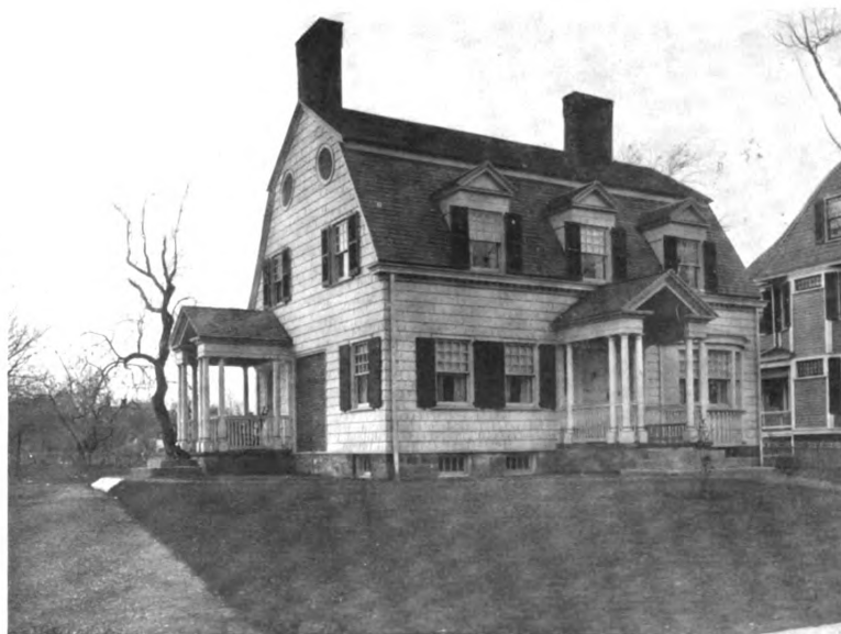
Front View of the Cottage
