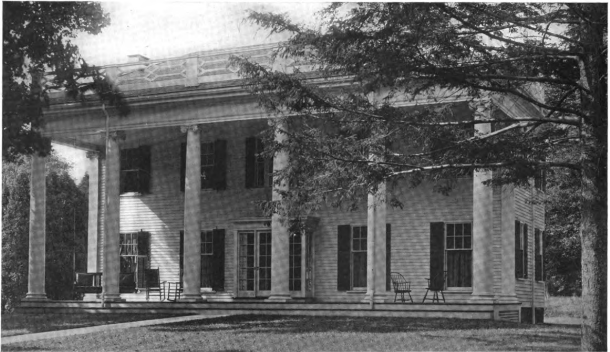
THE HOUSE FROM THE FRONT
