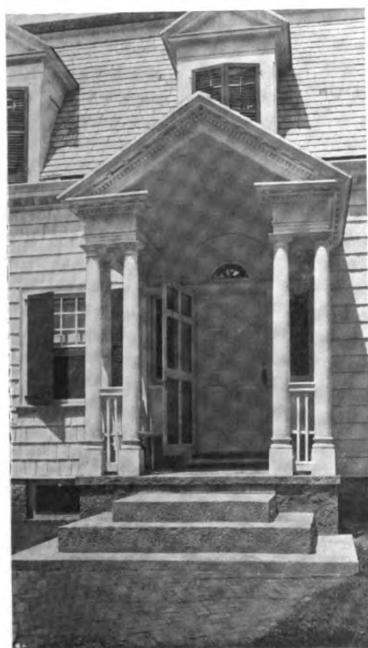
Detail of Entrance
