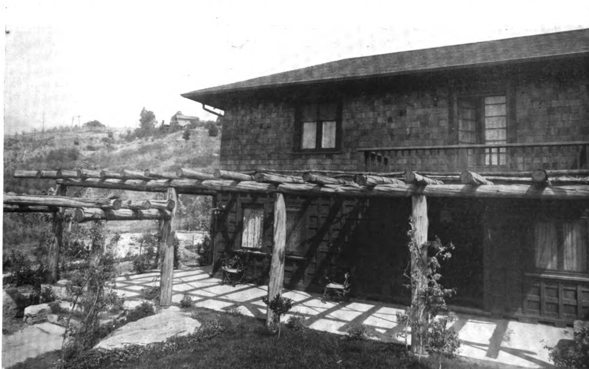
THE FRONT OF CHARLES PERCY AUSTIN'S SANTA BARBARA HOUSE
