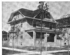
A No. 3-22 IDEAL Boiler and 400 ft. of 38-in. AMERICAN Radiators, costing the owner $205, were used to Hot-Water heat this cottage.
