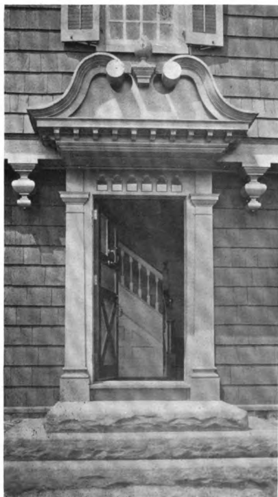
Detail of Entrance
