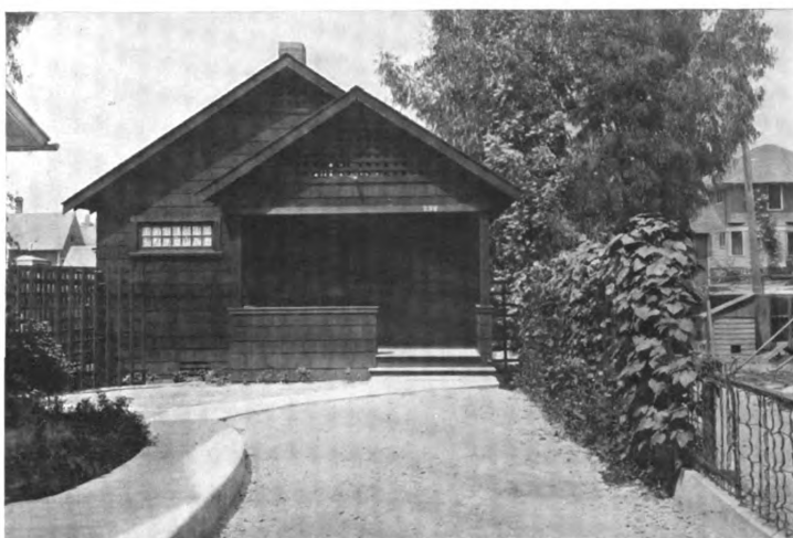
Cost $1,200. Five rooms and bath. Brick fireplace. Panel finish inside. Shakes outside. Rents unfurnished for $25 per month by the year
