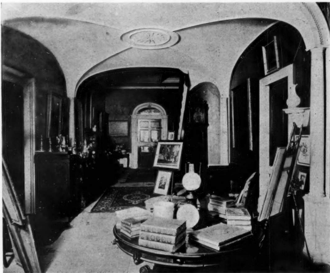
THE GROINED CEILING IS WELL DEFINED HERE
