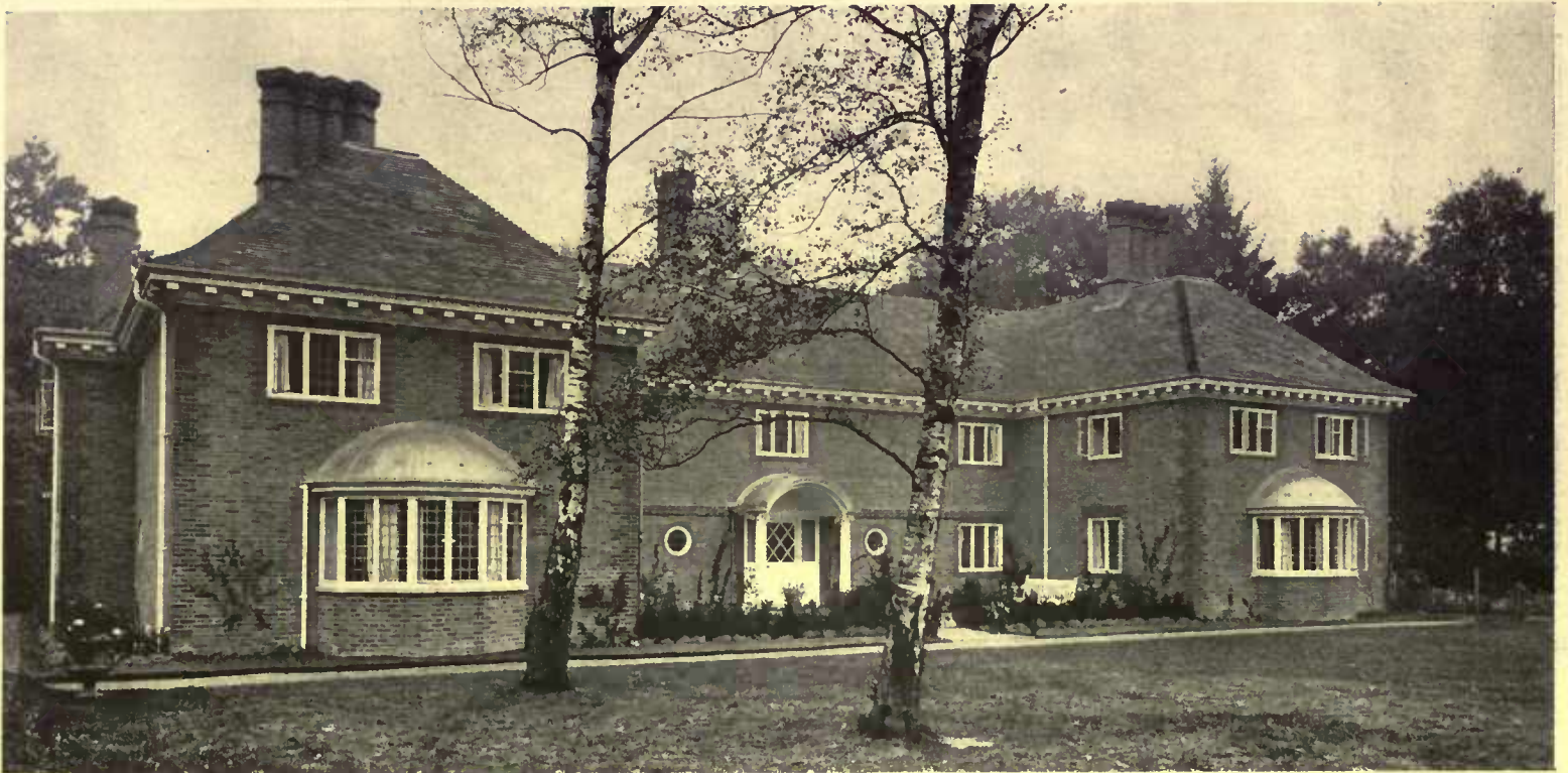
The house appears large, but is in reality not of such great area in floor plan. The cross-bar of the H is but 18 ft. in depth
