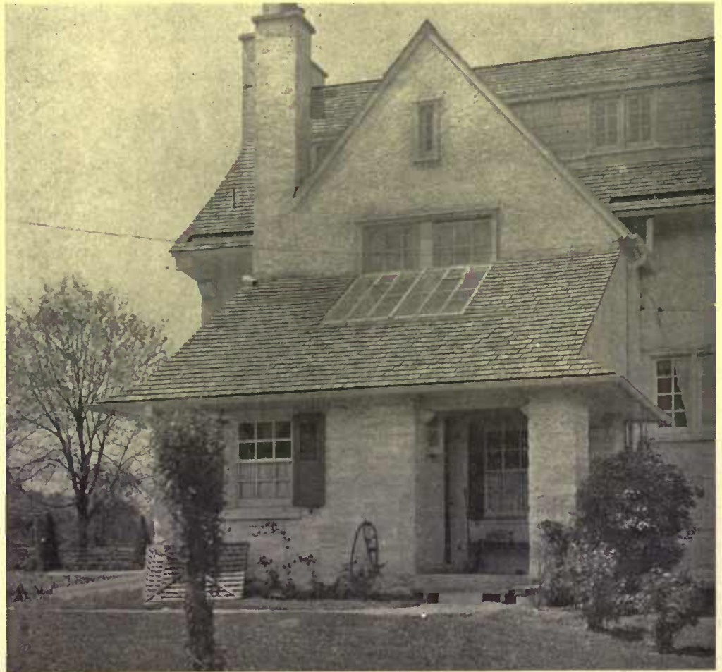
How one home-owner solved the problem of securing an effective and unobtrusive place for raising seedlings in the early spring. Unfortunately, not many houses have a roof of this form, but perhaps there is some other place about your own home in which you can build a garden under glass
