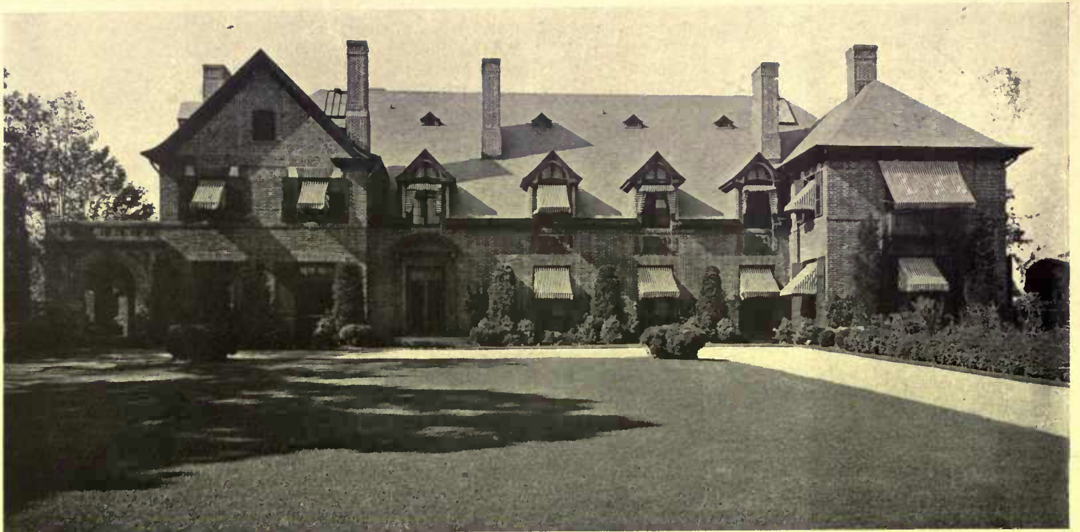
We in America are just beginning to realize that there are wonderful possibilities in the ornamental treatment of brick walls. In this country home at Oyster Bay a rough-textured brick of peculiar shape has been used with great variety in bonding. Carrère & Hastings, architects
