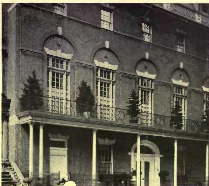
The Colony Club, New York—an example of the patterned surface and also of the value of countersunk areas in a brick wall surface. McKim, Mead & White, architects
