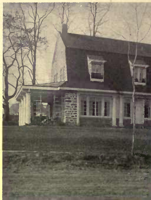
Compare the barren, cold appearance of this newly built house with the later picture of the same place a few months later
