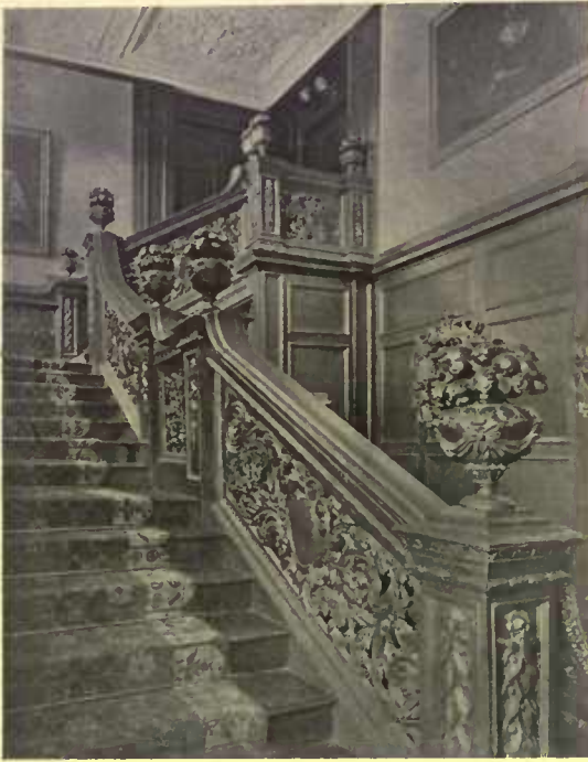
Carved and pierced detail in stair-rail of Forde Abbey, Dorsetshire—a form of decoration permitting the sumptuous adornment of both sides
