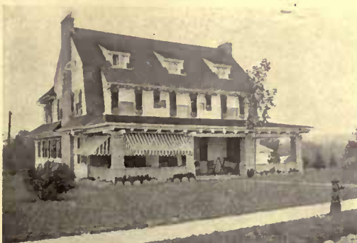
A house at Plandome that is a modern adaptation of Dutch Colonial
