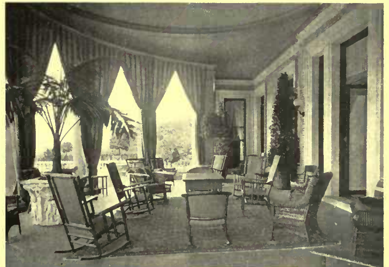
Projecting awnings would be awkward on the exterior of this curved porch; curtains of awning material solve the difficulty
