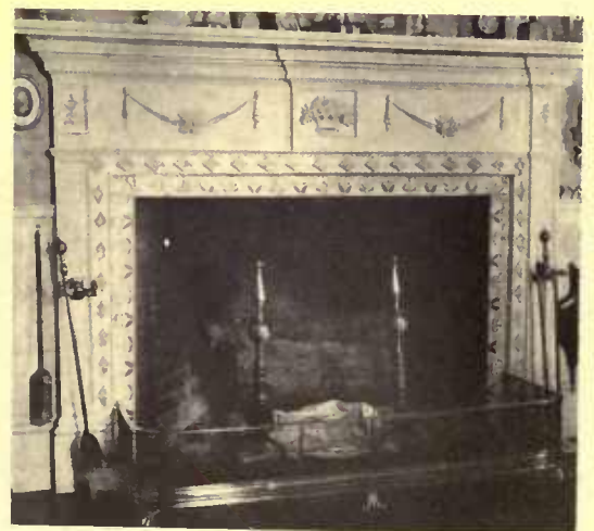
The use of baskets of fruit and other applied ornament in frieze panels over the pilasters or columns was a characteristic of Colonial doorways and mantels
