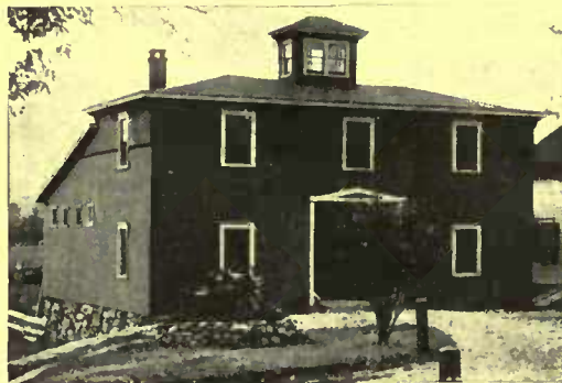
Here is a good seven-stall barn that could be turned into a garage
