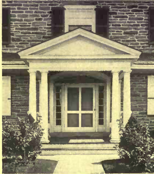
Quarry-faced course rubble, in which type an approximately horizontal line is formed with each course
