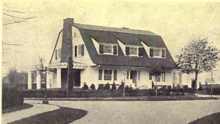
One of the new houses at Kensington—another adaptation of the Dutch Colonial to modern needs. Forman & Light, architects
