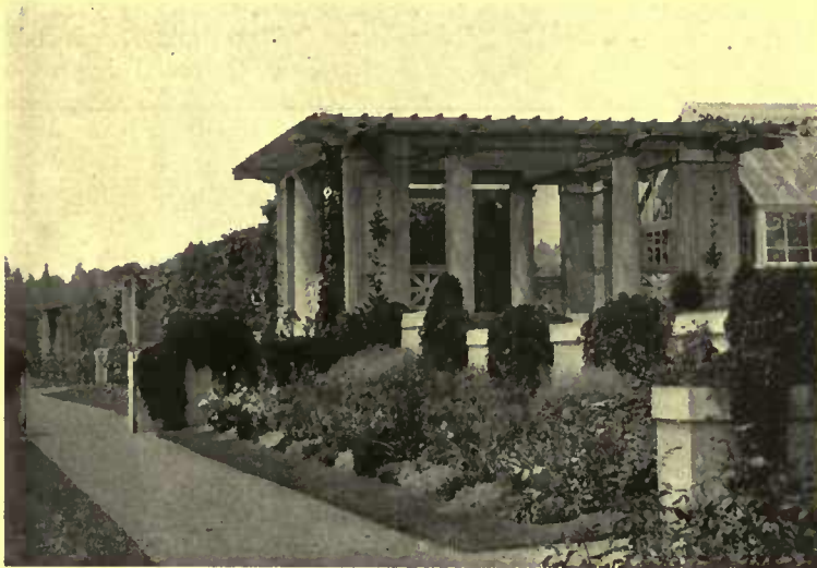
Too frequently we see concrete pergolas of crude form. Greater care and skill in making the molds will work wonders
