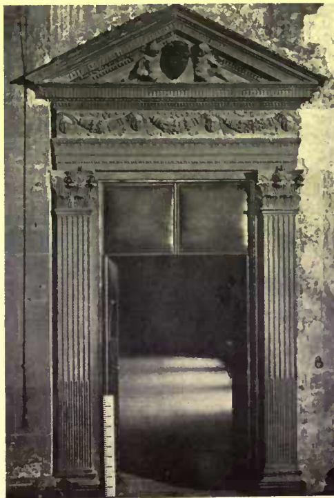
The garlands and heads in the frieze are typical, as is the reeding of the pilasters
