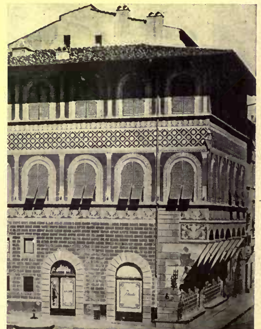
An example of sgraffito work—the top coat of light plaster is scratched away in parts to show the darker color below
