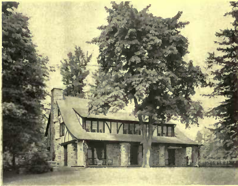
A country home at Pleasantville, N. Y., William A. Bates, architect. There is an interesting and unusual use of stonework in the circular columns supporting the wide overhang
