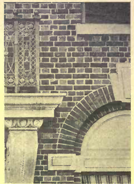
English bond—alternate rows of headers and stretchers, with joints of the latter over one another
