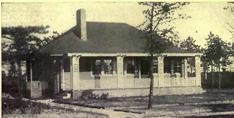
A simple bungalow of stucco at Brightwaters, Bayshore, L. I., with distinctive latticework columns for the porch roof supports.
