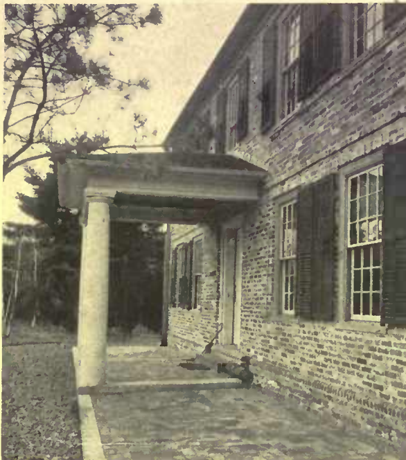
An interesting texture is obtained here with second-hand brick, from which the old mortar has not been fully cleaned. Philip B. Howard, architect
