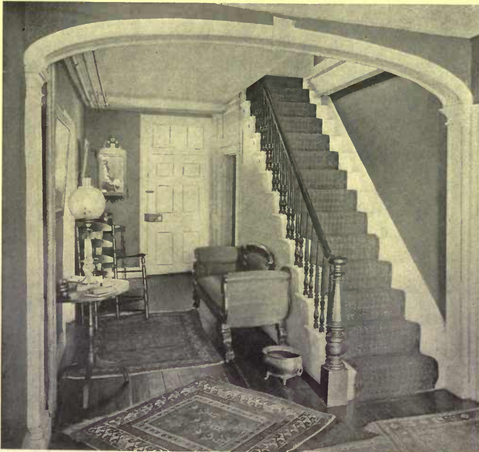
Originally the walls of the hall were probably finished in tinted or sanded plaster only. Papering was rarely found excepting in important formal rooms
