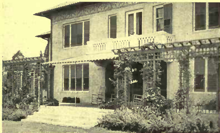
The frieze protected by the deep overhang of the roof was secured by stenciling with cement washes in subdued colors. Louis Boynton, architect
