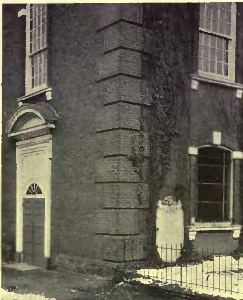
Corner block-like projections of this kind are called quoins. The motive is derived from stone work. St. Peter's, Philadelphia
