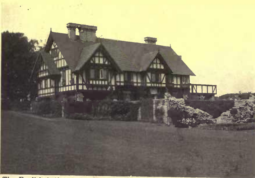
The English half-timber house as usually built in this country is merely a plaster house covered with wooden strips in a pattern. Here, however, the timbers are a structural part of the wall. Oswald C. Hering, architect
