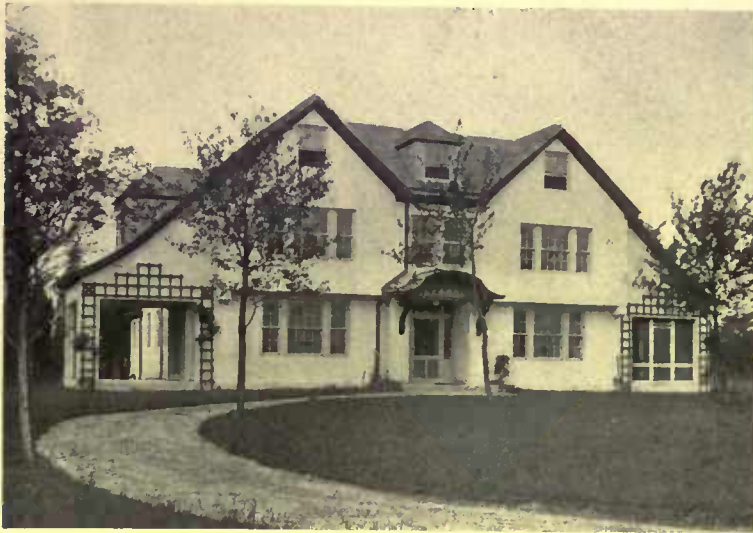
The house is of stucco on a wood frame. This use of two gables on the front is seen in many of the modern English homes, and there as here the bringing down of the roof lines at the ends helps greatly in tying the building to its site
