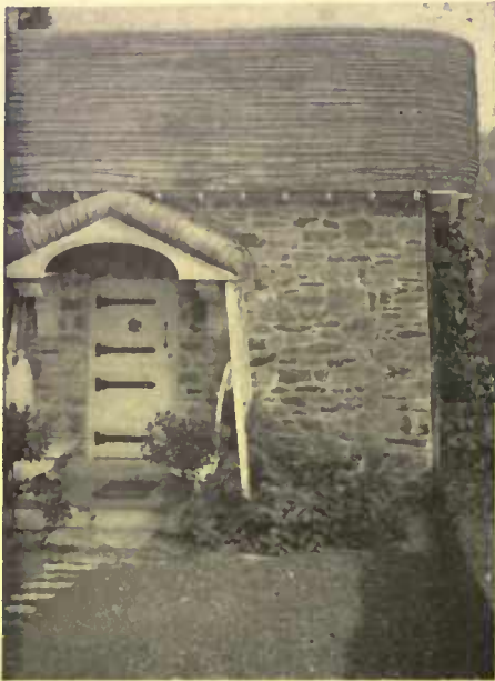
Random rubble of stone that has been left with its face as quarried. Donald C. Hering, architect
