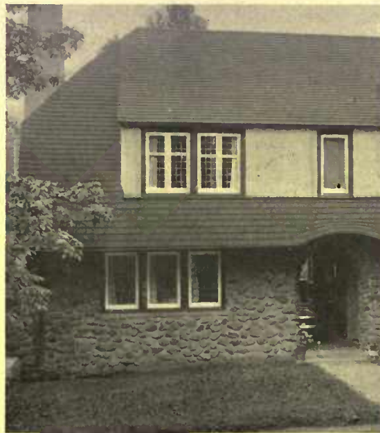
This cobble wall has had its joints raked out to give rougher texture to the surface and to gain strong shadows
