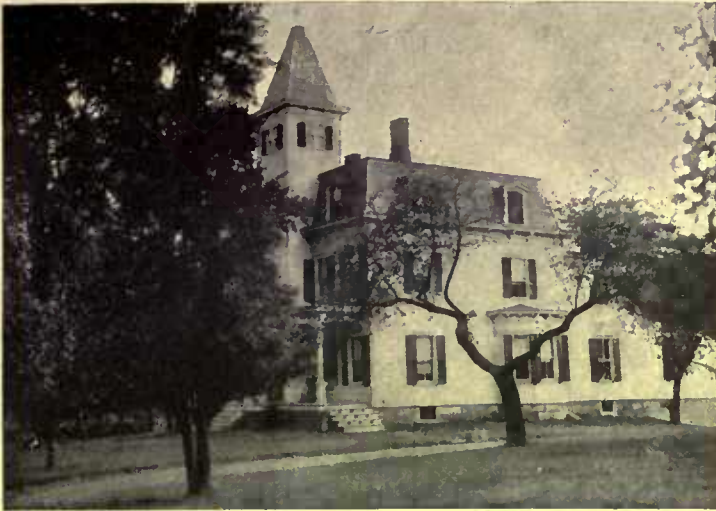
Here is the house as it stands to-day—substantially built and well adapted for remodeling
