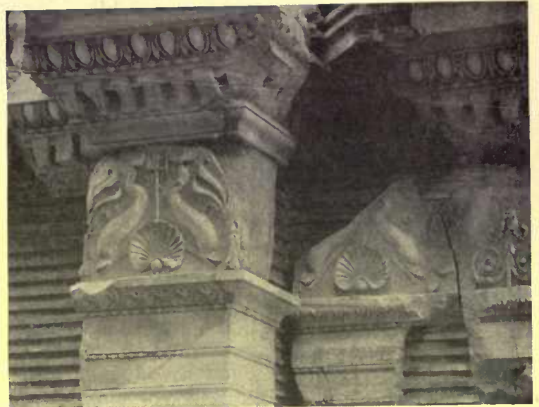
A classic stone fragment. The egg-and-dart molding appears at the top, with the bead-and-reel and a dentil course below it, the latter badly broken
