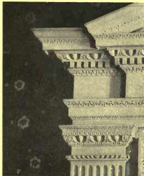
A bit of an interior doorway carved by the Colonial craftsman builders. There are several variations of the lamb's-tongue molding here
