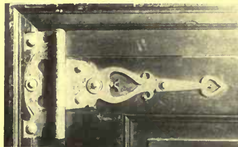
A closet hinge cut by Mr. Maxfield Parrish from a common strap hinge of brass—a practical suggestion for the amateur craftsman
