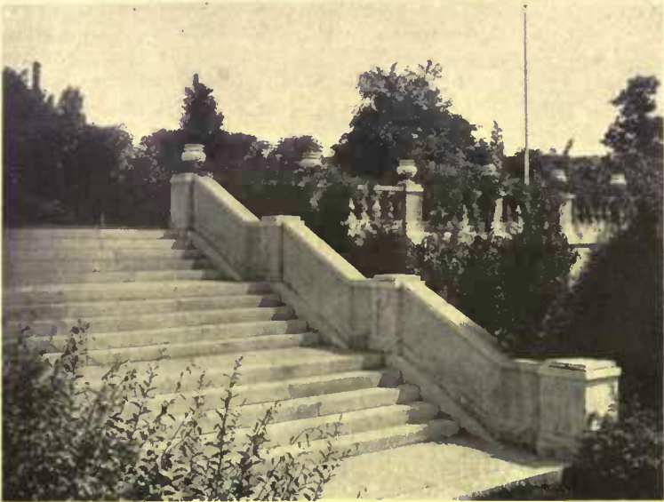
Garden steps of stone are expensive, those of brick are difficult to keep in repair, but those of concrete, if designed with some skill, have neither of these disadvantages
