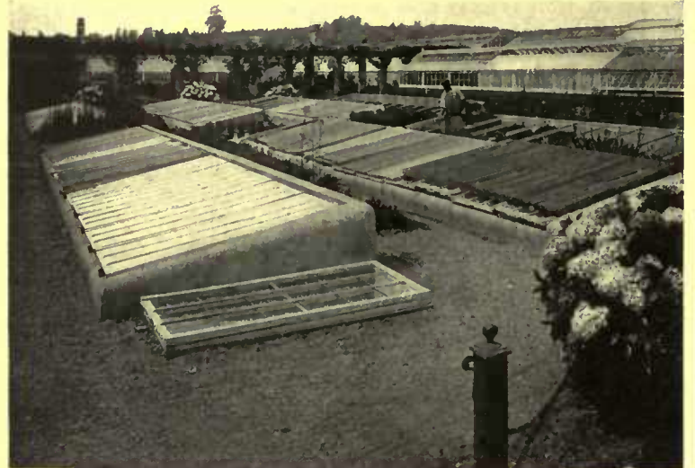
The decay and warping of wooden hotbeds and coldframes is a common fault. Concrete frames will last forever
