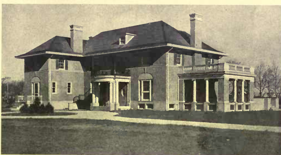
The smooth cement base, belt course below the second-story windows, and the recessed panels below the arches, give the house its character. O. C. Hering, architect
