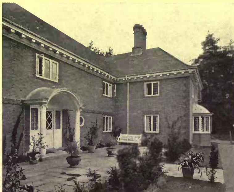
The walls are of vari-colored “clamp” brick from Chichester, with deep red bricks at the corners, around openings and in the belt course
