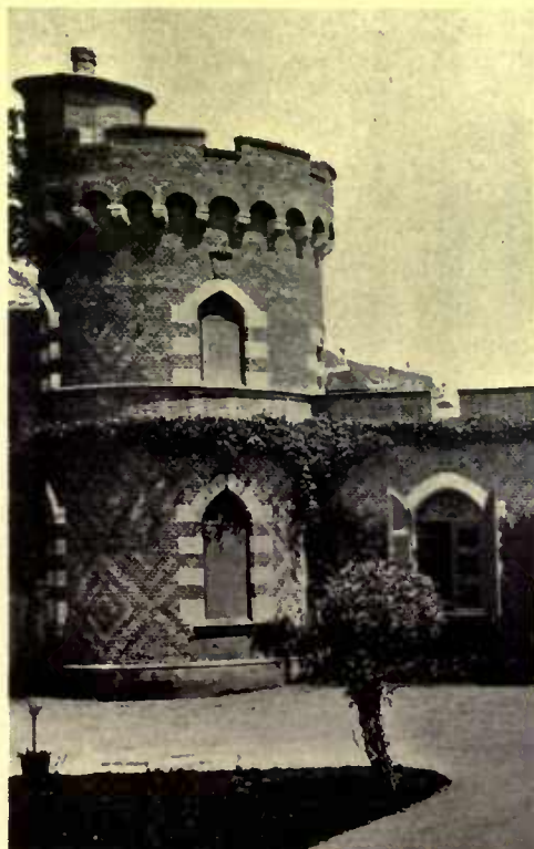
The hunting lodge of Moulemont, France. An example of the diaper pattern obtainable by different hued brick
