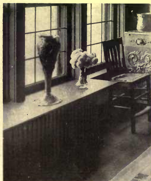
A projection of the window-sill throws into semi-obscurity this dining-room radiator
