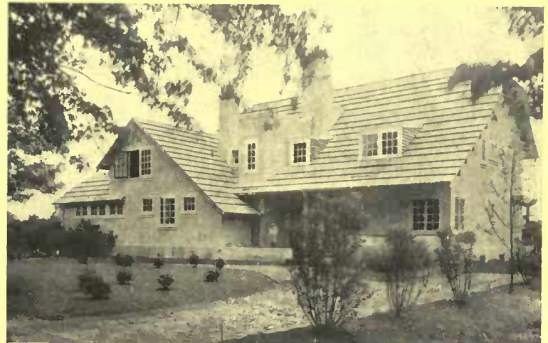
Shingles have been used here for the roof, doubled every fourth course, but tile or slate are more common in the fireproof type.
