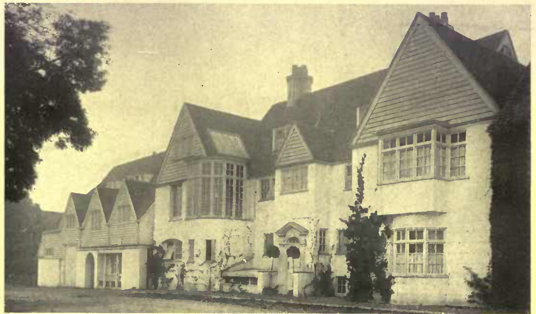
An English scheme for embellishing the surface of a stucco wall is to cover it with a network of wires on small iron posts, not unlike heavy iron nails, on which the vines are trained
