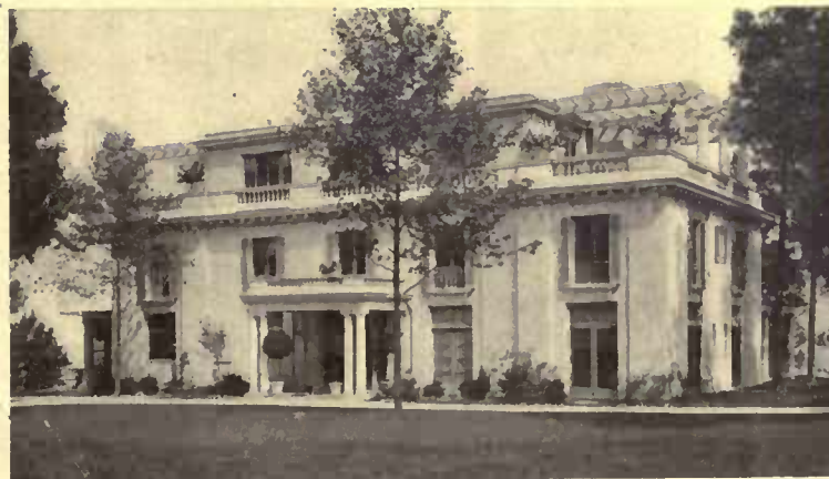
Where the design will permit a flat roof, this is made fireproof at a lower cost than a sloping one
