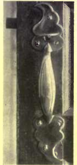
An old thumb-latch and handle secured by hand-wrought nails
