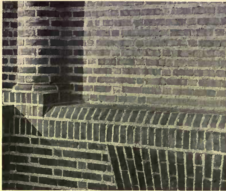
Double-stretcher Flemish bond as used in an interesting example of good brickwork—the University of Pennsylvania Museum
