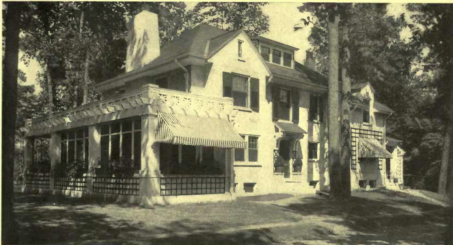
An objection sometimes heard regarding the fireproof house is that it is too plain to be attractive. The Holden house, at South Orange, N. J.—Hollingsworth & Bragdon, architects, shows that this is by no means a necessary fault
