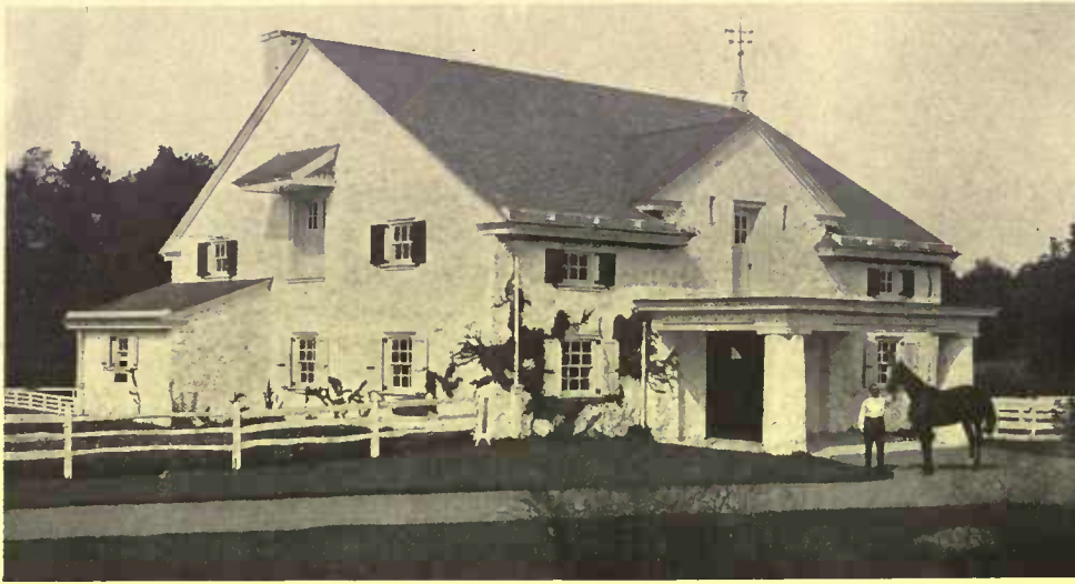
Another treatment of a stone wall where the stonework cannot stand on its own merits is to give it a very thin coat of stucco. Duhring, Okie & Ziegler, architects
