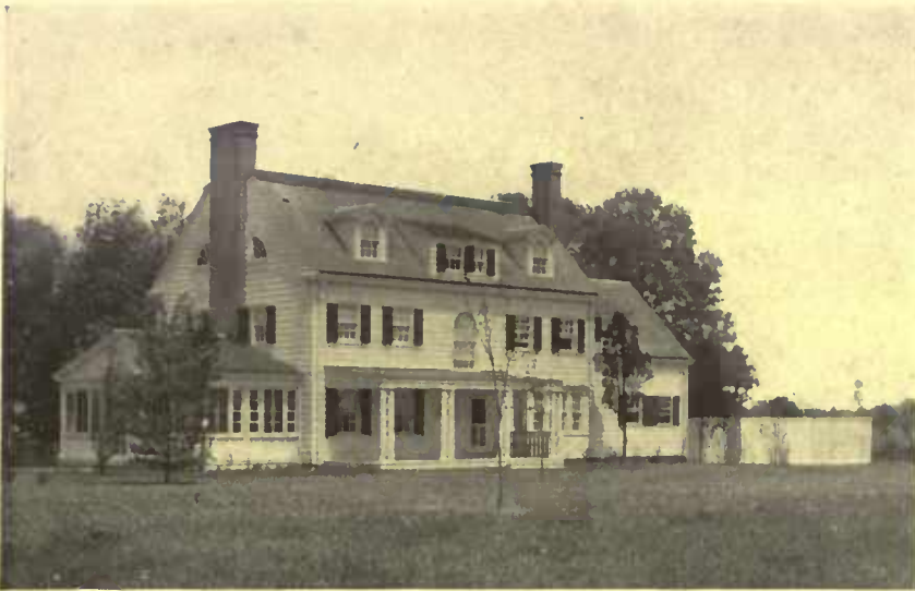
A modern Colonial house of clapboards on Long Island. With the exception of the gambrel roof this is a fairly representative example of the New England Colonial type. J. Acker Hayes, architect
