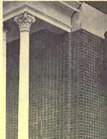
The startling bond used in the Colony Club, New York City, McKim, Mead & White, architects. Such a bond would be impossible without the aid of modern cement mortar, as there is no breaking of joints in the courses excepting at the corners
