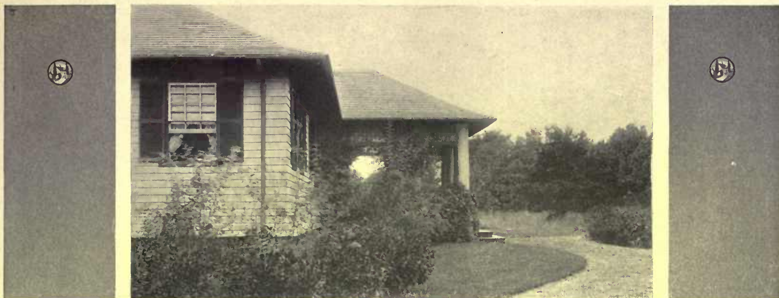
The broad overhang of the roof gives a deep shadow that is essential in a summer home not protected by large shade trees
