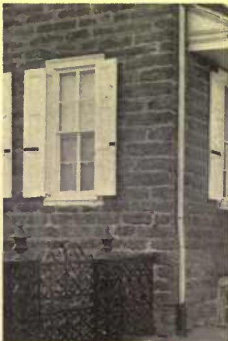
Regular course ashlar—stones squared up and laid with regular horizontal joints
