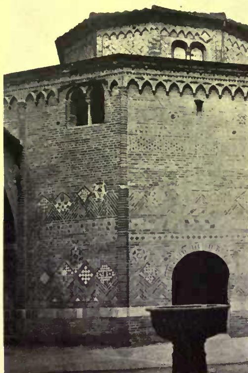
San Stefano shows ornamentation obtained in bonding, as well as the use of colored marble pieces set flush with the surface
