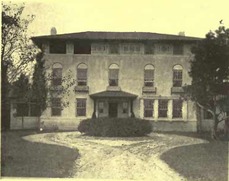
It seems rather strange that so few houses built of cement are in the Italian style, which, by reason of its flat wall surfaces, is well adapted to that material. Louis Boynton, architect
