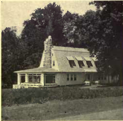
A distinctive house in the Scarsdale estates, which shows another type of the popular gambrel roof
