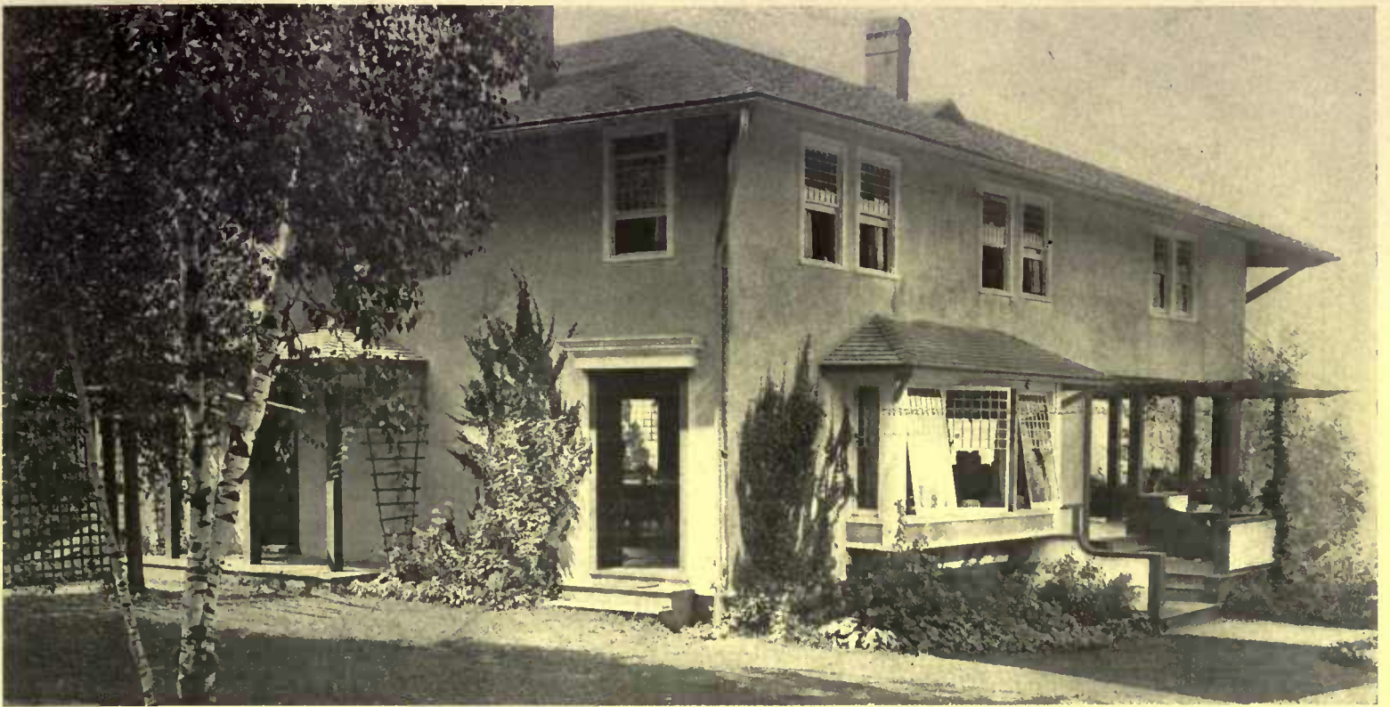
"The Fold" is practically a one-room dwelling on the ground noor, for besides the kitchen there is only the great Main Room. This opens on a veranda, however, which is used all summer as a dining-room, and is really an integral part of the house
