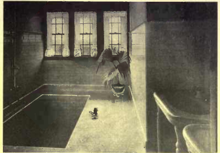
The sunken bath is a luxury beyond the majority of us. A low ceiling is necessary in the room below to allow for the sinkage, and this is frequently difficult to arrange
