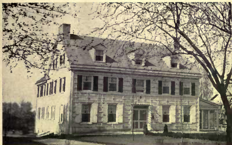
Where stone is cheap and not beautiful in itself, a stucco covering for it will result in an effective and durable house. Duhring, Okie & Ziegler, architects
