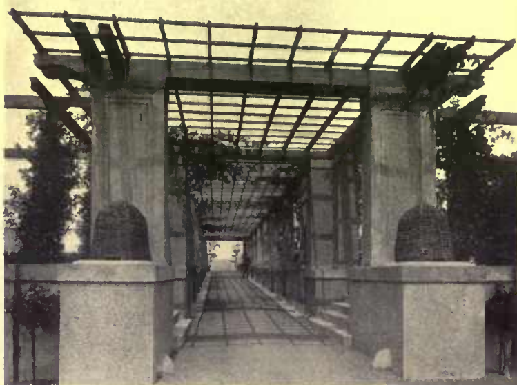
By means of paneling and a variety of textures on the different surfaces, concrete garden structures may be made far more interesting
