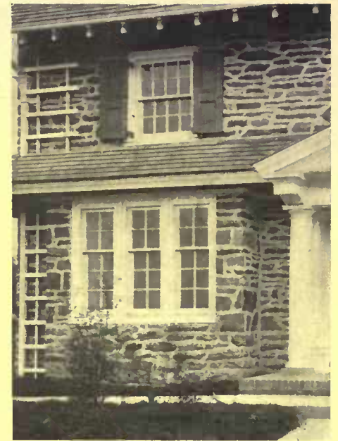
Wide flat pointing, where the front of the mortar joint is flattened out over the edges
