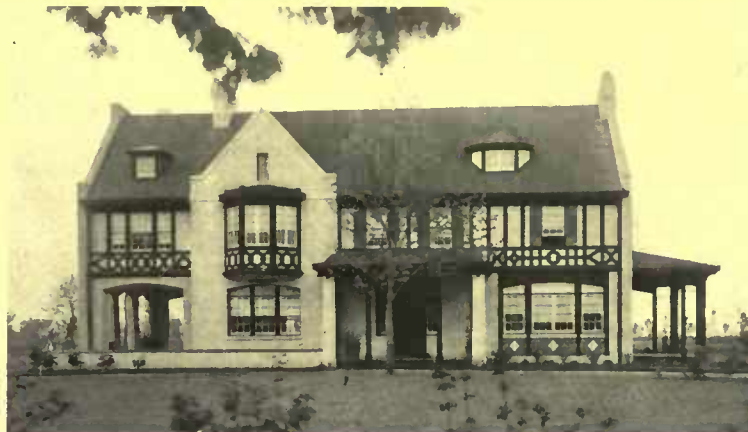
A Long Island house where half-timber work and brick paneling lend color to the stucco walls. Aymar Embury, II., architect
