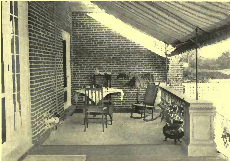
A terrace that may be shaded or left open to the stars by its roll awning on the framework of iron piping
