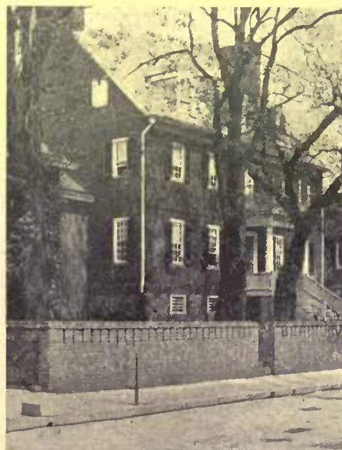
This old Southern mansion and its garden wall are of all-header bond, breaking joints
