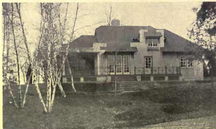
An interesting type of cement bungalow at Huntington Terrace. J. S. Conkling, architect
