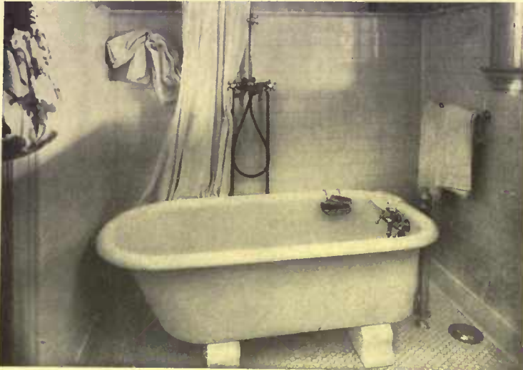
A shower arranged over the tub, with a linen duck curtain, is almost a necessity if one cannot afford a separate enclosure for it. A plan of this room is shown below, at the right
