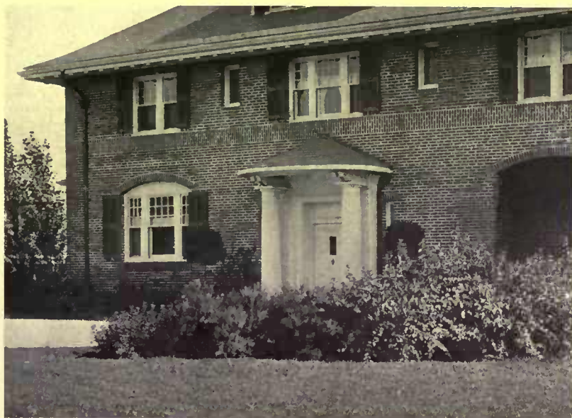
A flat belt course of bricks on end gives an interesting line just below the second-story windows, as well as for window sills and arched openings. Guy Lowell, architect
