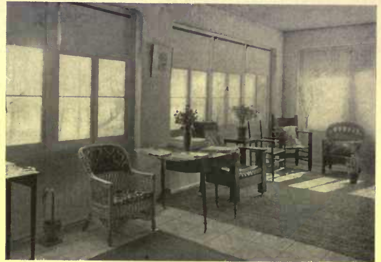
The larger of the two end porches is screened in during the summer months and provided with partitions of glazed sash above a wood base for cold weather. The plaster finish is very rough in texture. French windows open out upon the red tiled floor
