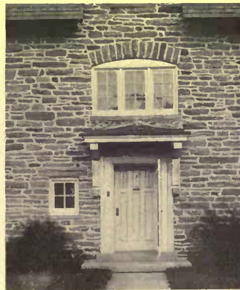
The need for color variety in masonry is well met in this Germantown stone marked with iron and mica
