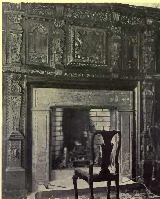
The dining-room fireplace at Baddesley Clinton—typical in its elaborate carving and the absence of a mantel shelf
