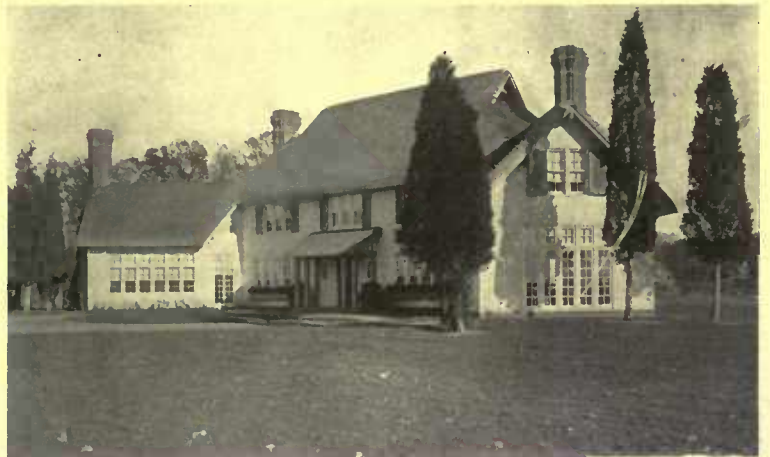
The summer home of Mr. George Davidson at Madison, N. J., Albro & Lindeberg, architects. An interesting variety in plan and also better lighting for the important rooms of the first floor have been obtained by swinging off at an angle the end wings
