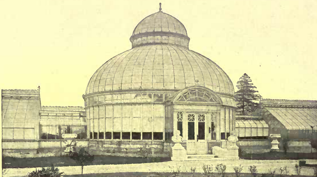
Erected for H. J. HEINZ, Pittsburg, Pa.
