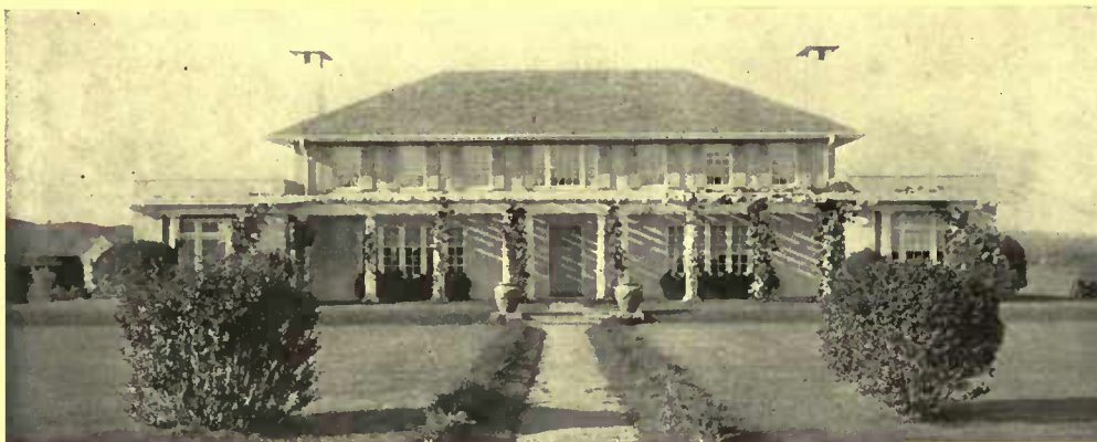
A sharp contrast is this summer home of Dr. Hollister at Easthampton, L. I., Albro & Lindeberg, architects, where the long horizontal lines of the building are accented in every way to harmonize with the lines of beach and horizon
