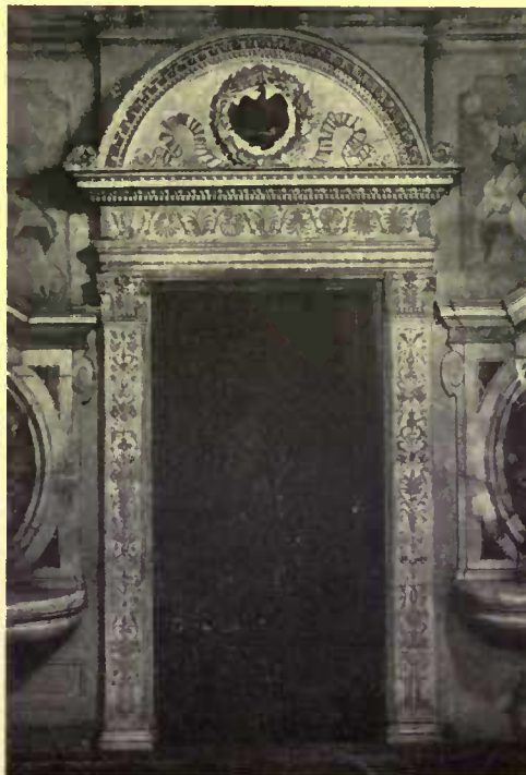
The use of pilaster and frieze was common in the treatment of doorways
