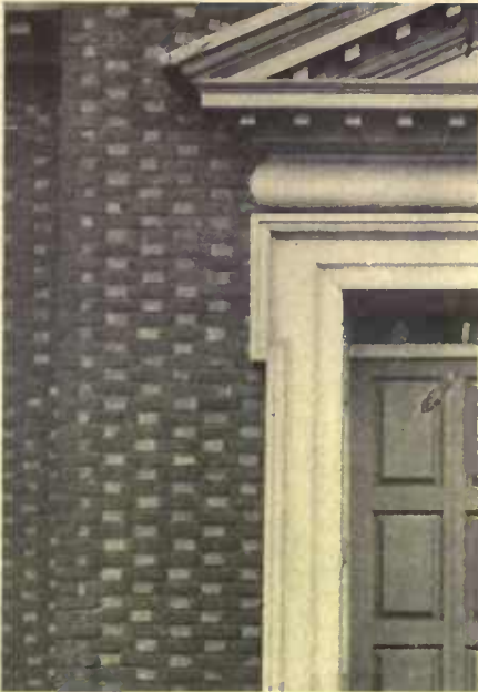
Flemish bond in the Old Swedes Church. The headers are burned to a bluish-black glaze
