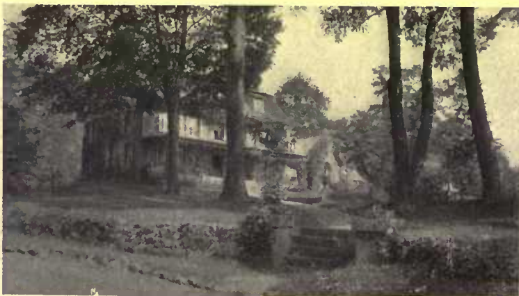
At Nyack, stone construction covered with vines seems most appropriate to the location.
