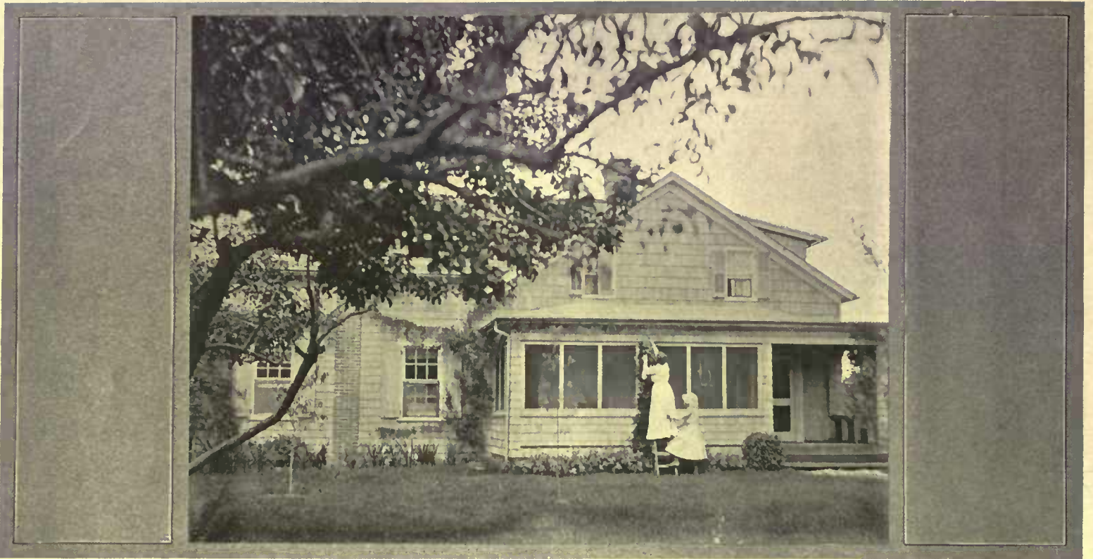
A screened porch was built across one end of the old structure, reached through a doorway from the living-room. A covering of shingles, dipped in a silvery gray stain, was put on over the original clapboards
