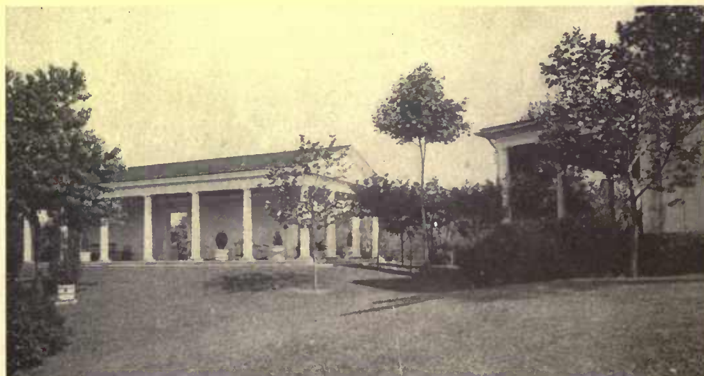
A novel form of porch that retains all the desirable qualities of the veranda without darkening rooms or spoiling the symmetry of the house. Mellor & Meigs, architects.
