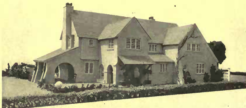
Rough-cast stucco walls are well represented by sandpaper. The roof is of overlapping layers of thin cardboard
