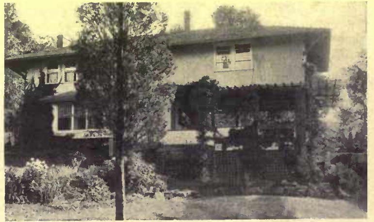
A feature well worthy of emulation is the awning-like projection of lattice-work over the porch railing, covered with vines
