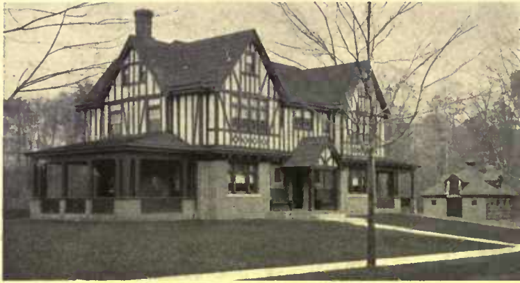
An interesting type of half-timber house in Cranford. Hollingsworth & Bragdon, architects.
