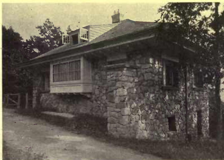
A random rubble of field stones and cobble-stones, with the joints raked out—modern work as is indicated by the latter feature; Colonial builders did not rake joints
