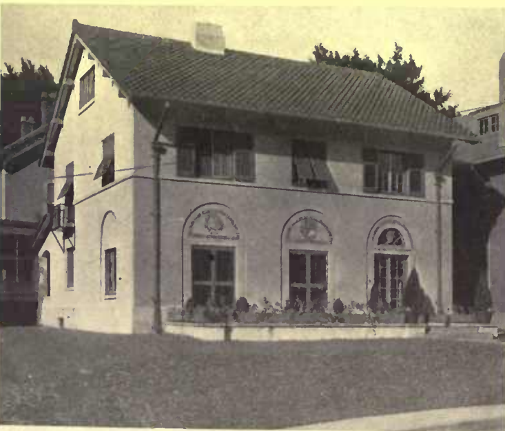
A particularly successful surface treatment of colored tiles and marble panels set in stucco. Mann & MacNeille, architects
