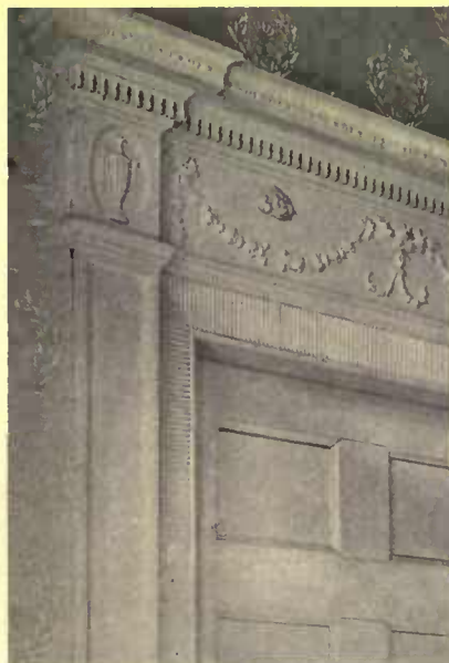
An old New England doorway showing curious dentils. The garlands are of papier-maché
