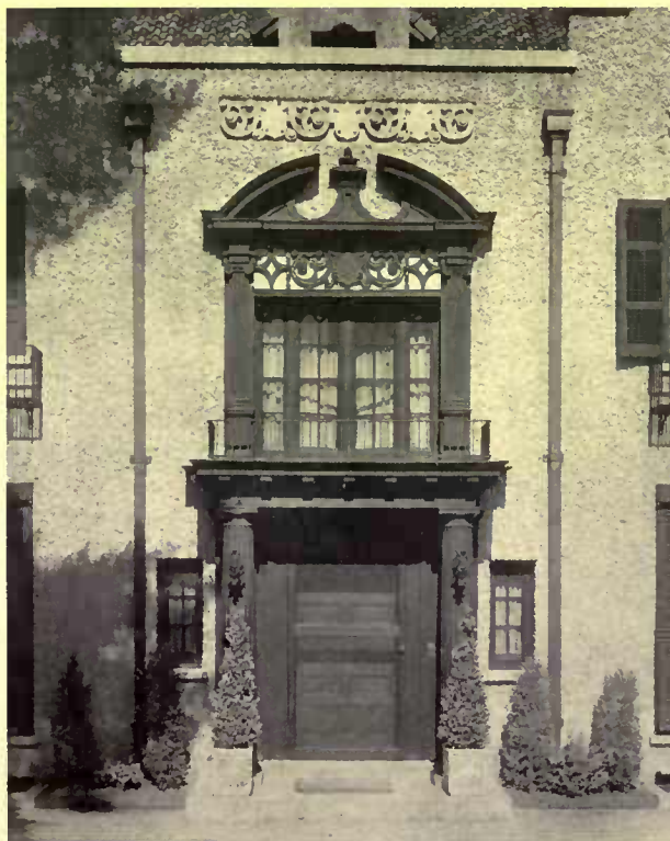
An example of moulded and colored cement panels set in a wall of pebble-dash that has been given a wash of thin cement. Oswald C. Hering, architect
