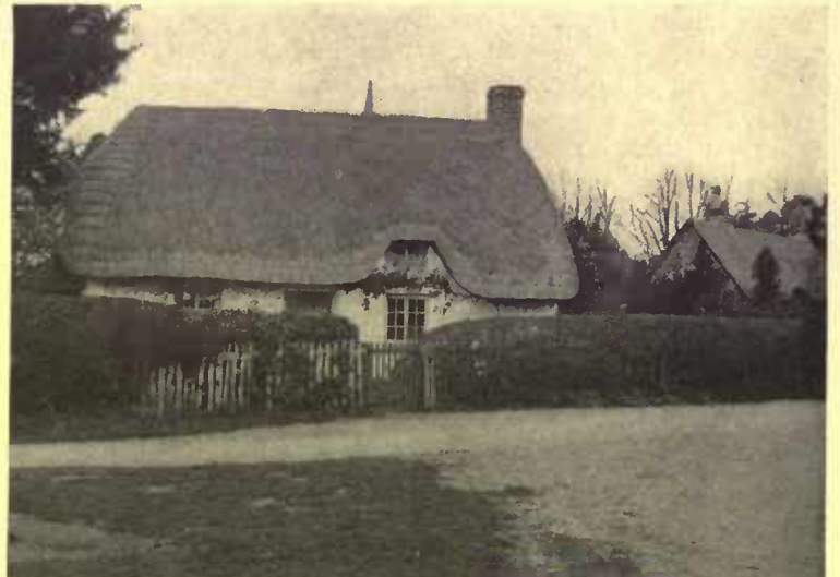
An important factor in the picturesque quality of English cottages is the fact that the builders were willing to sacrifice light and air upstairs for the sake of unbroken roof masses
