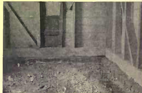
An earth floor lower than the outside surface is cold and damp
