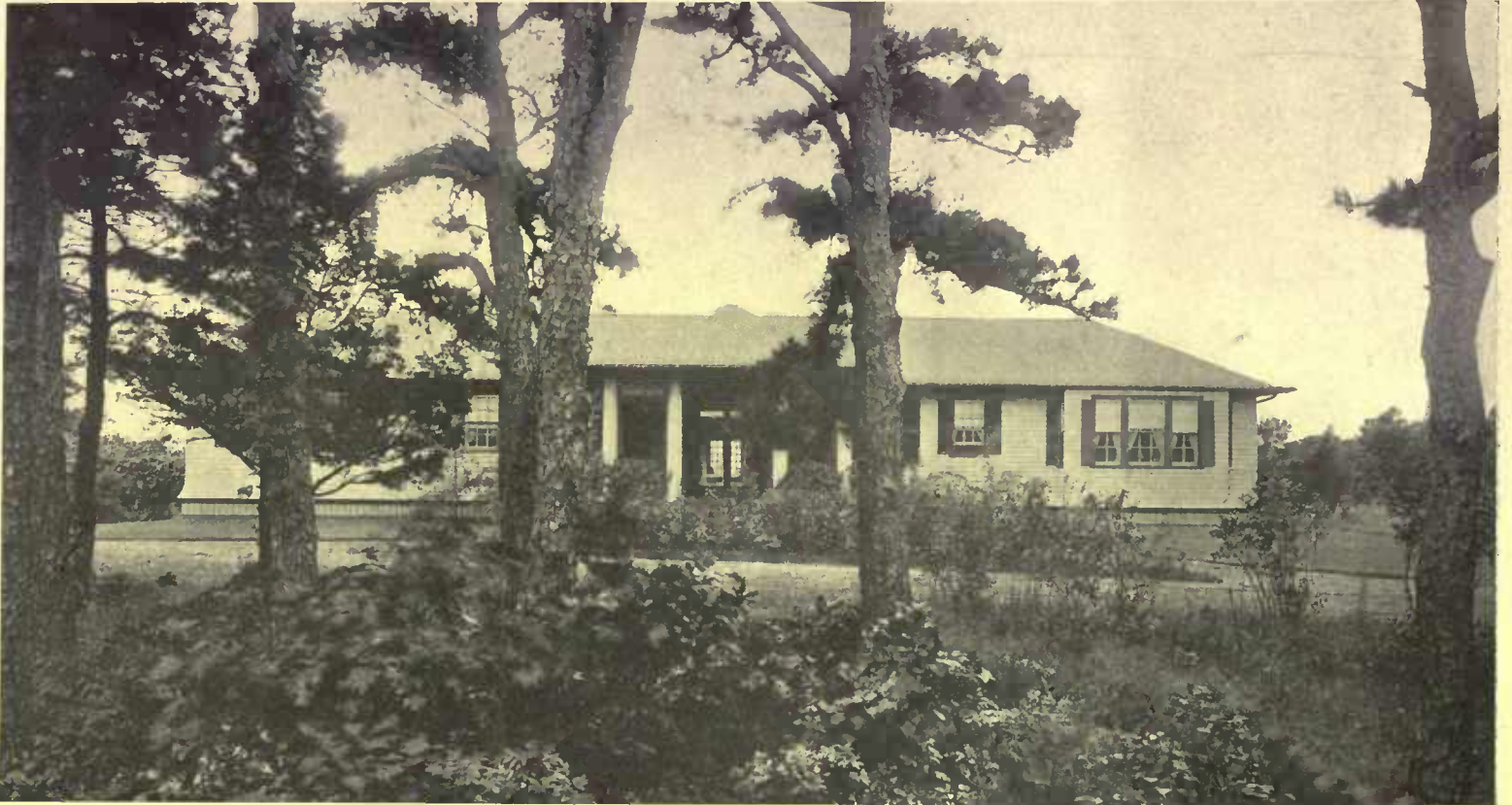
The large house that is built with but a single story is extremely rare. And the reason is not far to seek—cost. There is a great deal of satisfaction, however, in being able to do away with stairways, upper halls, etc., in favor of rooms that open directly upon the cool patio
