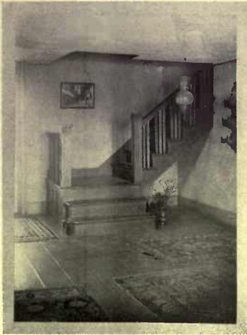
A new flight of stairs was put in at one end of the living-room—the latter combining the old parlor, sitting-room and hall
