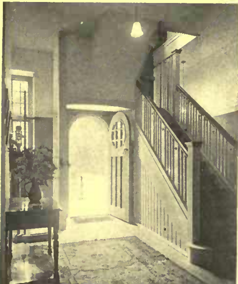
An interesting treatment of an entrance door and stairway woodwork. B. Parker and R. Unwin, architects
