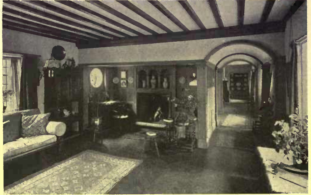
The hall, with its fire corner screened from the passage to the entrance hall. Teak blocks are used for the flooring, and oak paneling in the inglenook
