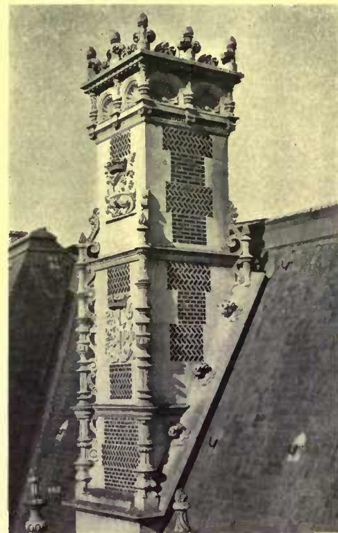
A chimney from the Château of Blois, France—alternating panels of herringbone and running bond, with stone quoins
