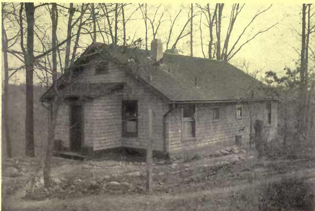
The extension porch serves for several rooms. It keeps tradesmen from the kitchen and the refrigerator closet makes a good storage cellar
