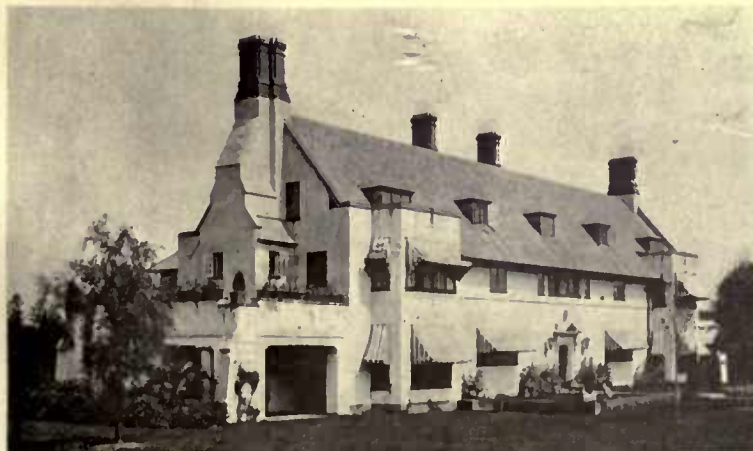
A felicitous arrangement of dormer windows so that the line and proportion of the roof are not disturbed. Light frames and casements are unobtrusive and do not destroy the balance
