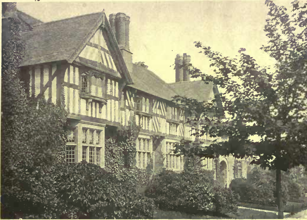
Modern half-timbered houses in a group at Port Sunlight, one of the model English villages. The pins holding the timber ends together form a very decorative detail
