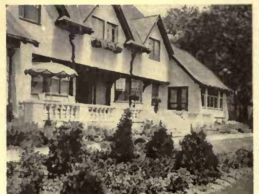
Along one side of the Corey house extends a broad terrace with the principal view
