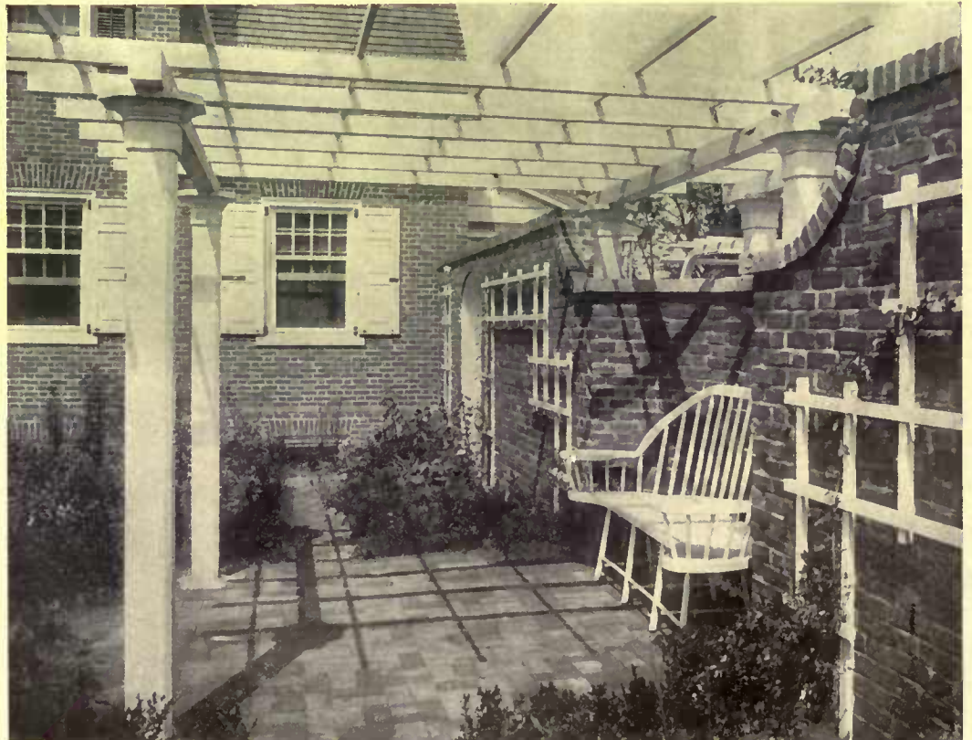
Where the garden wall is of brick, it is best of rough surface. Put the lattice work a few inches from the surface to prevent the accumulation of dirt and insects
