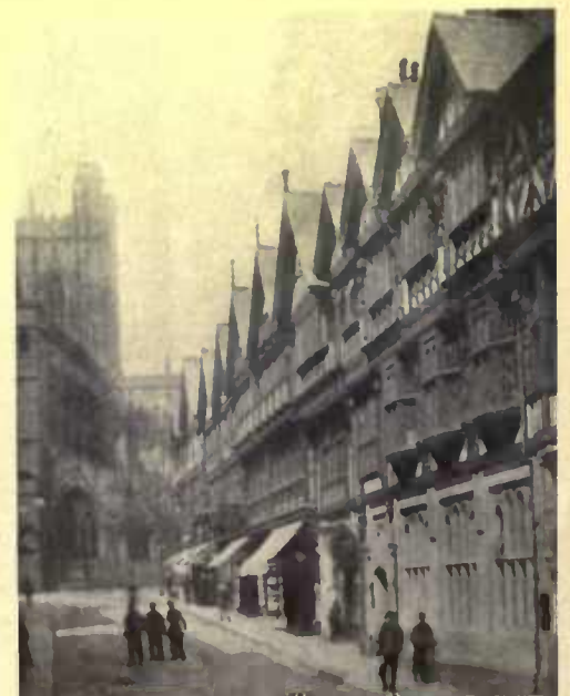
St. Werburgh's Street, Chester, showing the typical overhang and the use of carving on the main horizontal timbers
