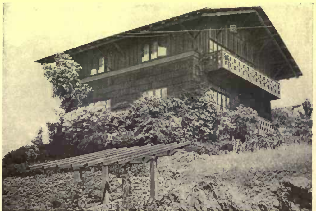
The home of R. C. Hutsinpillar. A pure type of the lowland chalet, giving a good example of the use of projecting roof supports—a common feature abroad. Maybeck & White, architects
