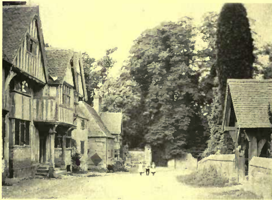
A street of old half-timbered houses in Chiddingington, Kent, marked by the overhang of upper stories—a characteristic feature
