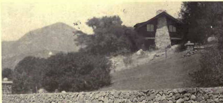
Felsengarten, the California chalet, is built according to all the conventions of the Alpine chalet. Myron Hunt & Elmer Gray, architects.
