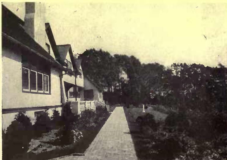
Looking across the south front from the billiard-room corner. The wide brick-paved path is equivalent to a second terrace
