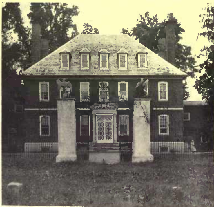
The hip roof on this old Virginia house avoids the effect of extreme width by the use of five narrow dormers. It is suggestive of strength and virility consistent with the hospitality of the time
