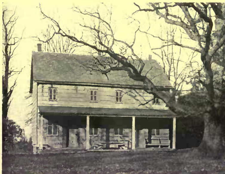
In contrast to the similarly built house above the stained and weathered walls with bleached blinds here give the impression of desolation and poverty. Painting has been put off too long
