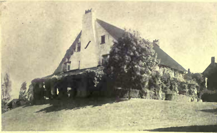
There is a convincing charm in the perfectly simple roof. The ridge falls away on either side of the ridgepole and the slope is entirely unbroken by dormers. Chas. Barton Keen, architect
