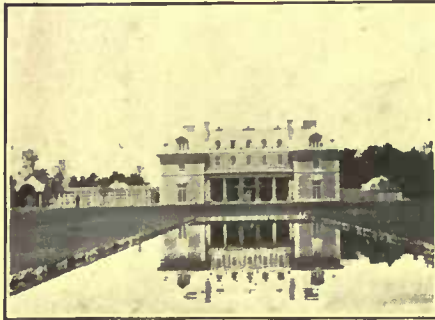
Kelsey Heated. Berkshire Hills, Mass. Delano & Aldrich, Architects, New York
