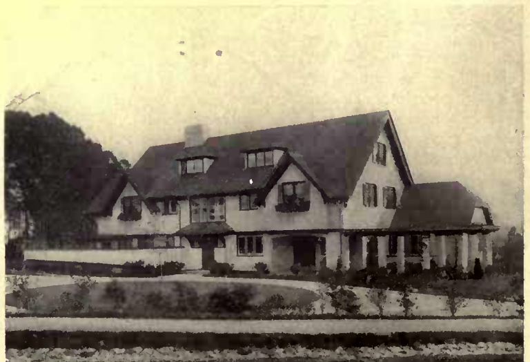
On the north side at the rear corner is a small covered piazza with a pergola adjoining. A plastered wall encloses the kitchen yard
