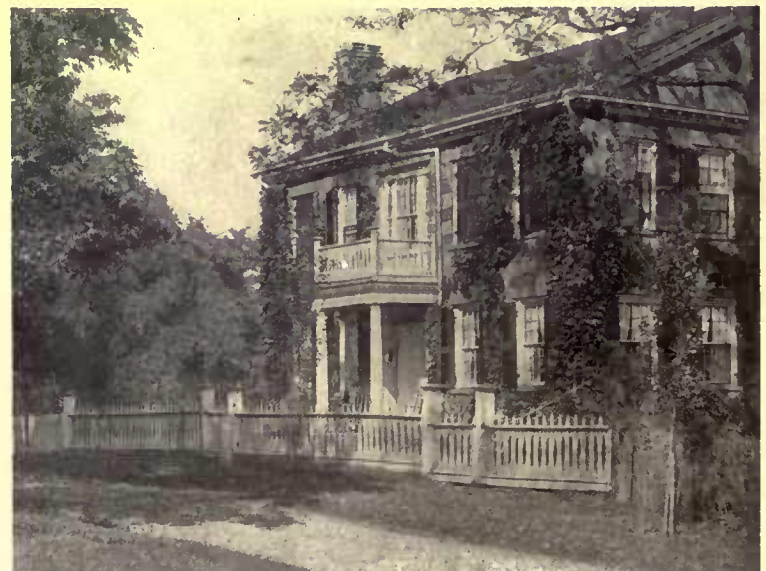
The sheaf pattern of these fence pickets is duplicated in the balcony rail, thus increasing the unified effect of house and grounds
