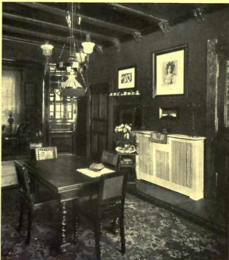
The German architect makes his heating apparatus a decorative feature by using unfinished radiators and covering them with a removable screen
