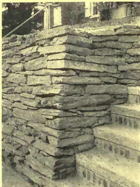
The dry wall is a great deal more effective if irregularly laid
