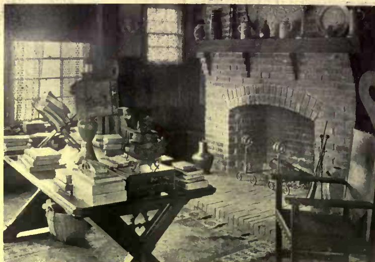
The raised hearth with flanking seats is characteristic of the inglenook and results in making the fireplace a distinctive feature
