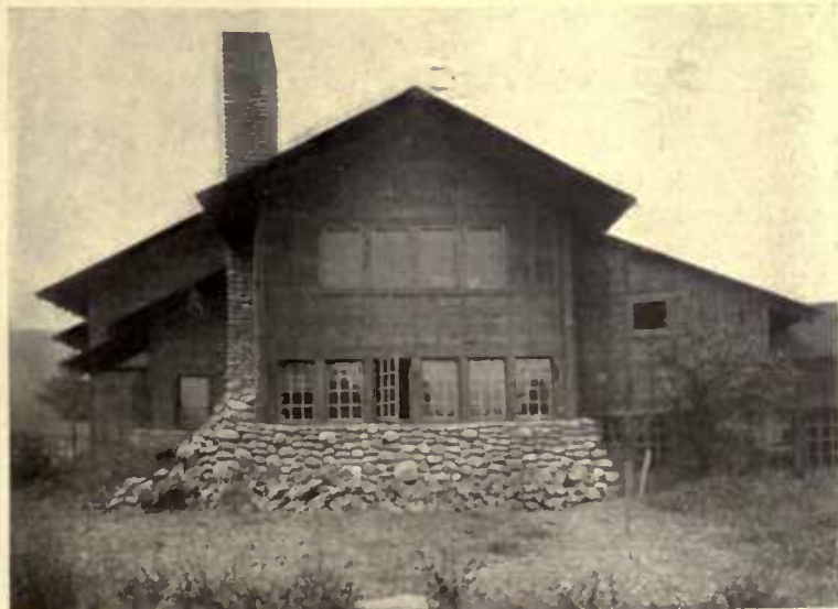
The office, chicken houses and trout hatchery are built as they would build in our climate and with our materials
