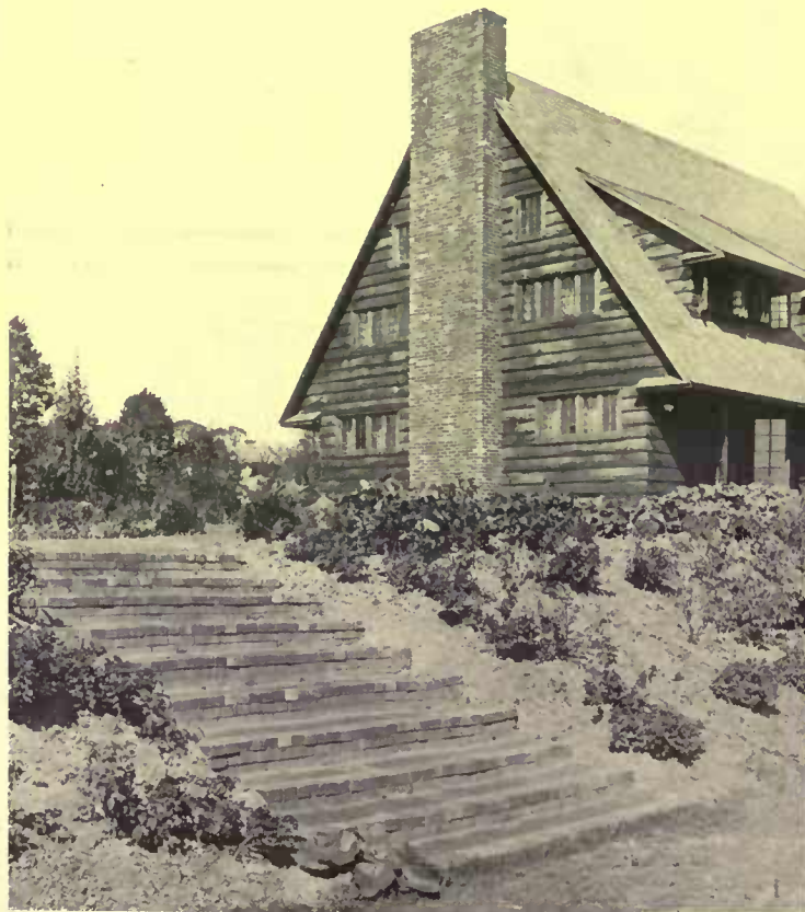
Another view of the terrace front of the cottage, with the brick steps, which lead from the pergola to a lawn and tennis court several feet below. These steps are another example of the artistic value of bricks irregularly laid and of different color
