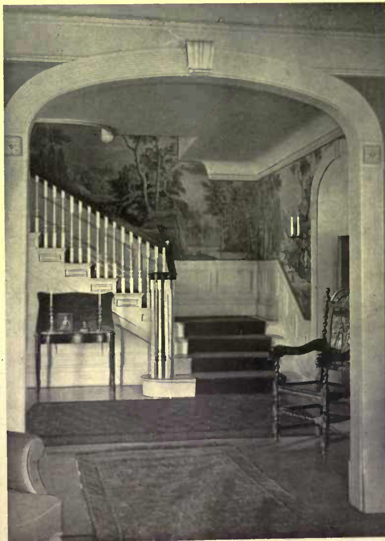
An old house that was redeemed largely by the new staircase and the changing of dark, gloomy woodwork to the white by refinishing. It seems hard to paint walnut, but that is sometimes the only way out of the difficulty
