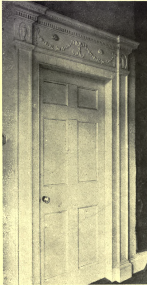
The reeding and detail around this door are typical of the best Colonial work. The garlands were seldom carved, but were of papier maché and very lasting
