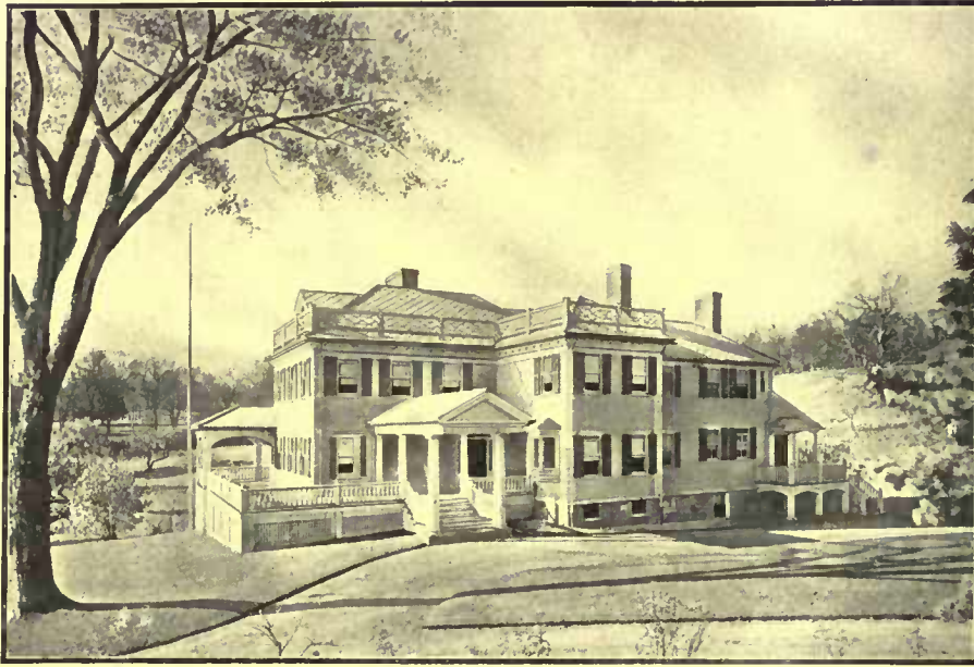
Asbestos "Century" Shingle Roof—Residence Frank C. Childs, Lexington, Mass.
