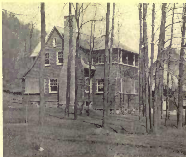
When the sleeping-porch occupies a free-standing wing as here, sliding sashes should be provided at either end, but ordinarily the whole side may be left without them
