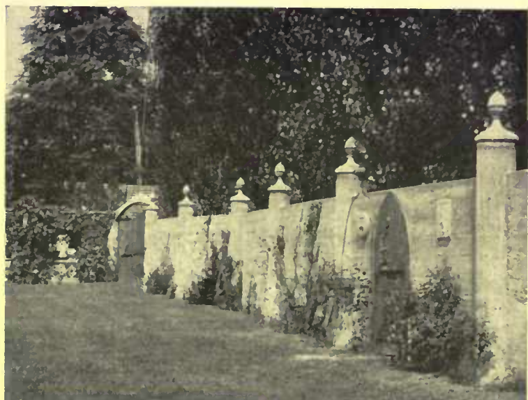
The concrete wall should be of rough surface and is made attractive by vines and shrubs
