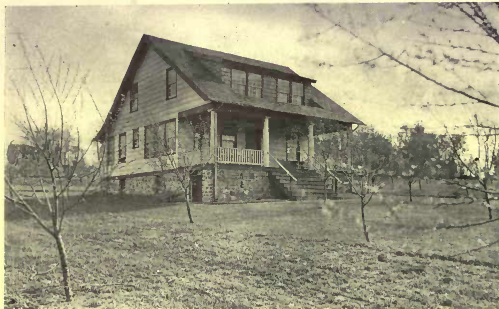
Wide boards are laid up horizontally like clapboards on the wood frame over the underpinning of local stone. There is a splendid place for garden tools under the porch
