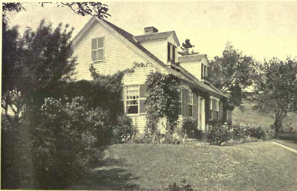
Farmhouse at Cornish, New Hampshire, showing the alteration of an old house without the destruction of its original character of roof lines
