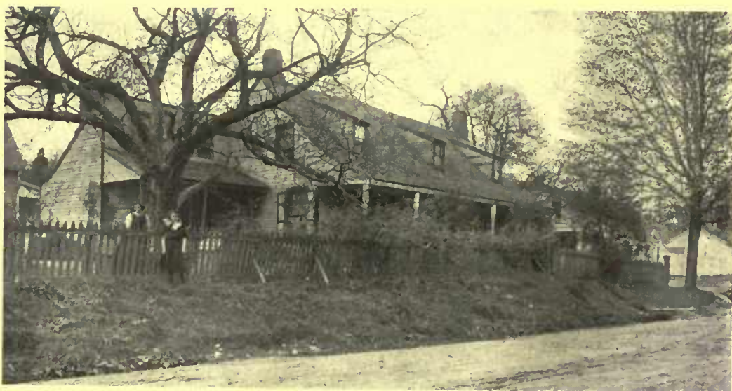
A house at Mianus, Connecticut; an early example of the forerunner and inspiration of much that is evidenced and delineated in the Woodmere type below
