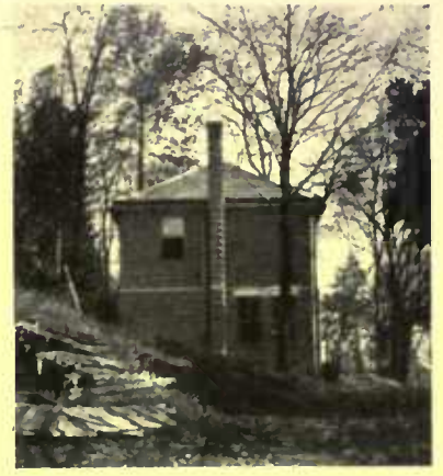
Over the cement blocks wood lath and stucco were applied
