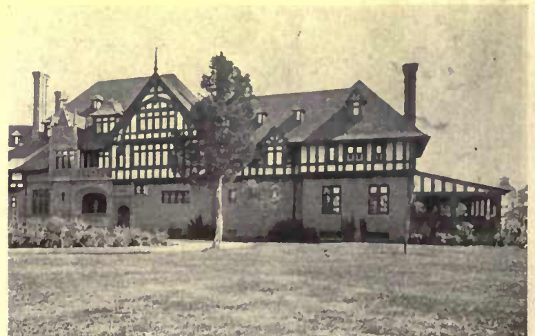
A Cedarhurst, L. I., example, Barney & Chapman, architects, where the horizontality of the building has been accented over the brick base
