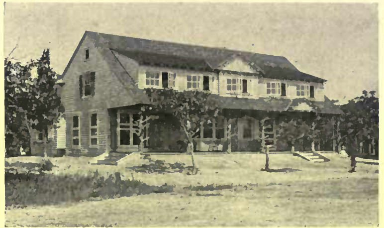
The solid line of windows breaking through the roof on the second floor is successful in that they appear to be part of the roof and the effect of a one-and-a-half story house is preserved
