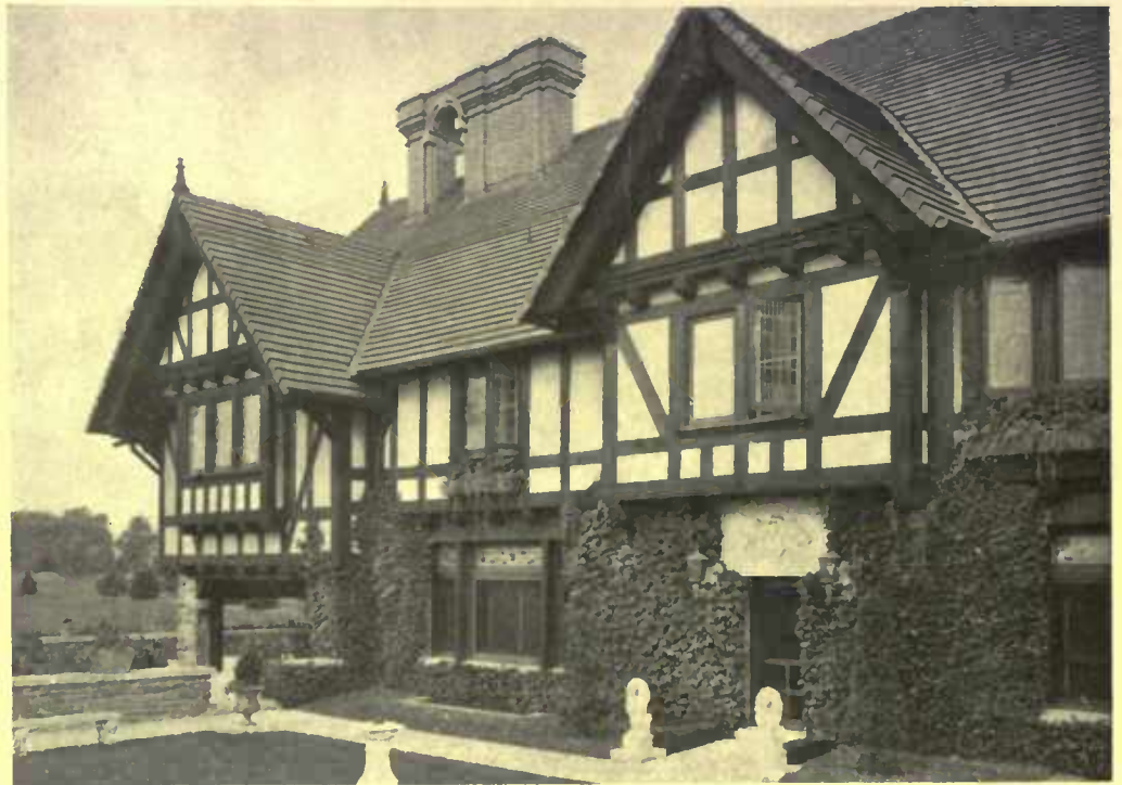
A modern country home near Philadelphia, Oswald C. Hering, architect, where the timbers are really structural, not mere strips nailed on afterwards
