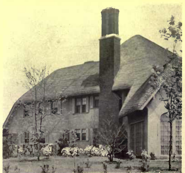
The softness and flexibility of the thatch roof is sometimes simulated to advantage by laying shingles with varying but narrow spaces exposed to the weather. Albro & Lindeberg, architects
