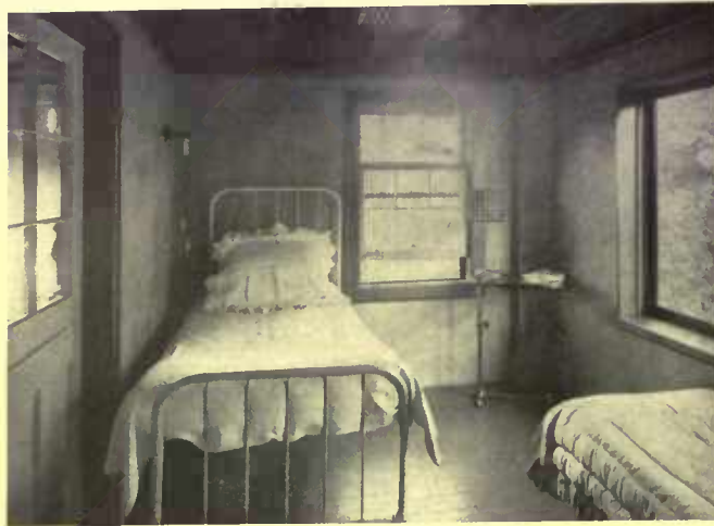
Where the exterior walls are of stucco, the inside of the sleeping-porch is usually finished in the same material, though it is cheaper to sheathe it with wood
