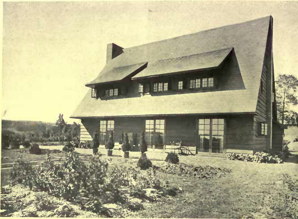
The rear of the cottage is really the garden front. At the left is a formal arrangement of rose beds, with a sun-dial in the center; beyond, at the right, is the orchard
