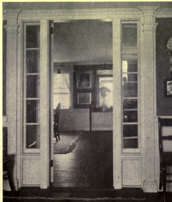
Such treatment as this successfully shuts off a room from the hall without the disagreeable or darkening effect of solid doors
