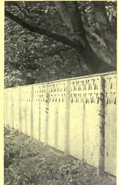
A well designed series of openings along the top of a high board fence will redeem it.
