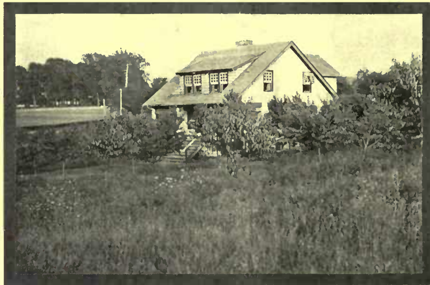
One end of the lot, 50 x 200 feet, adjoins the street, to which the house turns its back, giving the porch the splendid view over miles of country
