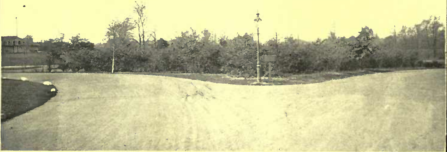
ENTRANCE TO BRANCH BROOK PARK, NEWARK, N. J., ROADS CONSTRUCTED WITH TARVIA X
