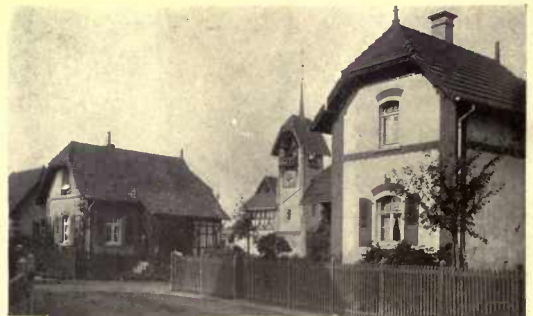
The jerkin-head roof is not apt to be successful unless managed by very skillful hands, and is to be used when the conditions approximate those of its original environment
