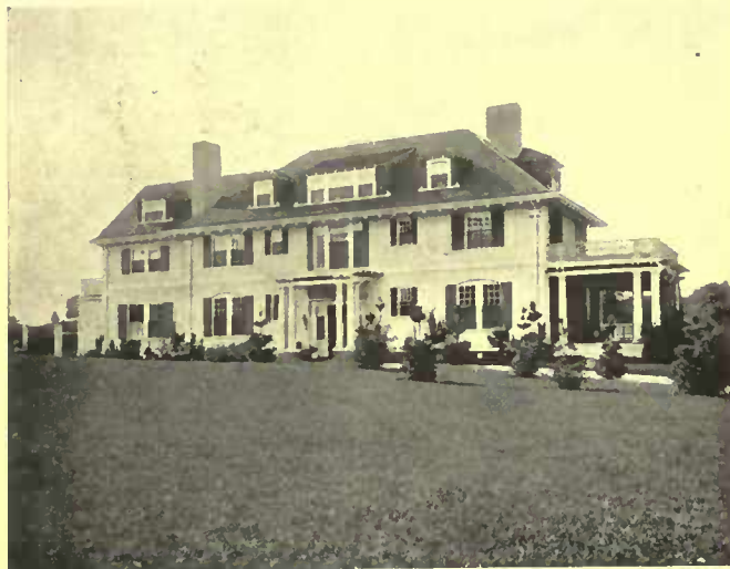
Residence of Chas. F. Leland, Southborg, Mass. Heated and Ventilated by the Kelsey System. James Pardon, Architect, Boston, Mass.
