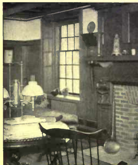
The window-seat is only one of the means whereby a radiator may be placed almost entirely out of sight
