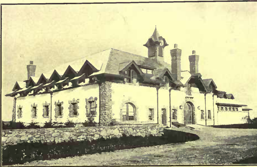
Asbestos "Century" Shingle Roof—Stable, Theodore M. Davis, Newport, R. I.; Architect, Theodore Davis Boal, Washington, D. C.; Contractors, Simpson Bros., Corp., Boston, Mass.
