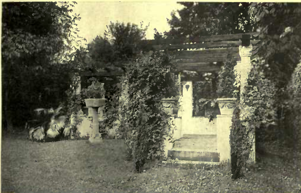
Where porch space is at a premium the detached arbor with a paved floor and low wall is a successful substitute
