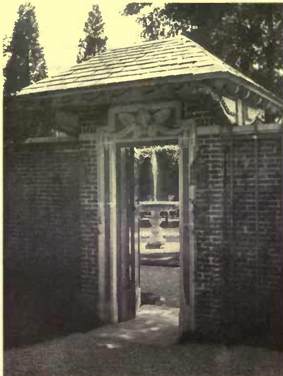
In the entrance gates Mr. Hastings has given a freer rein to his fancy for color, using terra cotta with the brickwork
