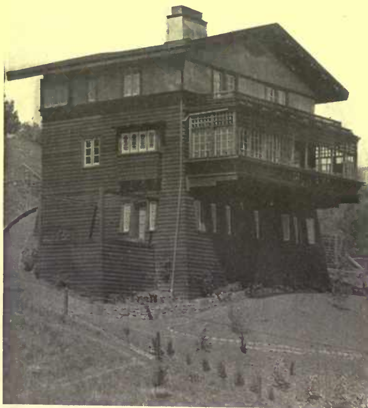
This picturesque house shows how American ideas in plaster and timber may be applied to the chalet type. The enclosed balcony is an elaboration of the little balcony in the Swiss chalet above. L. C. Mullgardt, architect
