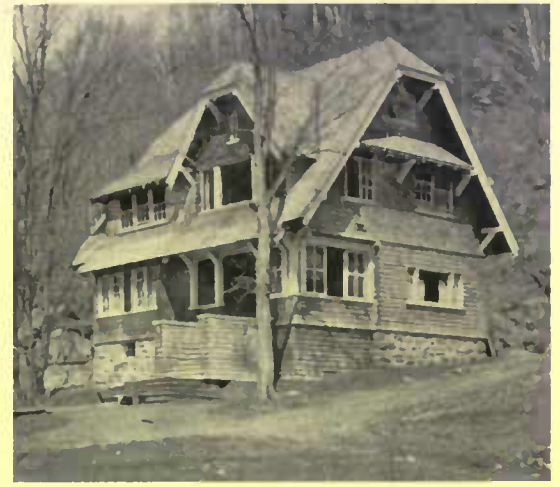
It is no easy matter to design a sleeping-porch as an integral part of the mass, yet that is one of the most important considerations aside from the practical ones
