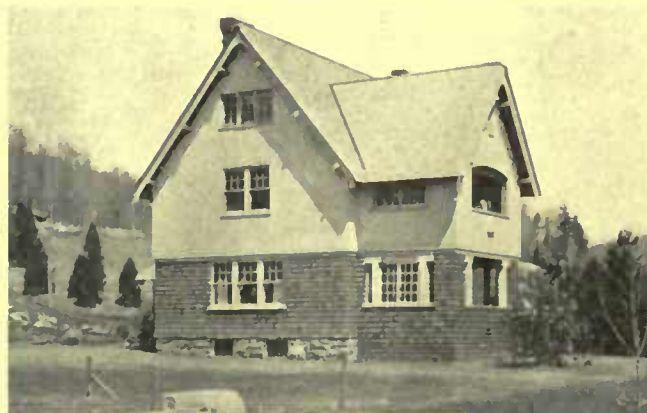
One can readily see that the two south porches, one above the other, contribute to the unity of the design by their treatment as a separate gable
