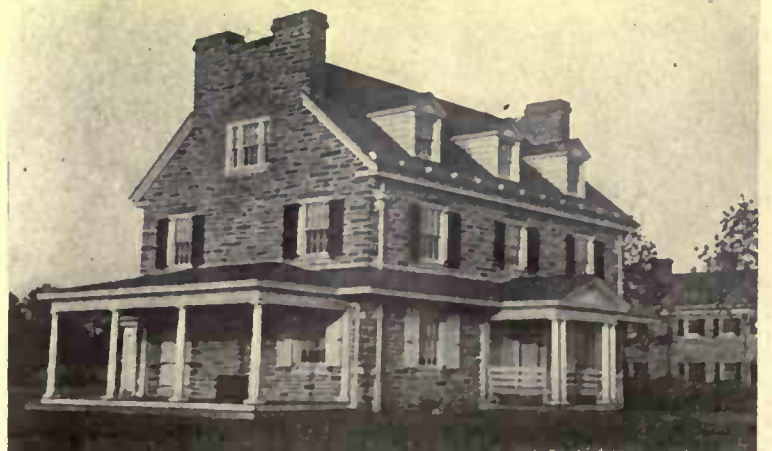
Great flanking double stone chimneys at each gable end of a Colonial house give an appearance of strength and solidity that diminishes the importance of the roof itself
