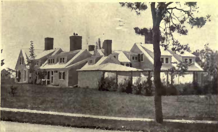
The spasmodic sky-line and confusing angles of this collection of buildings may serve as an example of what not to do when planning a new building if unity and repose are to be obtained
