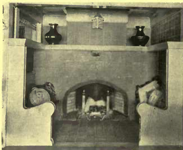
An interesting effect is obtained here in tiling the entire inglenook. The seats and mantel are all one
