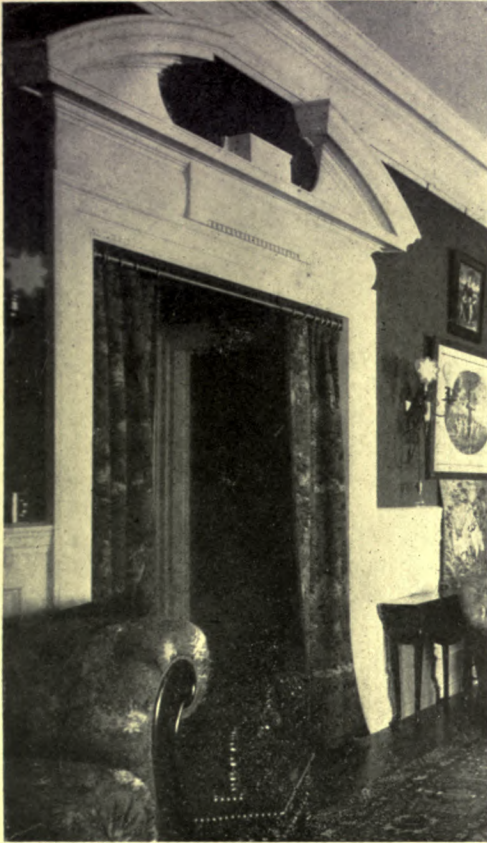
The form of the broken pediment over this doorway lends dignity to the apartment by the use of simple lines. There is little detail work here
