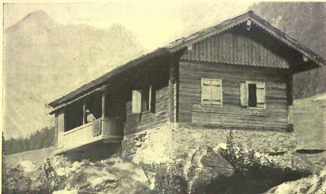
A Swiss mountain chalet, which has features evident in the two American adaptations below it. The dovetailing of the timbers at the corners is noteworthy
