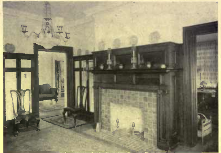
The woodwork of the dining-room is of birch and cherry to match the mahogany furniture. The fireplace here is also of hand-made tile
