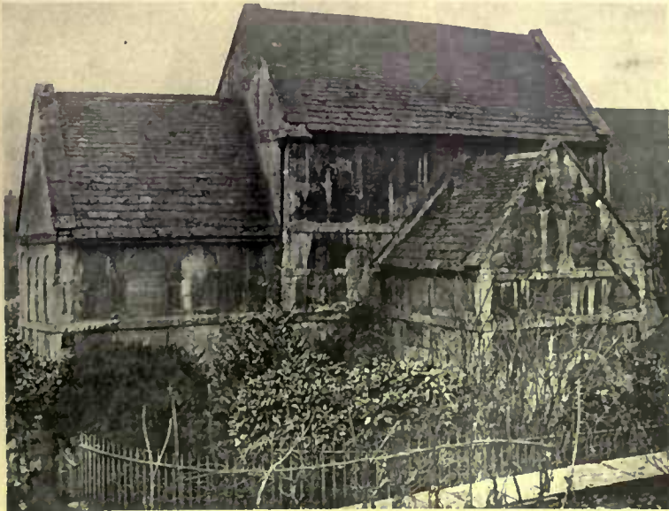
Slates of graduated size and thickness, varying in color, give unlimited possibilities for obtaining distinctive character in the appearance of the roof
