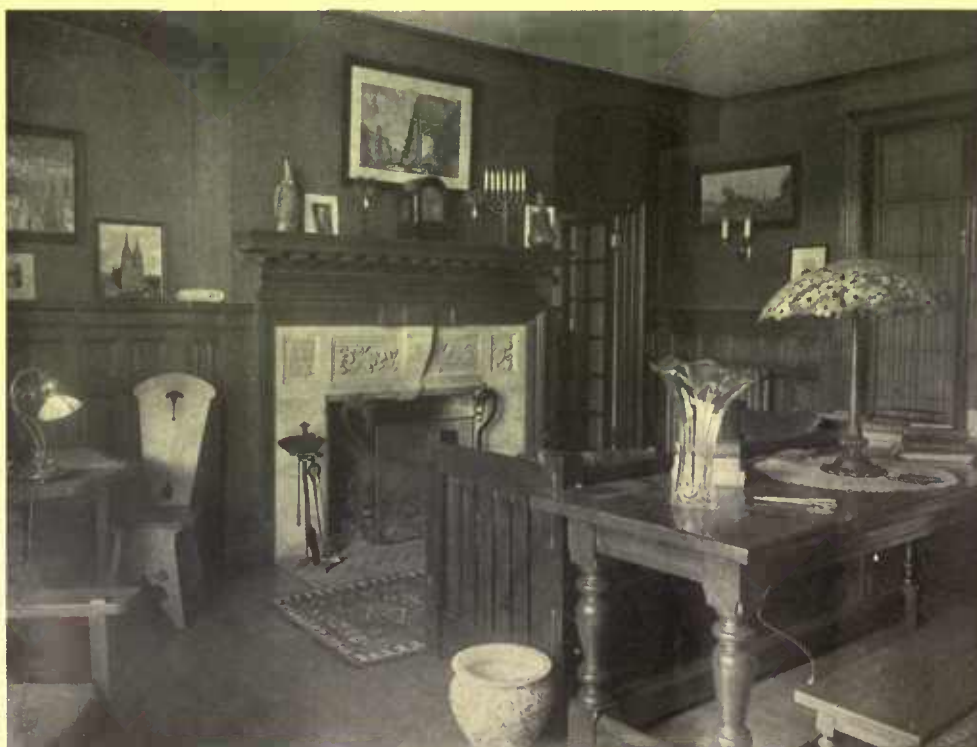
One knack in remodeling is the adaptation of materials to new uses. This caen stone fireplace was too narrow. The addition of the keystone rendered it available
