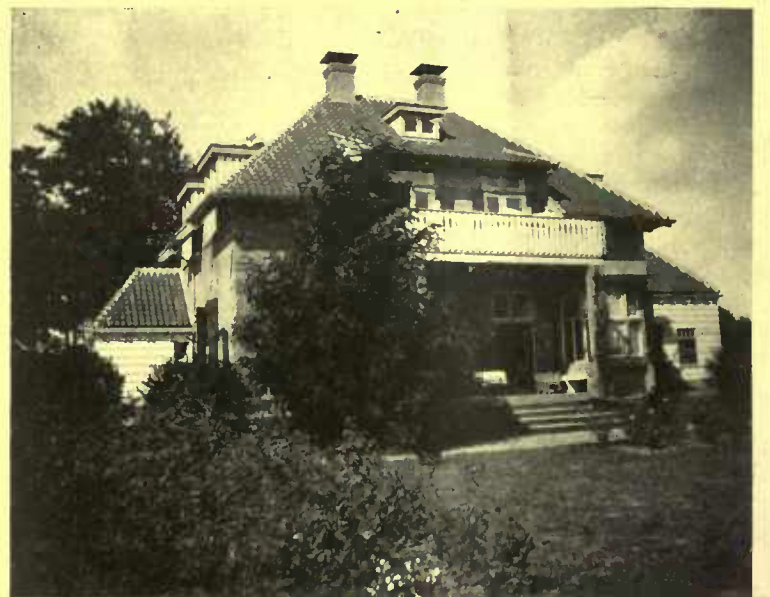
Instead of being a mere shed, this piazza roof is inclosed with a railing and fitted up as a useful porch
