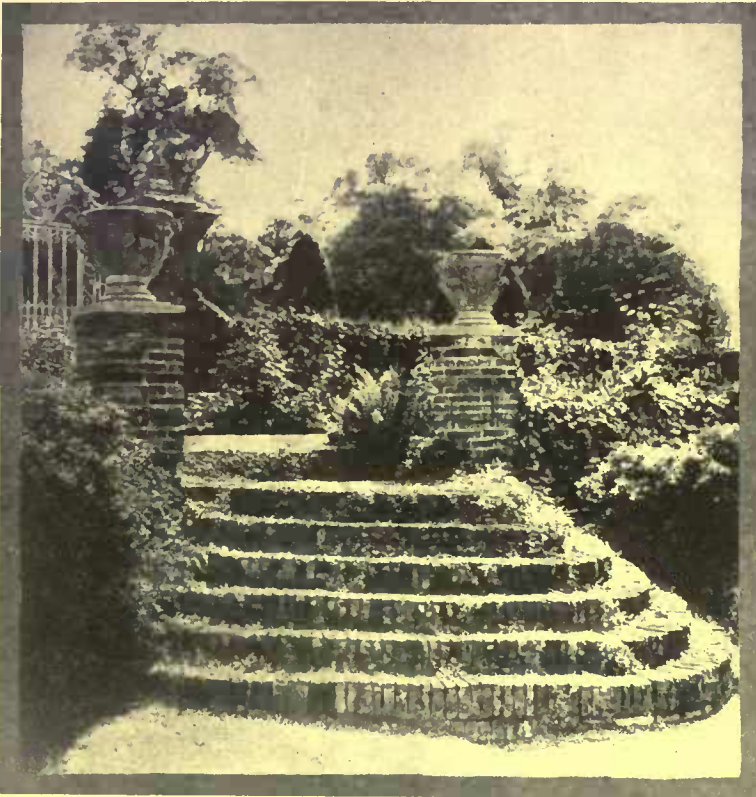
A very successful treatment is achieved by laying circular steps of bricks; rock plants may grow in the crevices
