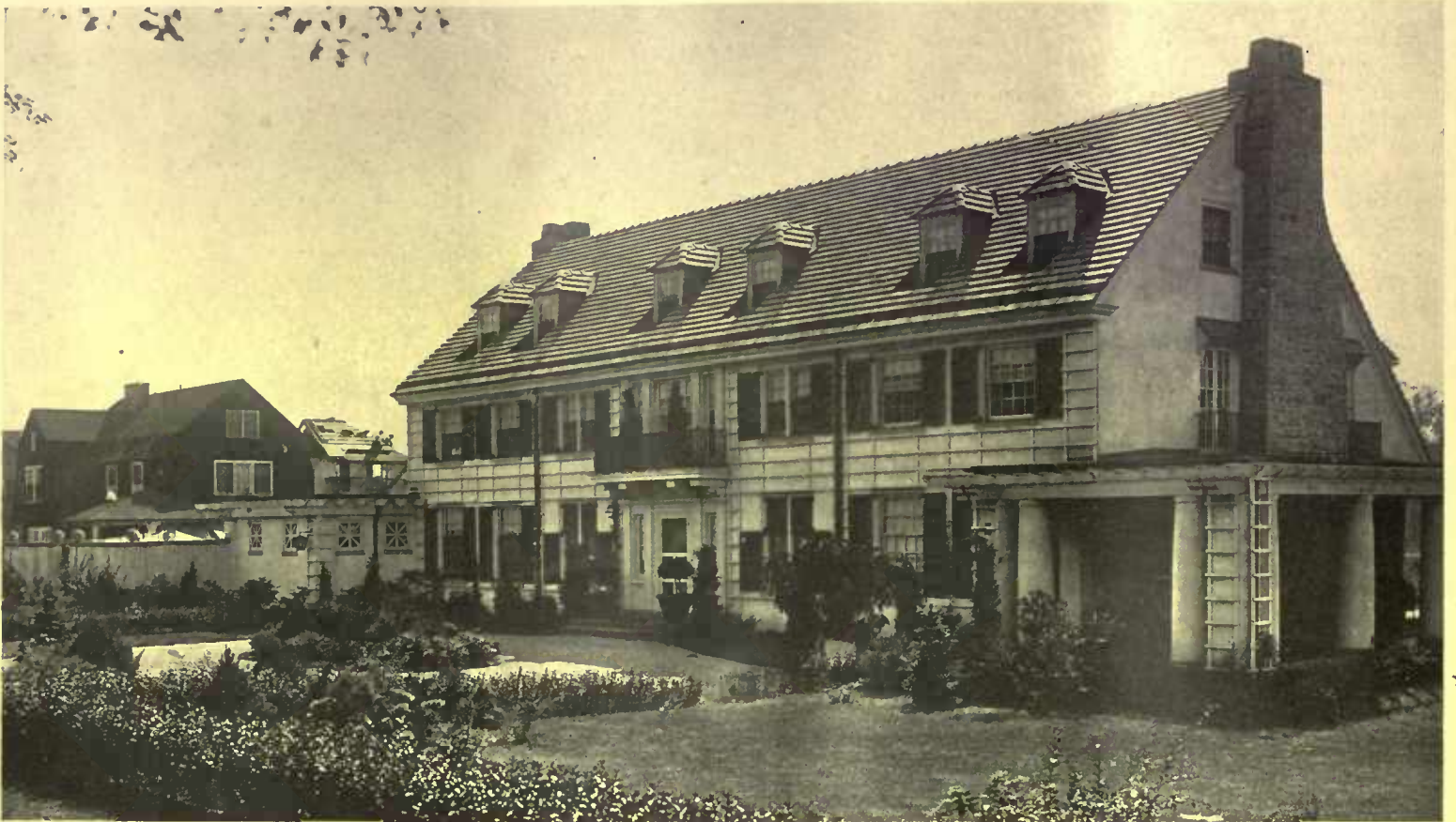
The north elevation of Mrs. Graham's house faces the street, but is not more elaborate than the garden side. Its treatment, however, is more formal. The service section and drying yard is on the left. It is made attractive and almost symmetrical with the porch. This entrance opens upon the main hall
