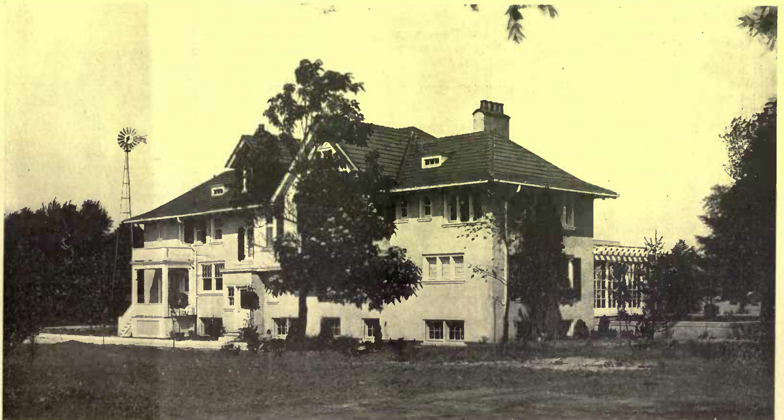
The rear of the Coffin house shows the advisability of their foundation plans in the height of the cellar windows. The sleeping porch can be seen at the right. The second rear entrance noticeable in the plan permits tradesmen to bring in supplies without tramping through the kitchen
