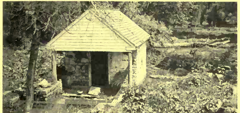
The spring itself is located at one side of the door and the water flows thence into the house
