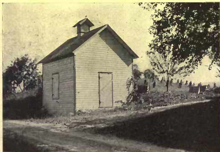
The best site for the ice house built above ground is one where the land slopes sufficiently to drain off the water from the melted ice
