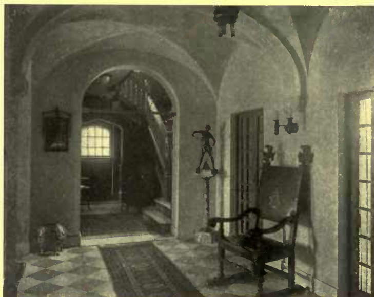
As solid supports were necessary for the additional development of the upper story pillars were used which suggested the vaulting in the hall
