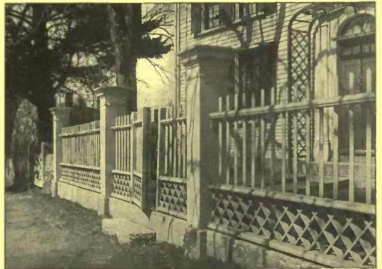
A combination of a stone foundation with the wooden fence is permissible and adds to the term of service. A front fence at Bedford
