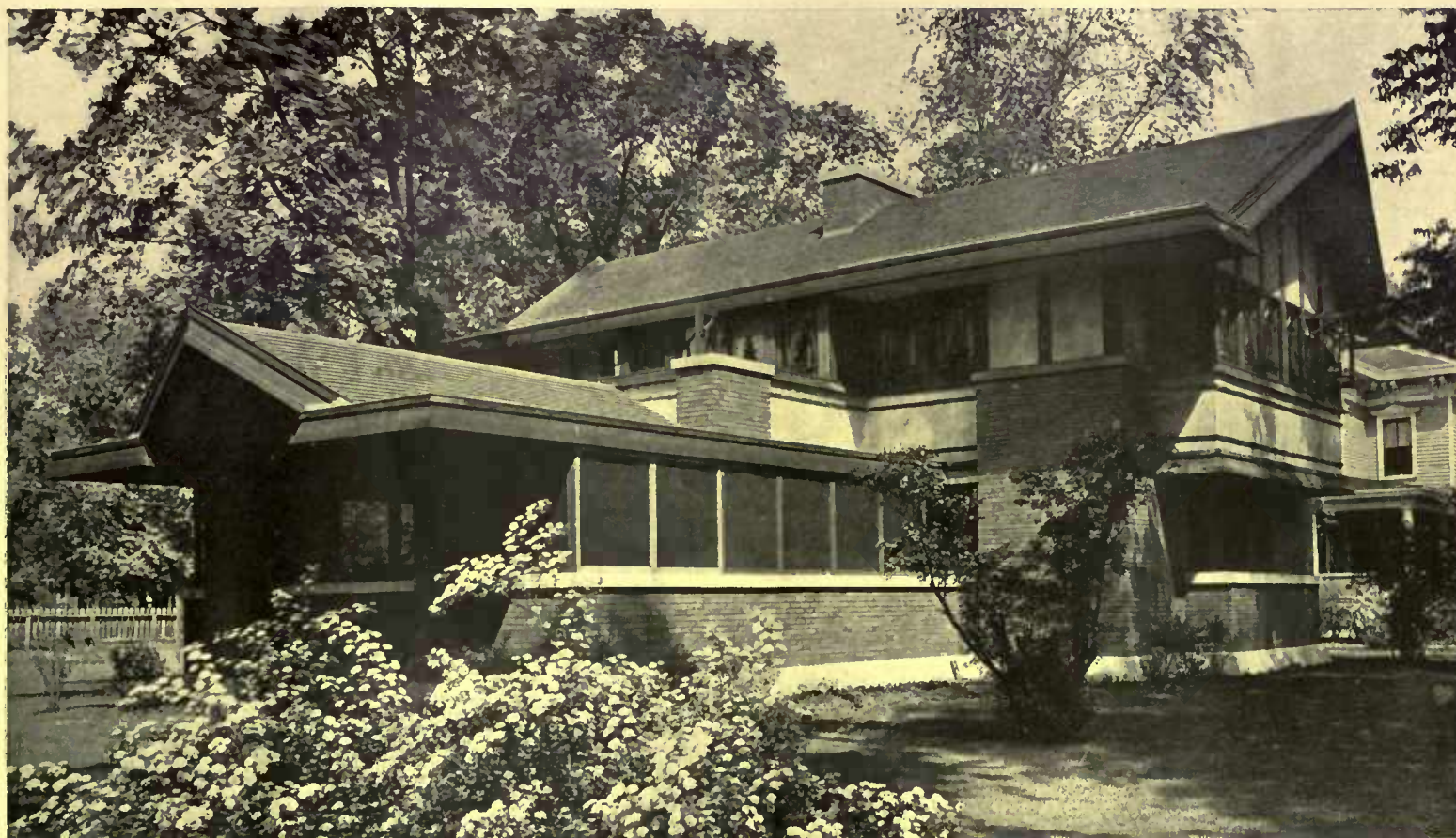
In the environs of Chicago has arisen a distinctive type of house design sometimes called the Chicago School. This style is well represented in much of the work of Mr. Walter Burley Griffin. It endeavors to produce a home that reflects the environment of the vicinity and to create a background that is entirely consistent with the life of the place
