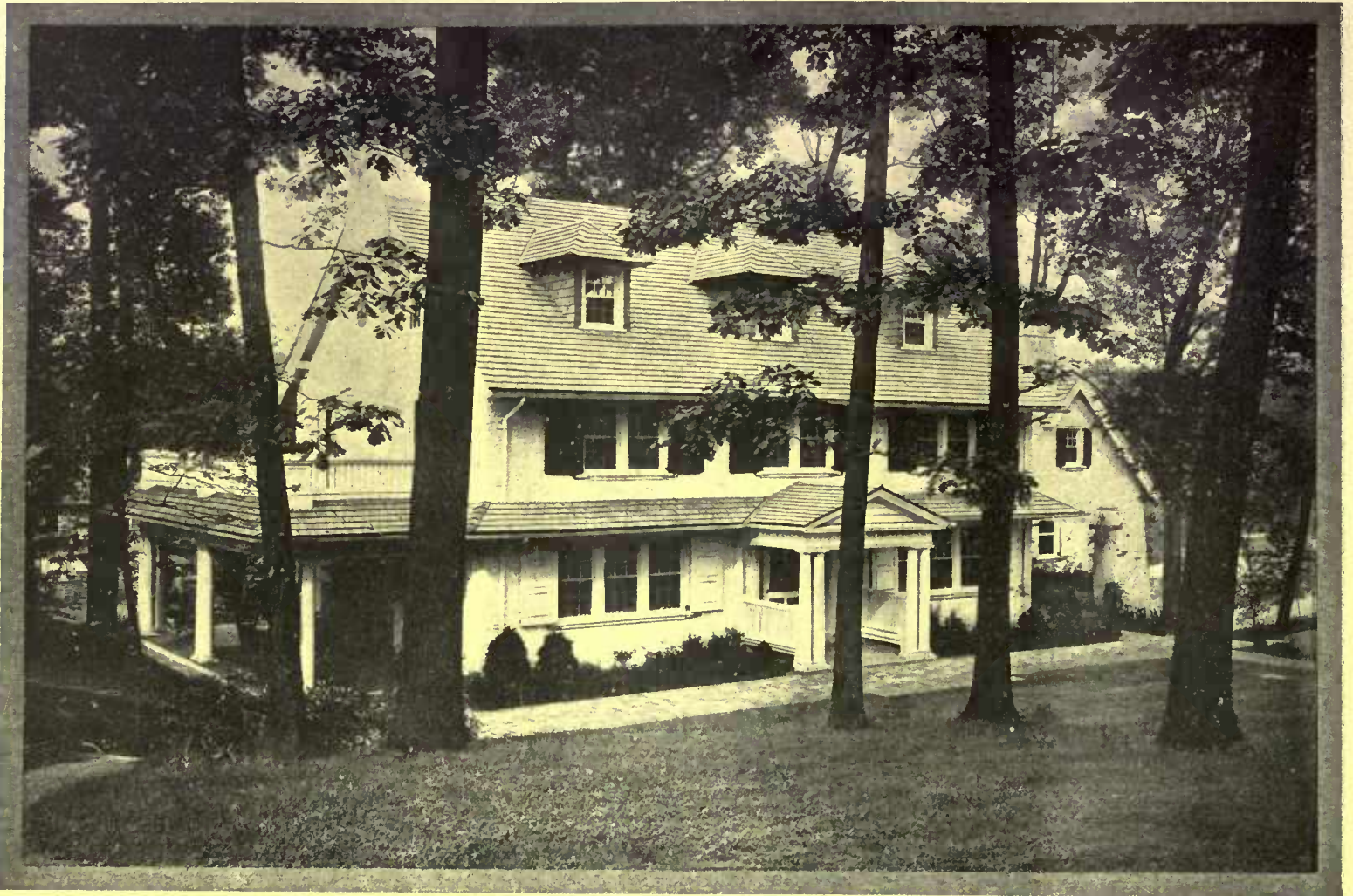
In Mr. Baker's house the architects have excellently coped with an irregular situation. The house fits naturally into the different levels, yet has a compact mass and a main outline undisturbed by cuts and breaks. The problem of saving the trees is beautifully answered
