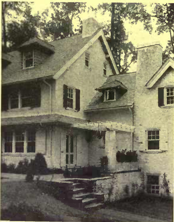
A loosely laid brick walk running before the house lends a touch of warm color consistent with Colonial houses
