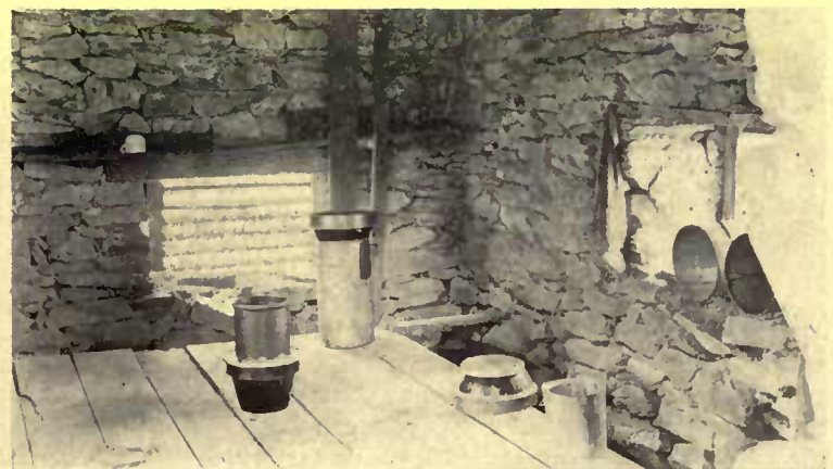
A wooden platform may be used instead of cement flooring in the spring house. The water flows around this raised portion
