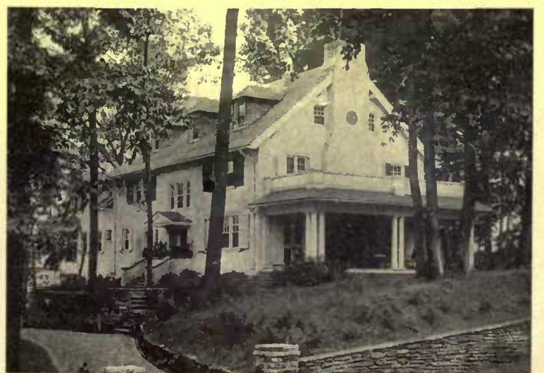
Both front and back are equally attractive in finish. Here the straight stairway ends in a terrace landing that serves as a porch
