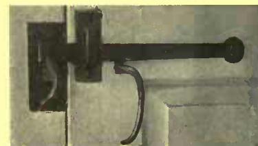
An inside latch lifted by an iron lever
