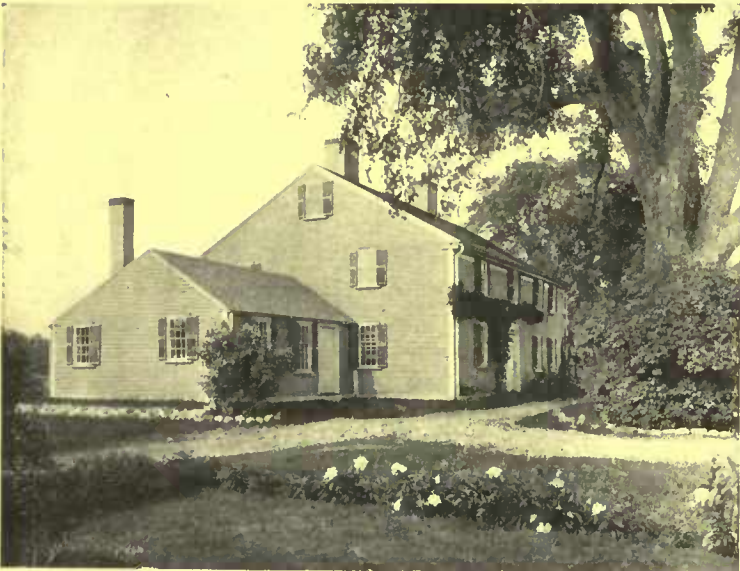
The original lines were very little modified in changing the house, and the surface was easily restored
