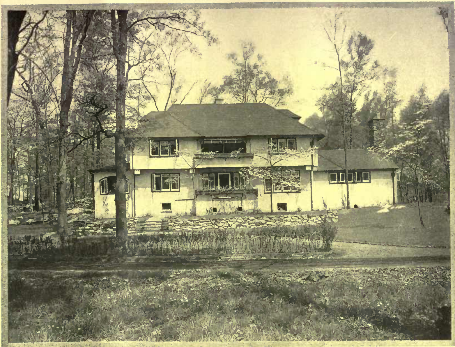
Mr. Wurzburg's house is of stucco with brown trim except that the casement sash are painted white. The house shows particularly good treatment of the sleeping porch. It is an architectural feature and not an excrescence as is so often the case. W. A. Bates, architect
