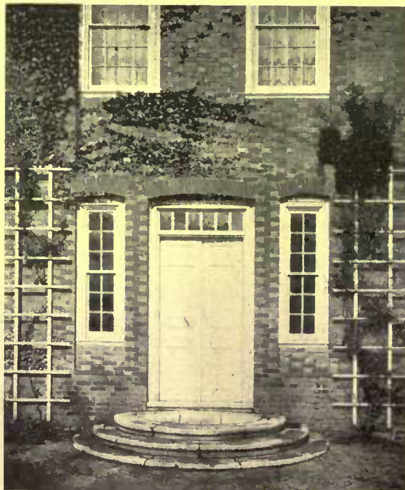
The Stenton doorway is very simple for a Colonial house, but there is an attraction in the flattened arches
