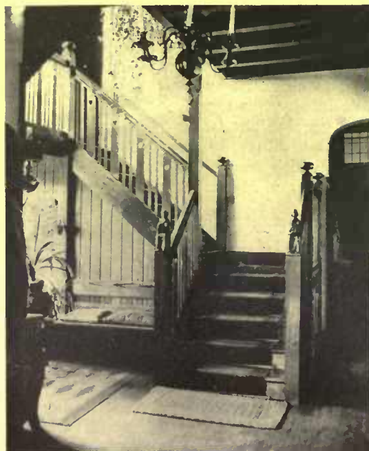
A staircase in which an interesting touch is added by the carved figures on the newel posts
