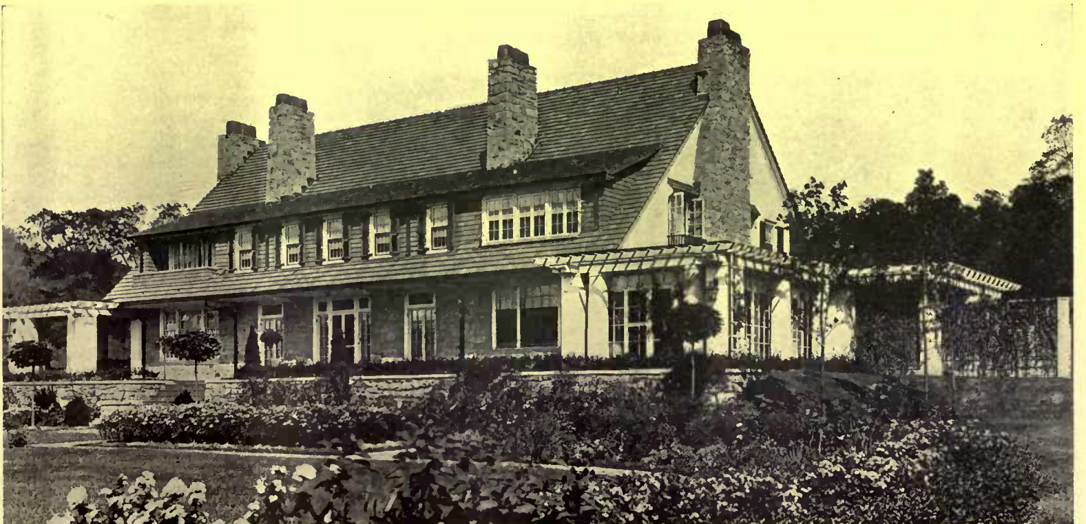
Throughout the Graham house are many modern ideas worth adopting. The garden side has the greatest sweep of roof, which bridges over a terrace forming a porch. The treatment is more informal than the street side and rough stones are used instead of the stucco finish. Privacy is thus insured for the intimate life of the inmates
