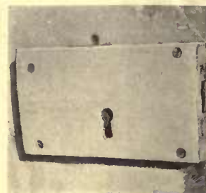
The surface lock often was covered with a wood box
