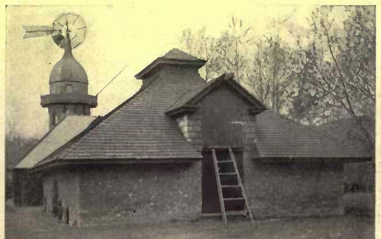
A variation of the frame ice house that is shingled throughout and in quite good keeping with the other outbuildings around it
