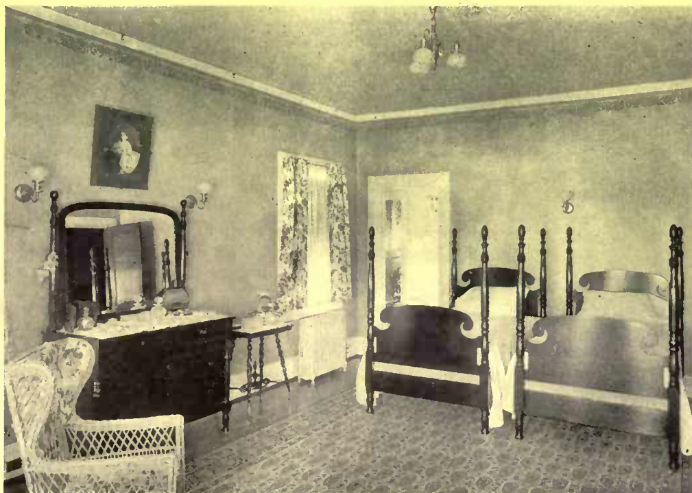
In the bedroom also the walls were plaster finish and painted and an attractive stencil border in two colors giving results as striking as a printed paper frieze but more durable
