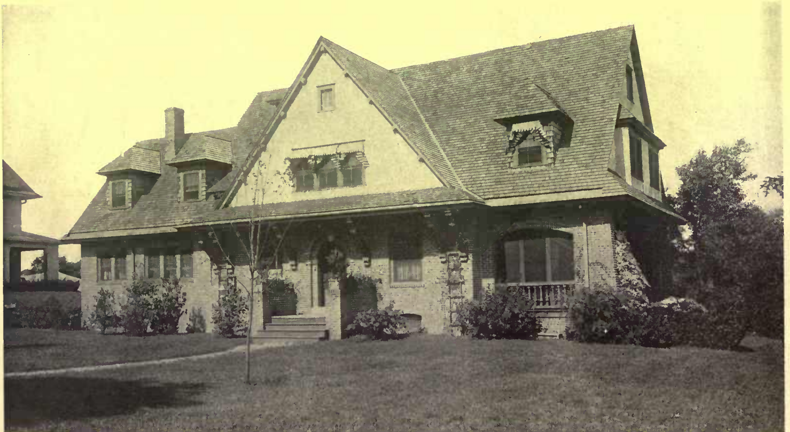
The porch is really an integral part of the house and is patterned on the idea of the Italian loggia. It allows the porch to be built beneath the upper stories of the house without giving the effect of insecurity so often seen
