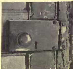
The old time brass surface lock was attached thus
