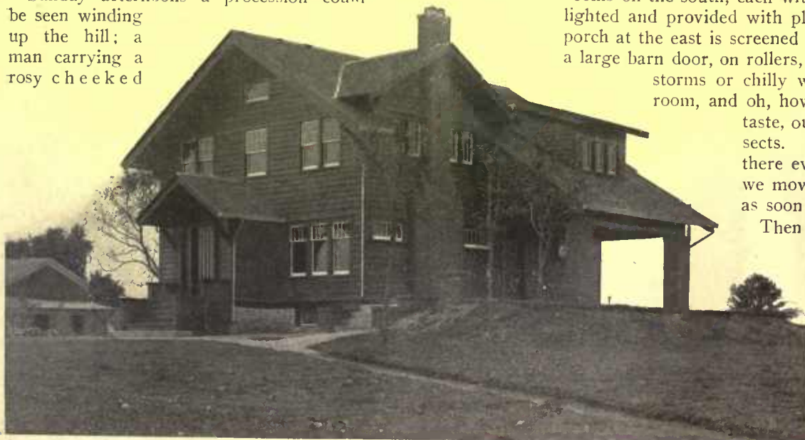
Living on the ground gave an excellent opportunity to oversee the building work and made us appreciate the house still more for our early acquaintance with it
