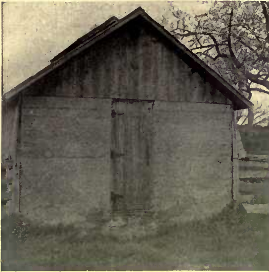
The grout style of field stones bound together with concrete is very durable and keeps ice well
