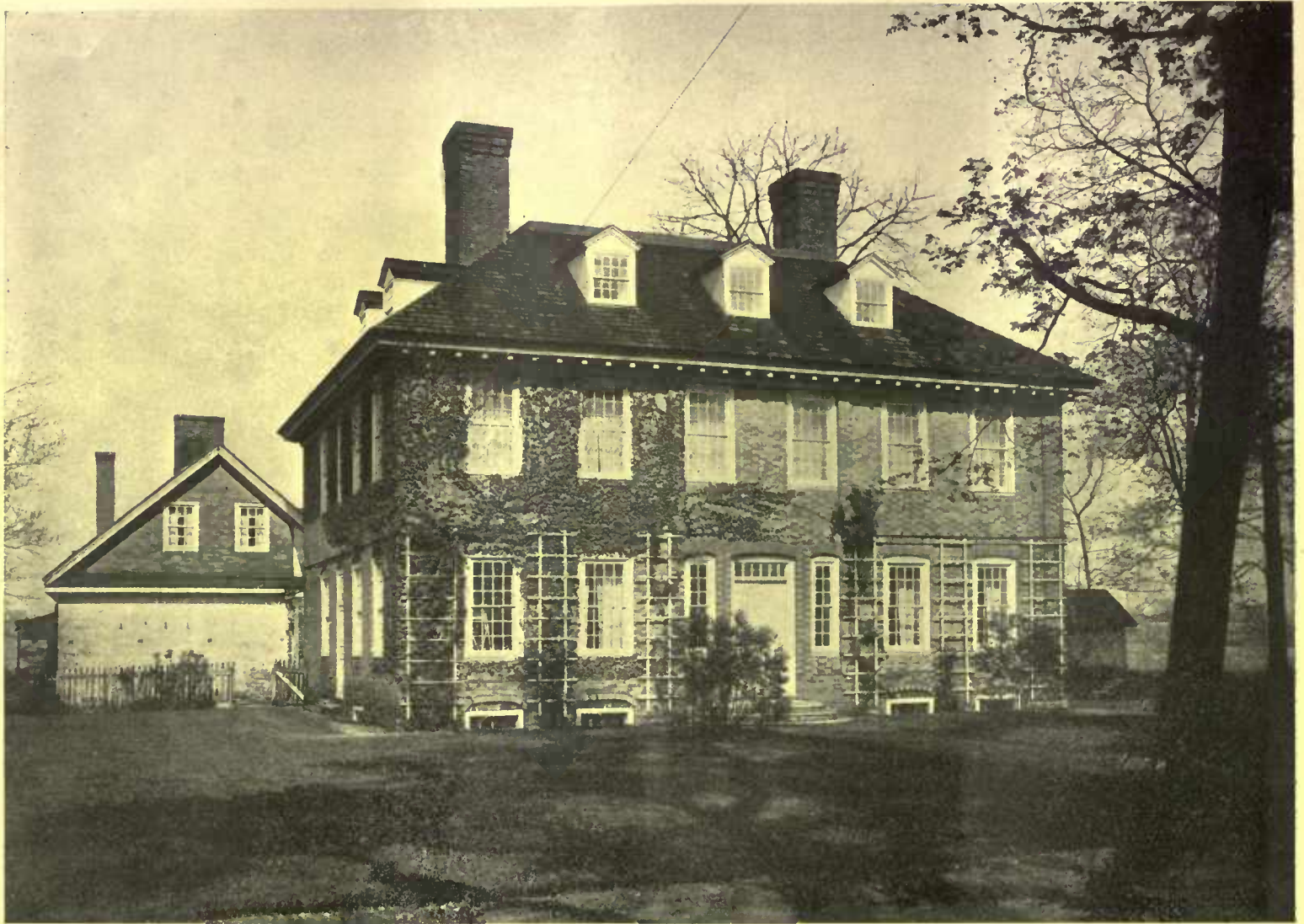
Stenton shows the best preservation of many of the Colonial houses about Philadelphia. It is interesting for its simplicity and the excellent use of Flemish bond and brickwork. There is very little decoration beyond the cornice at the roof line, but the house has a decided charm.
