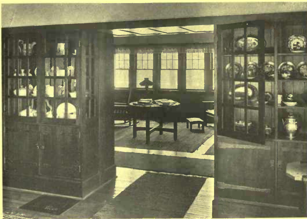
The china closet became the nucleus of a partition between the dining- and living-rooms. On one side are the china cabinets; on the other, bookcases of similar size and design
