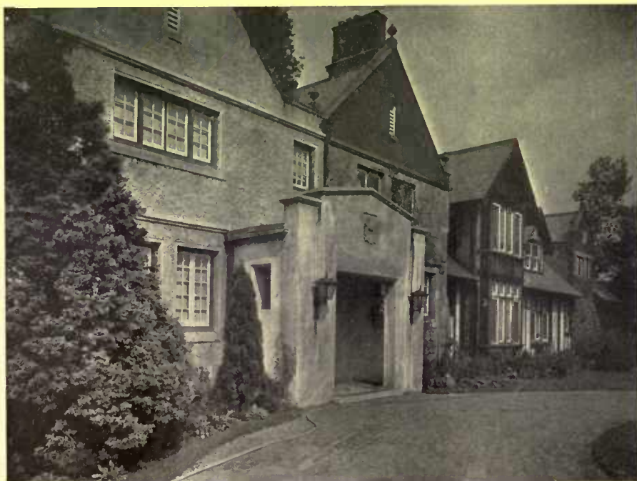
Stone and stucco combined in this way suggest different periods of growth
