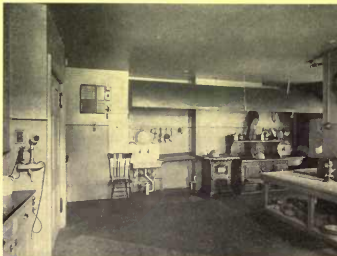
This complete kitchen offers suggestions in its table against the wall and wide hood covering the sinks as well as the stove
