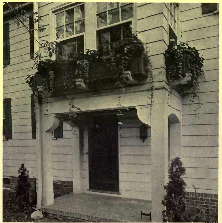
The jutting beams which here support the boxes are in themselves true architectural features of the house
