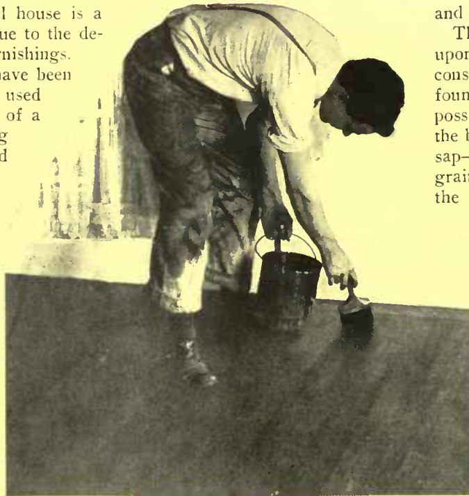
When shellac is applied to the floor it is essential that it be evenly distributed. If necessary, thin out with wood alcohol
