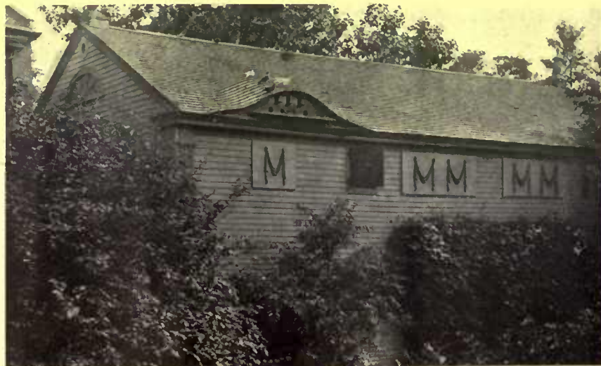
An old barn utilized the vacant attic space by curving the roof over the dovecote. The birds can be reached from inside
