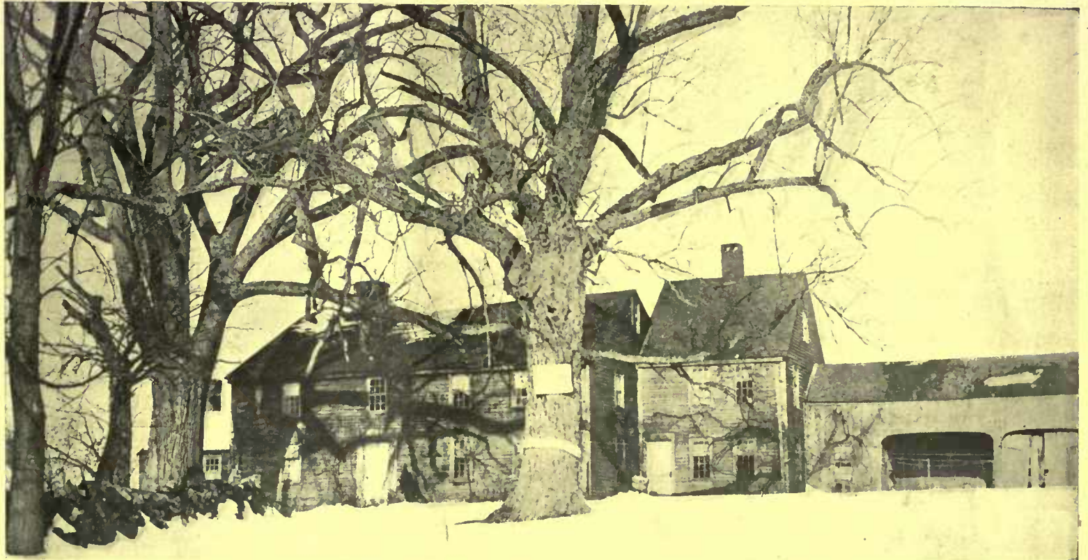
Beneath this shabby exterior Mr. George C. Wales saw great possibilities to restore the house. One ell too far gone to be restored was replaced by a new one; otherwise the original building was unchanged
