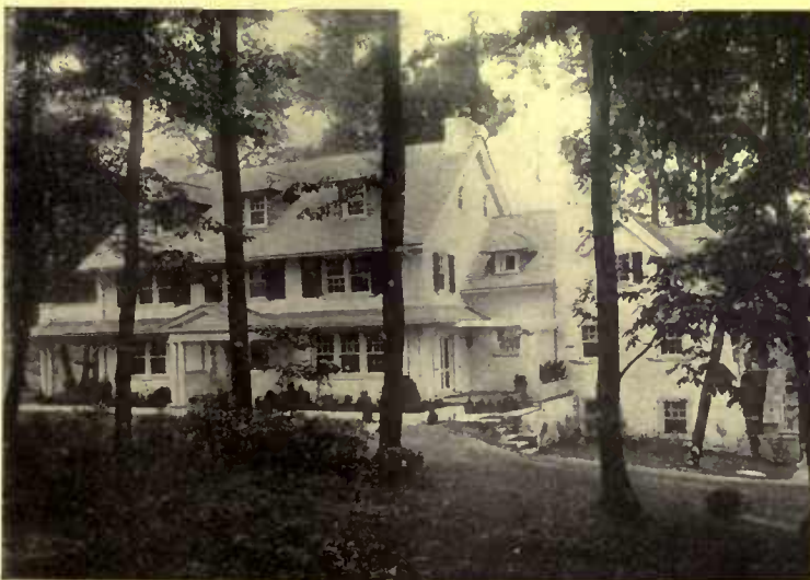
The rough stone walls have been coated thinly with stucco, which gives a uniform color and a satisfactory and pleasing surface
