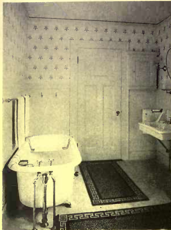
The bathroom was finished with a waterproof white paint that served just as well as tiles
