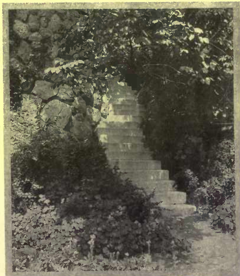
Although these steps are an attractive feature in this garden, their ascent is so steep that they will always be uncomfortable to climb
