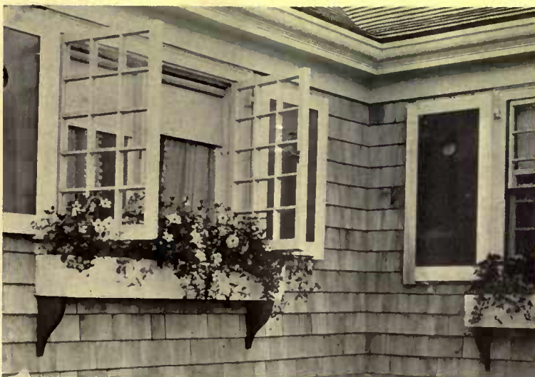
When placed outside of casement windows the box should not be too close if the windows are often opened and closed
