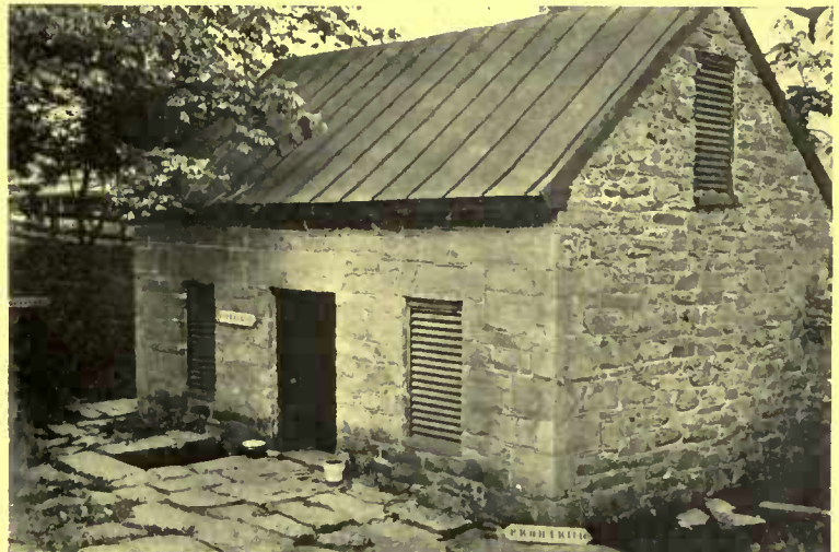
Heavy fixed slats for windows allow a circulation of air and the thick stone walls help to maintain an even temperature
