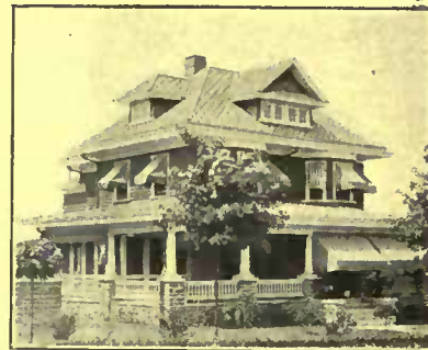
Residence of Mrs. Kircher, Lanerch, Pa. Covered with J-M Transite Asbestos Shingles.
