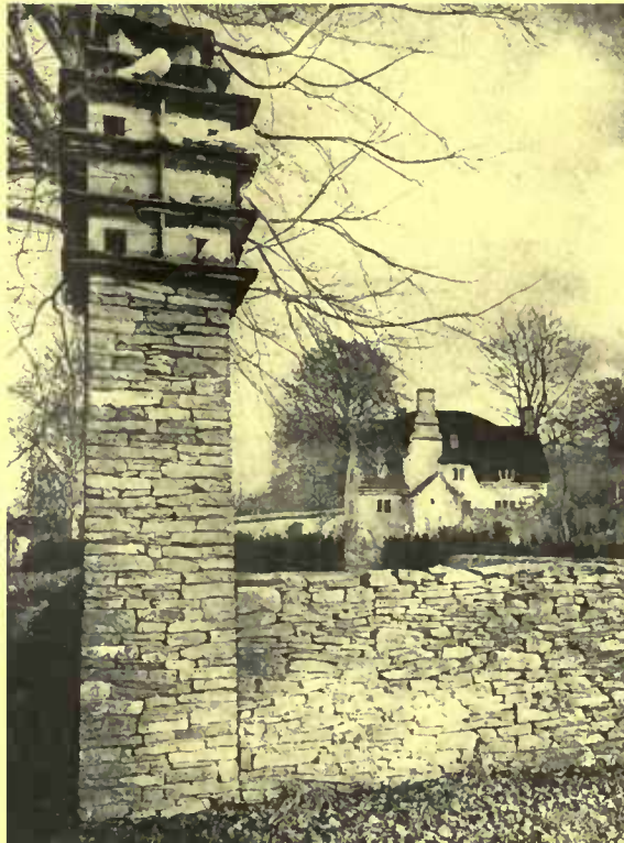
By building a tower at the end of a stone wall a satisfactory and picturesque dovecote was made
