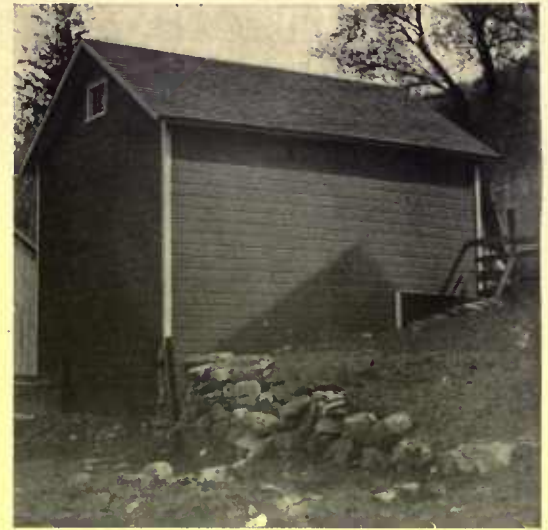
If set in a hillside the ice house may be filled from the upper side with less labor
