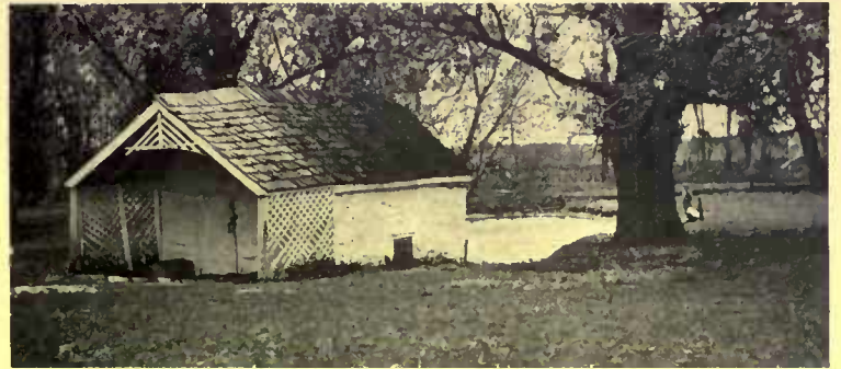
The spring house usually has a projecting roof which protects the spring besides forming a sort of porch
