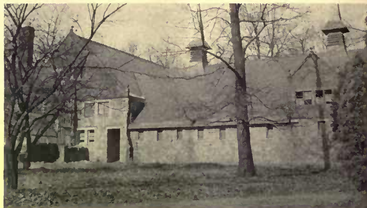
The stable originally appeared like this. At the extreme left the conservatory may just be made out. Behind this the wall was of brick
