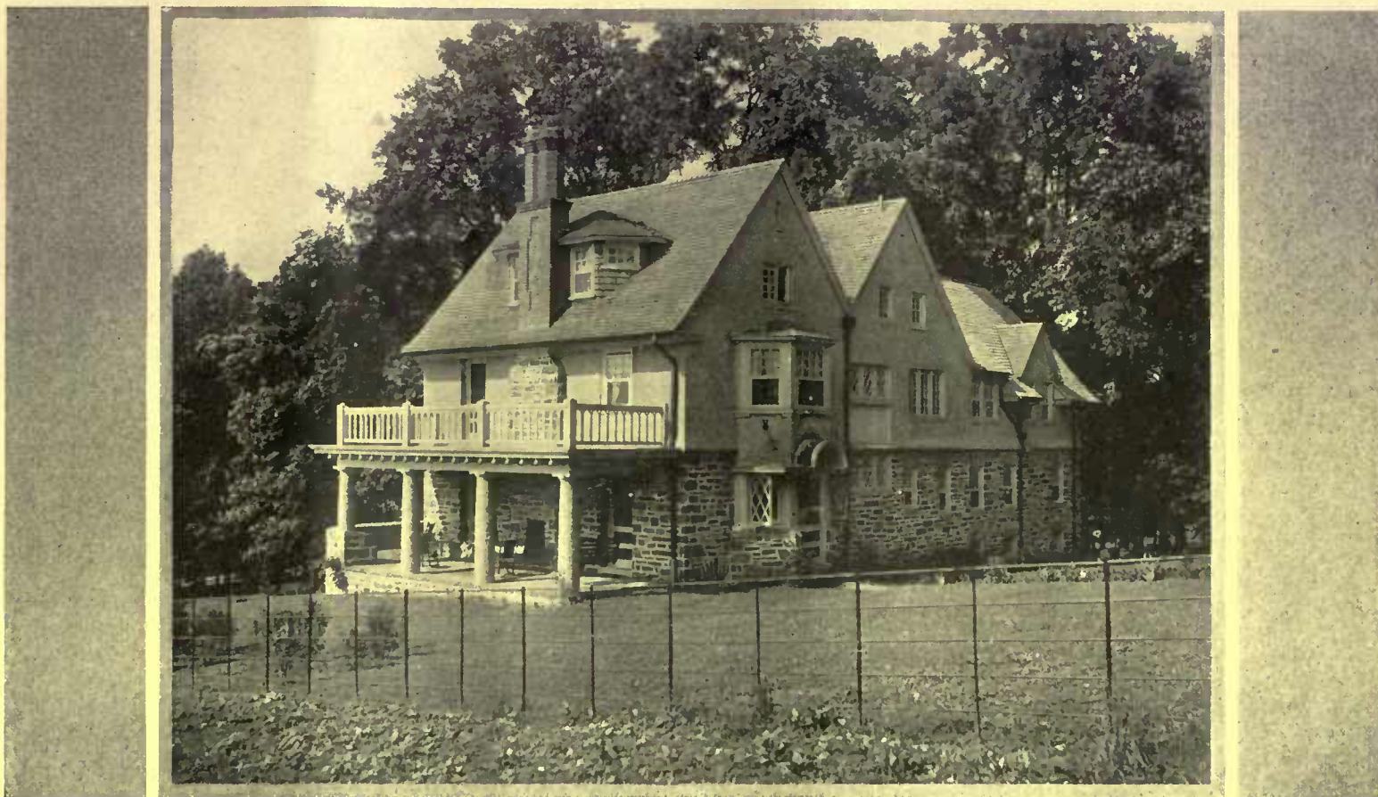
The Germantown stone that is the logical building material in this section is used for the first story of the house. The upper stories are covered with rough cast stucco that blends well with the general tone of the exterior. The double-gabled roof is very common to England and is a pleasing variation from our common style
