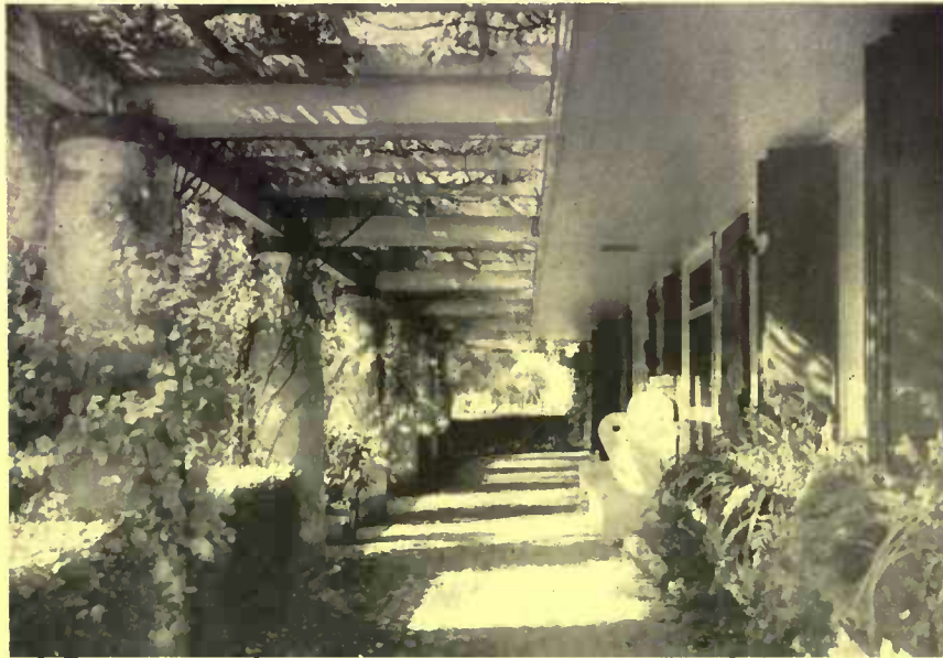
One way of admitting plenty of light and air to the wide porch is to have part of the roof open save for the girders over which vines grow
