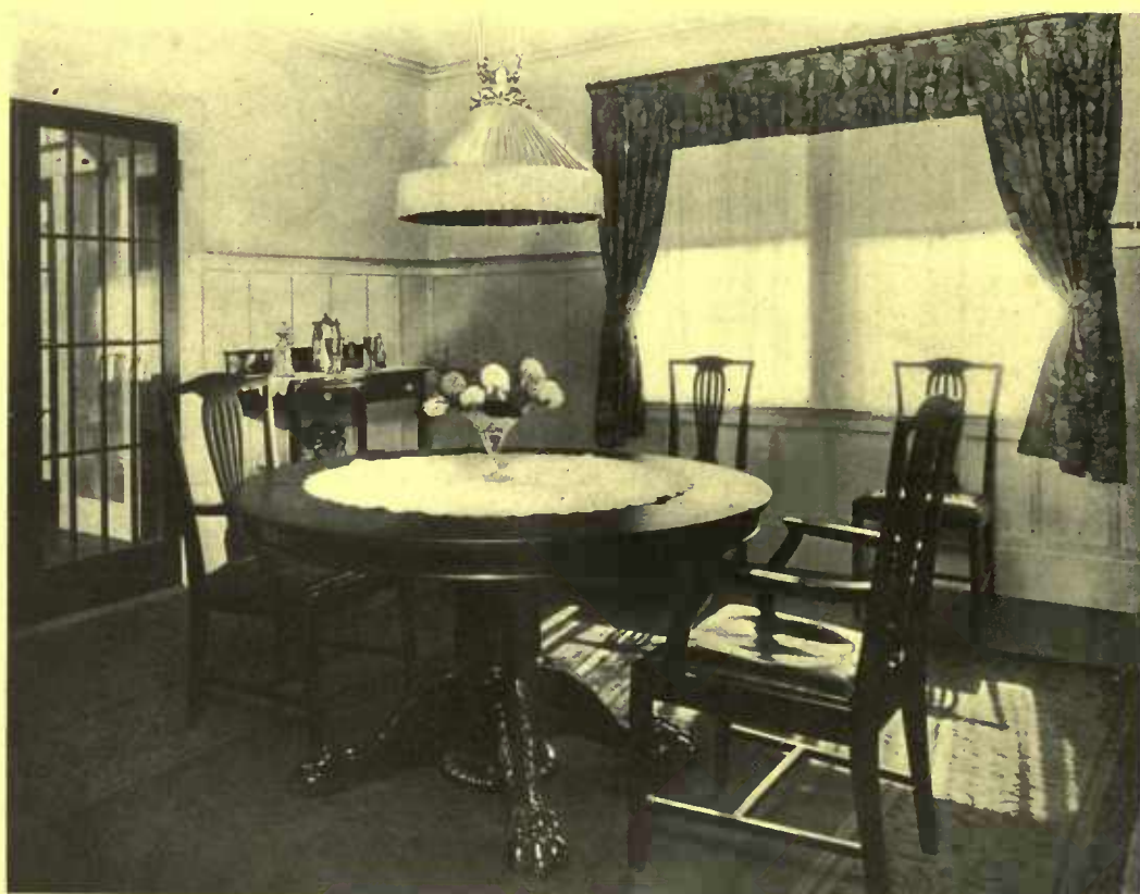
In this dining-room a wood wainscot effect was created by connecting the plate rail and the baseboard with wood strips. Give both wood and plaster a generous coating of enamel
