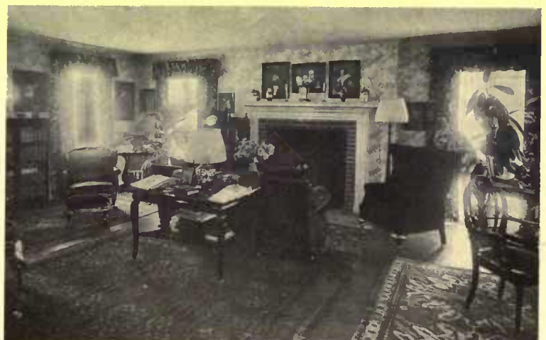
In the living-room of this house the mantel consists of a simple molding treatment of cornice without carving. The combination with the brick is effective
