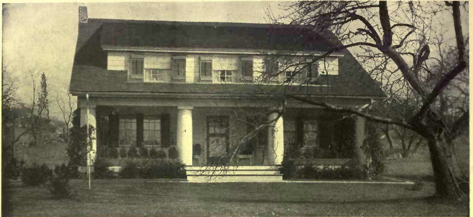
Mr. Wood's house is of the American farmhouse type rapidly gaining in popularity here. In general it is a variation of the Dutch gambrel roofed style, affording more porch room and greater ceiling space above stairs. The long porch boxes filled with evergreens are particularly effective
