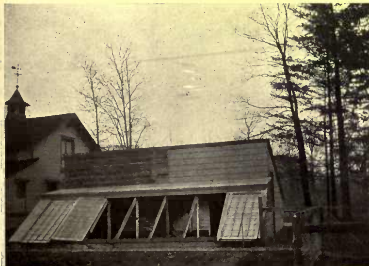
A sunken path in this greenhouse-coldframe allows one to work comfortably at the waist-high beds
