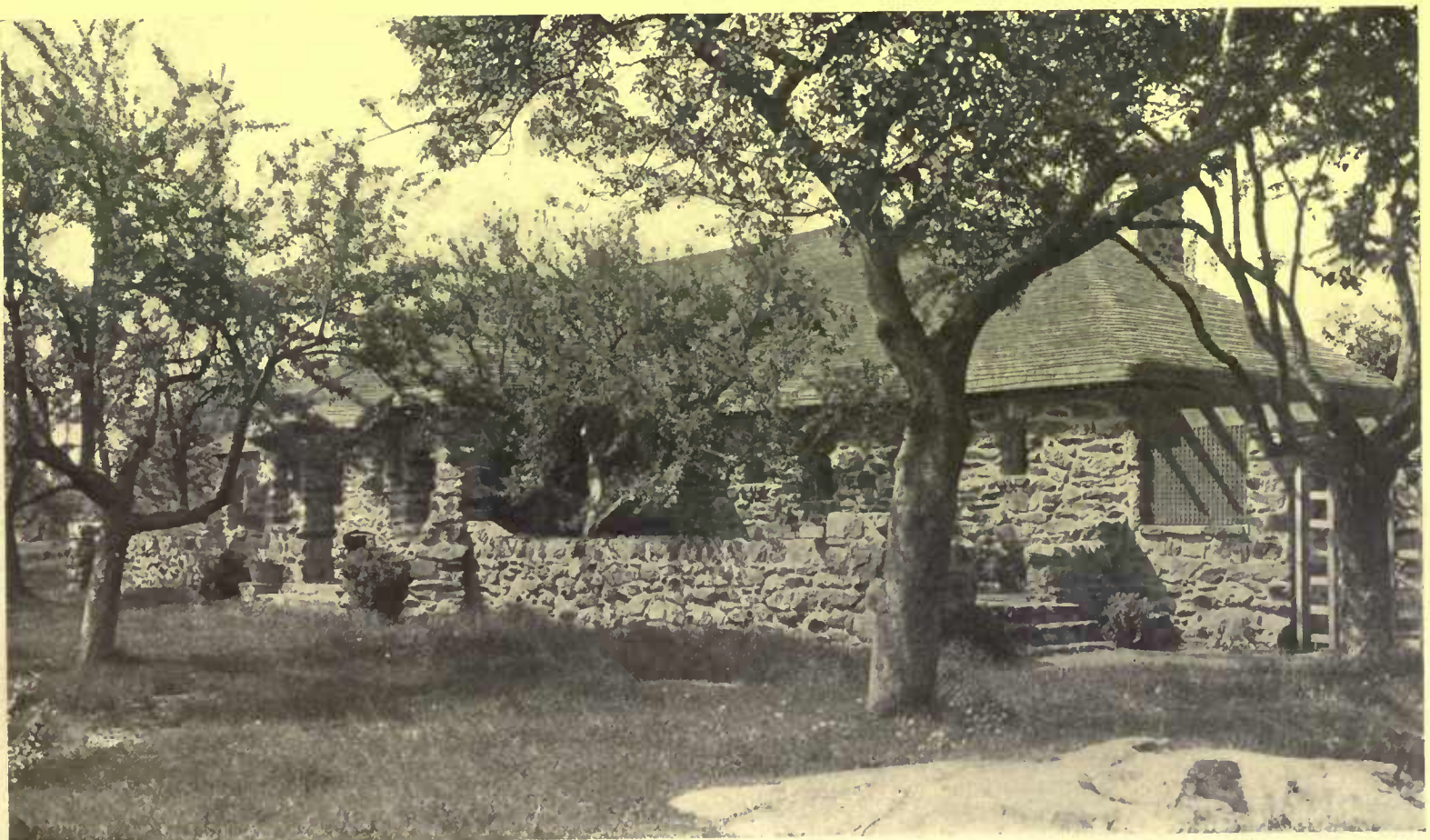
Field stone is the logical medium for the small house in many locations and it is seldom used to better advantage than here. Many of the stones gathered nearby show a fine sense for color effect in their various shades, which add an agreeable warmth to the surface
