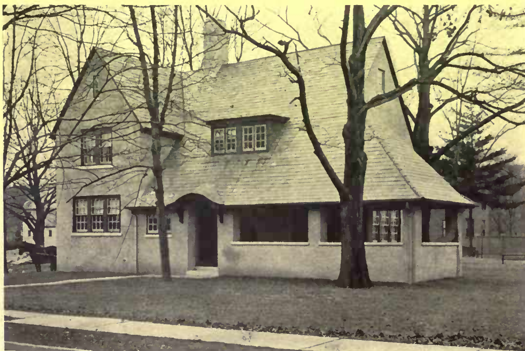
Separate porch roofs may be avoided in such designs as permit of the main house roof being extended to cover the porch
