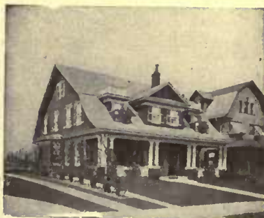
Residence of Joseph M. Dale, Asbury Park, N. J. W. C. & A. F. Cottrell, Architects.
