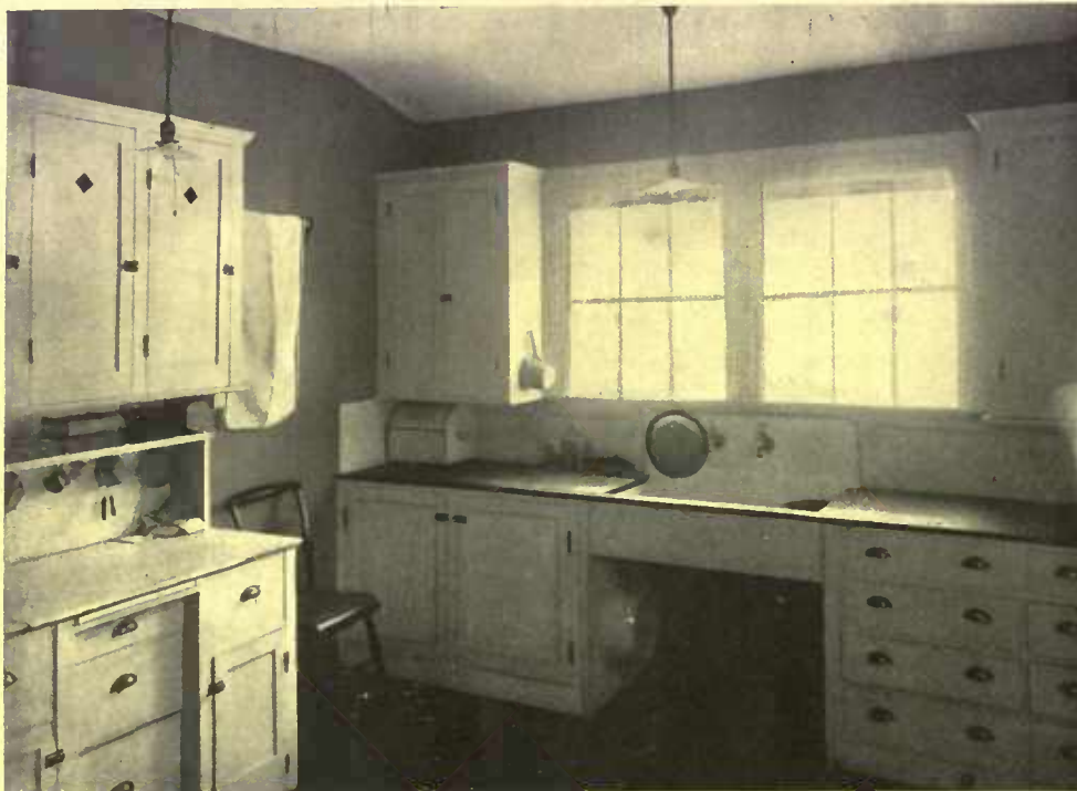
A well-lighted sink is desirable for comfort and efficiency. The space directly below it should be left open, thus making for greater cleanliness
