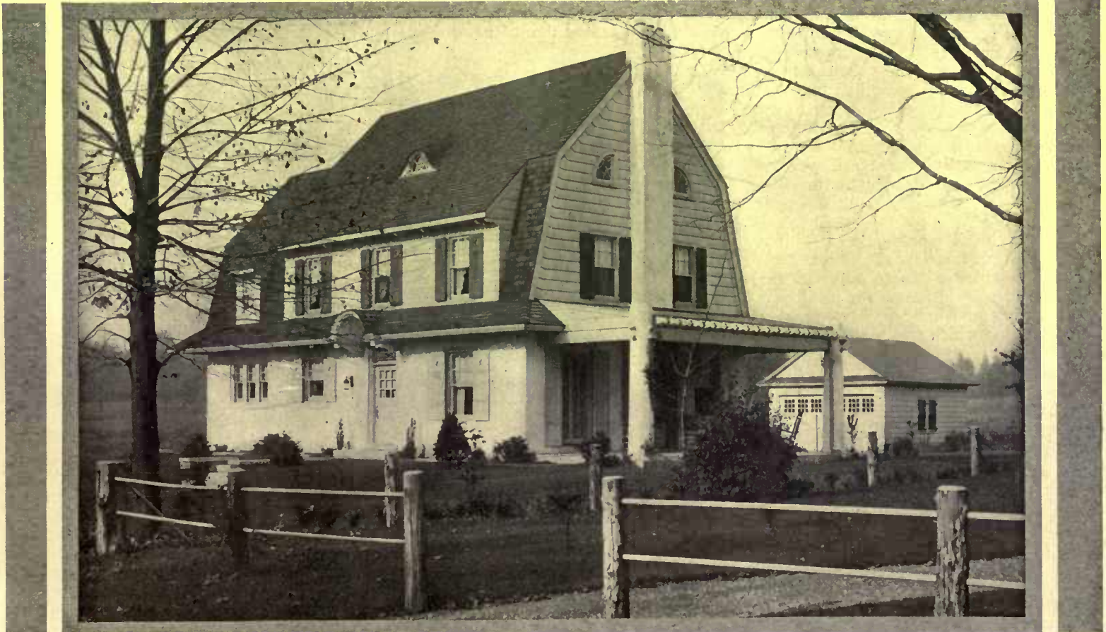
At one end the hip roof is extended into a porch roof supported by heavy stucco columns. French doors open onto a porch floored with tiles and having an outdoor fireplace connecting with the main chimney
