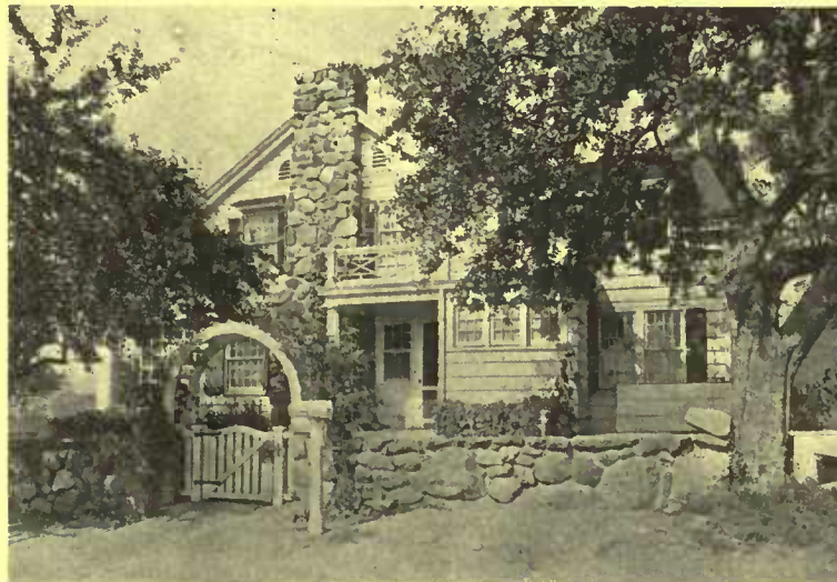
Where the house above is cut off slightly in back of the chimney, a kitchen wing has been built on this superintendent's cottage to provide for the needs of the help on a large estate. The side view is not spoiled by any means with this addition
