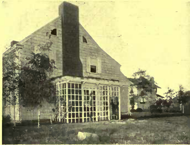
On the small place a lattice work screen may be built about the doorway. This pergola can be used to support vines
