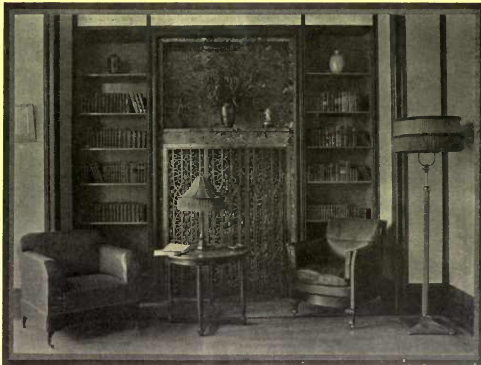
There is a good example here of how the radiator may be so placed that when covered it is a decorative unit. The screen of wrought brass is an example of the best German work. As there is polished marble above the radiator no dust can settle
