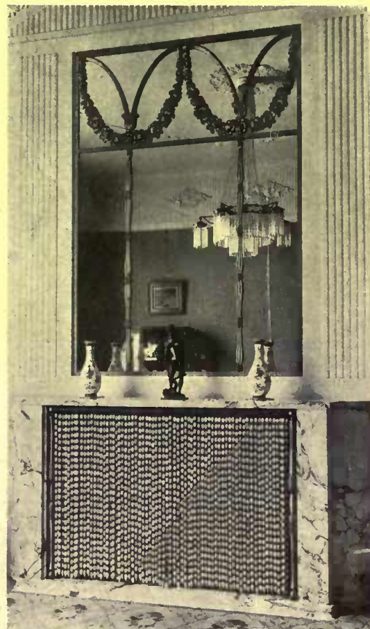
In many finely decorated rooms a curtain of strung beads serves to hide the heating pipes
