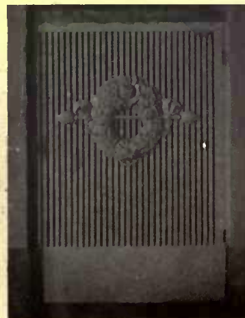
A wooden radiator cover set in the wall between two rooms
