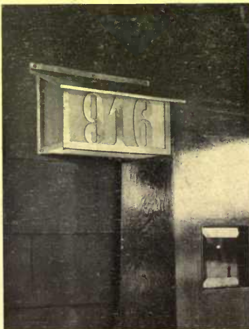
An electrically illuminated house number serving also as porch light
