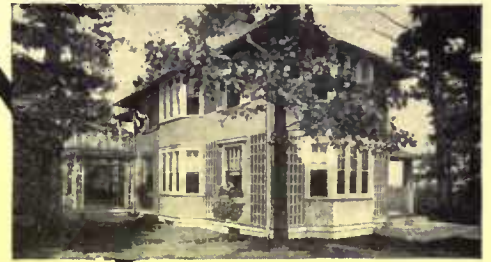
Residence of L. R. Hoff, Patterson, N. J., roofed with J-M Transite Asbestos Shingles. F. J. Parsons, Architect, New York.
