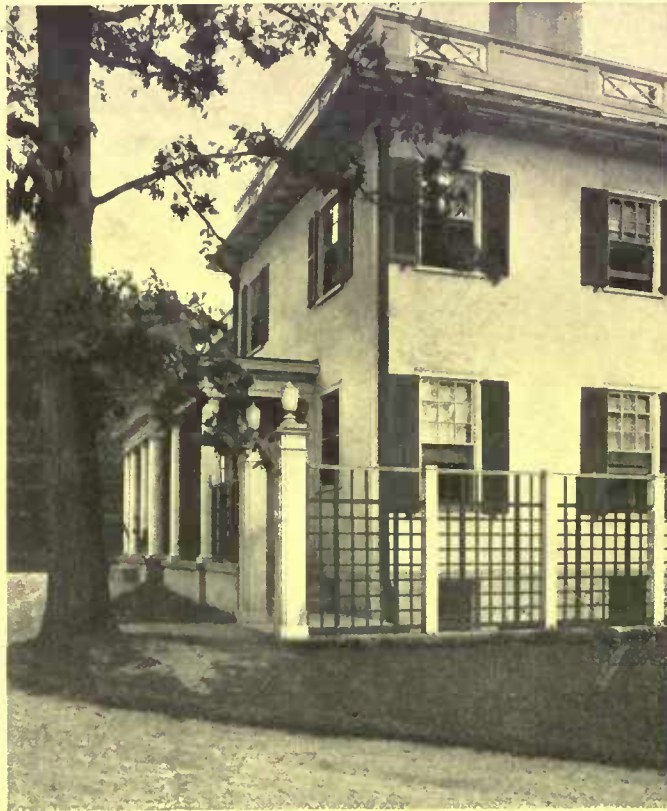
Even the formal type of house finds use for lattice. This dignified screen takes away from the ugliness of a basement area
