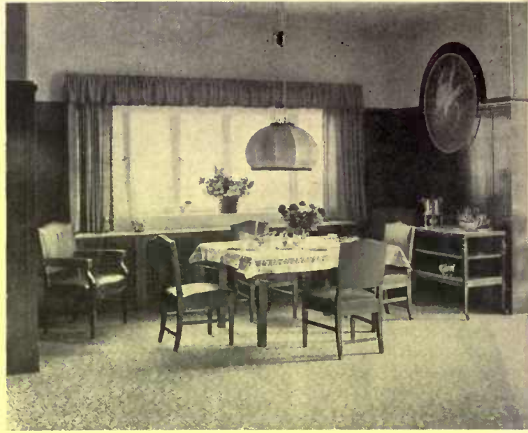
Since the air is coldest at a window, the most advantageous place for a radiator is beneath the window sill. Here a lattice work hides it
