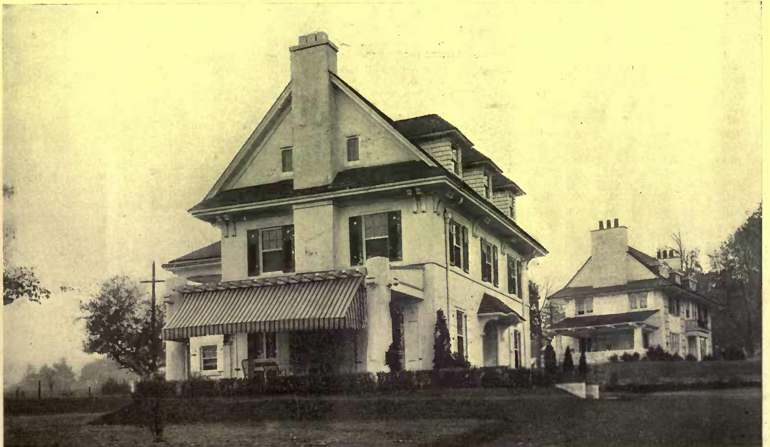
A deep green stain on the shingles is fitting with the stucco finish. The blinds are also green and the putty beads on all the window panes are painted black, which enhances the brilliancy of the glass. There is a rough stone fireplace on the porch
