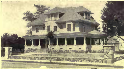
Residence of Mrs. Clara F. Taylor, De Land, Fla. Roofed with J-M Transite Asbestos Shingles.
