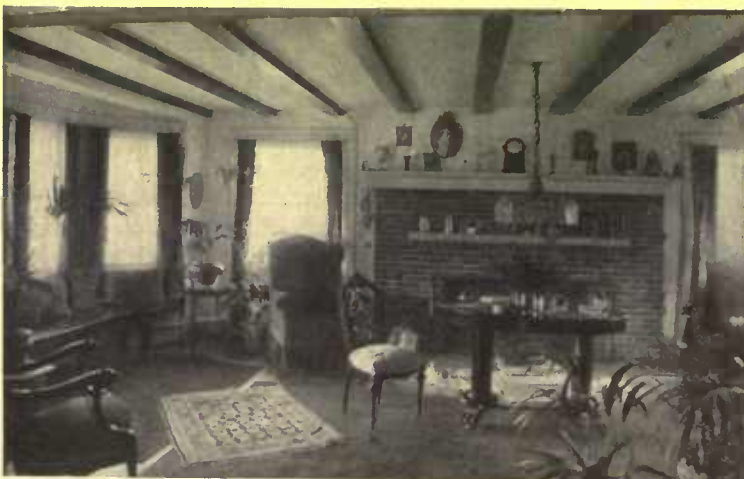
The long living-room is provided with a beamed ceiling of flat timbers as was found often in Colonial houses. The spacious fireplace makes the room homelike
