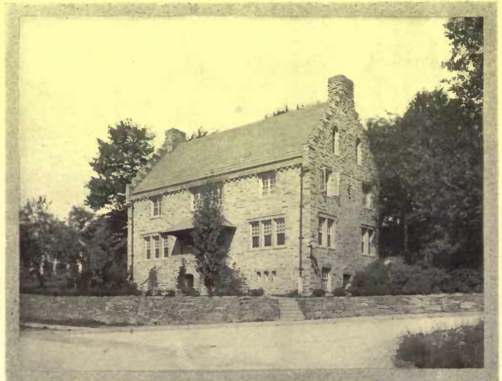
The first story is at the top of the old ice house foundation, necessitating a flight of entrance steps. In this way the basement is almost entirely above ground
