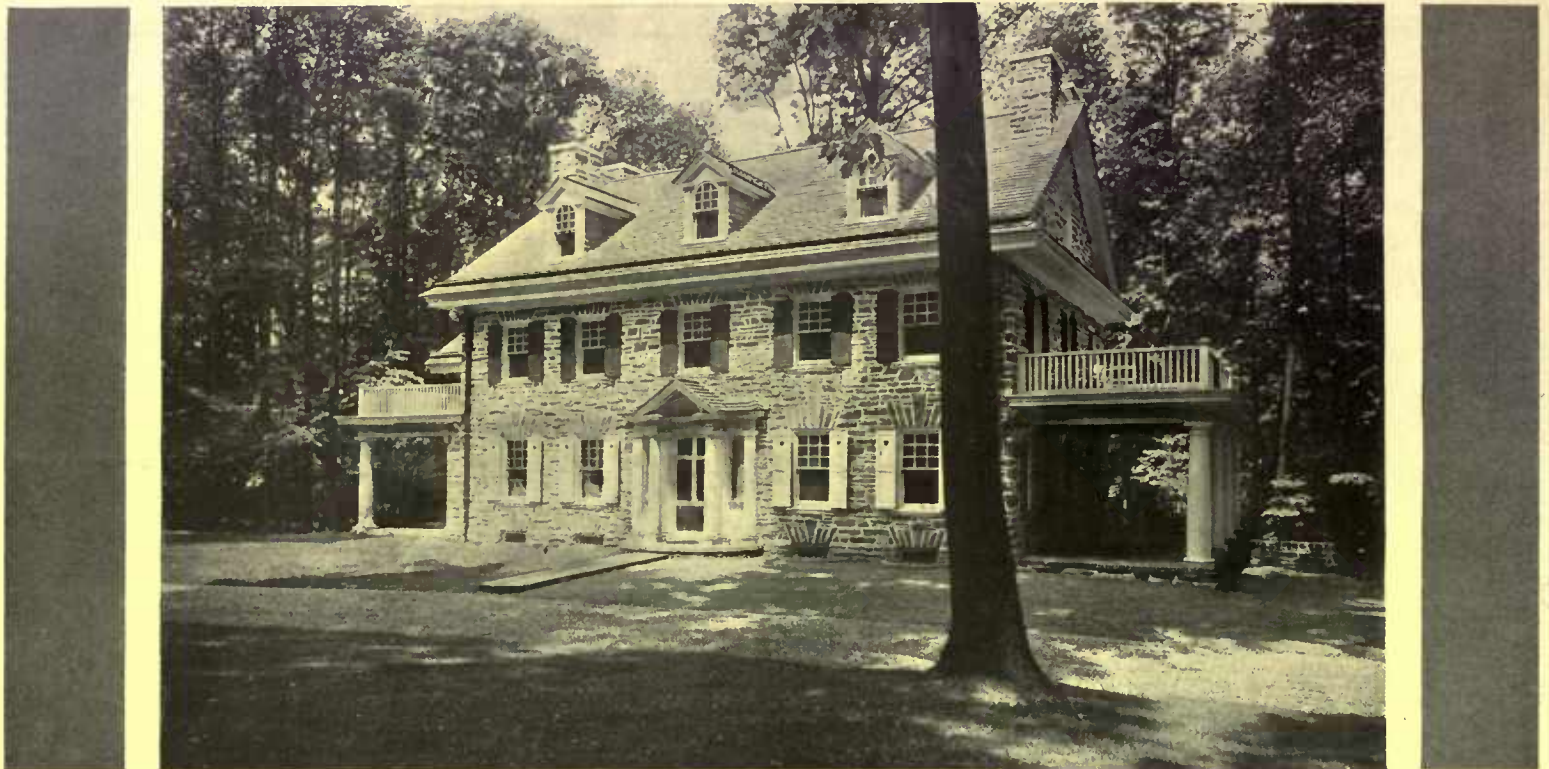
Mr. Vaux's house is built of fieldstone found in the neighborhood and laid with white mortar joints. There is a hip to the roof projecting about the house common to many homes in this neighborhood. Here its strong, horizontal line decreases the apparent height
