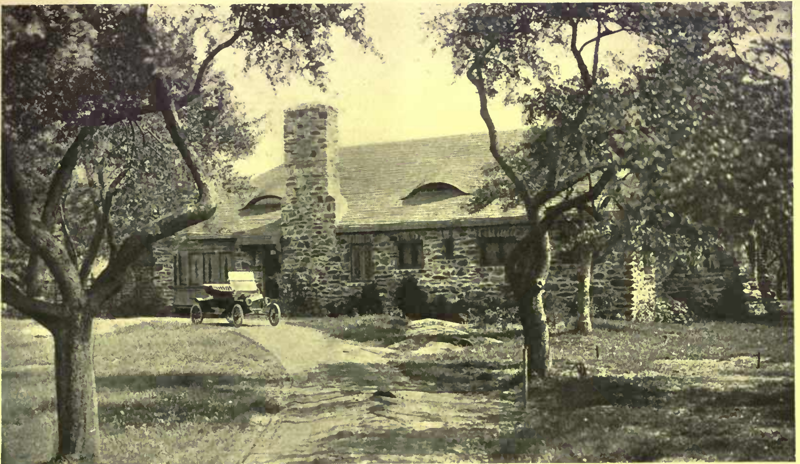
Mr. Selsor's house shows a very happy use of shingles laid to imitate thatch. The fitness of his home to its site is shown very well here where the outcroppings of native rock in the foreground appear almost to be roots of the building extending into the ground
