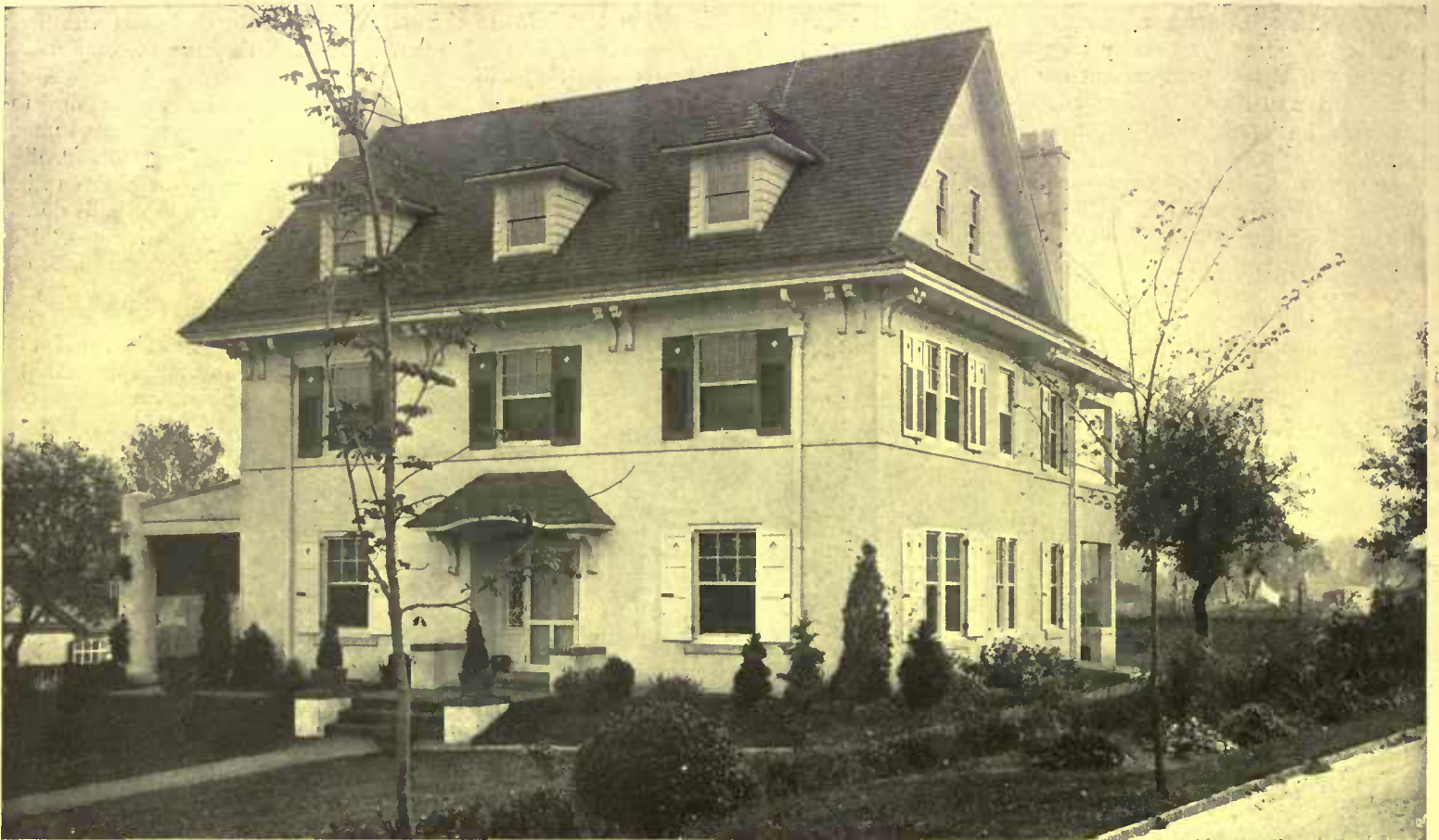
Mr. Shrigley's house is a good example of hollow tile construction, twelve-inch blocks being used on the first story and eight-inch above. To finish this, plaster and stucco are applied directly to the tile. In the floors of the entrance vestibule and the porches hollow tile and concrete were used and finished with cement
