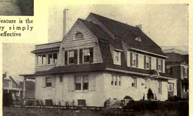
Adding sash to the window openings of the screened porch makes it a winter bedroom; as it is it may serve as a sleeping porch
