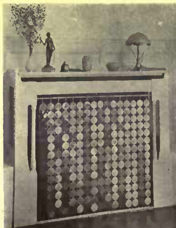
Thin metal plates hung on wood screen a radiator
