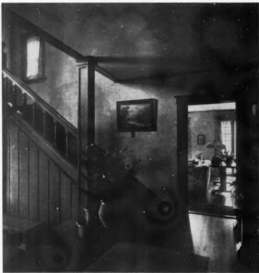
Although in this instance the stairs were built open, it suggests a possible treatment for stairs that have been boxed in, a change worth considering in remodeling an old house
