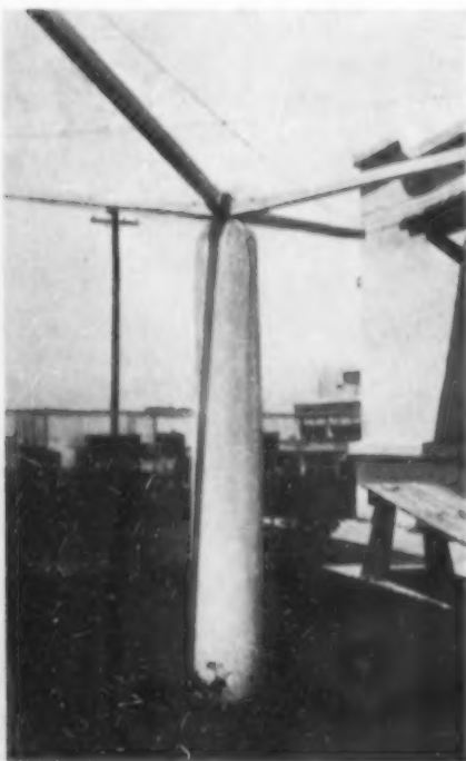
A substantial post for the clothes dryer was made of concrete, to be later planted with honeysuckle
