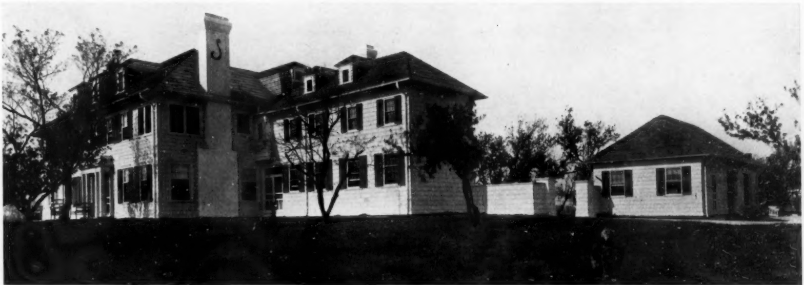
The wall, shingled in like the house and garage, connects the two, tying the group into a pleasing, congruous whole, and carrying out the single direct lines to the best advantage. Note also the small bay in the angle and the roof treatment
