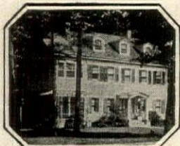
Residence at Plainfield, N. J. Redwood siding painted white
