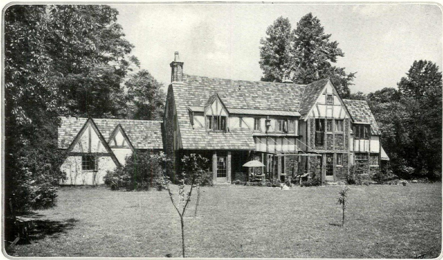
In this house at Scarsdale, N. Y., the architect, being the owner as well, has indulged his fondness for early building methods and craftsman-made materials. Most of the oak timbers were cut in the neighborhood in 1812
