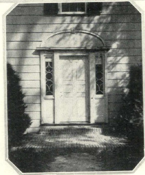
The wooden fans over the door, the two leading lights and the paneling of the door itself are typical Colonial details. D. J. Baum, architect
