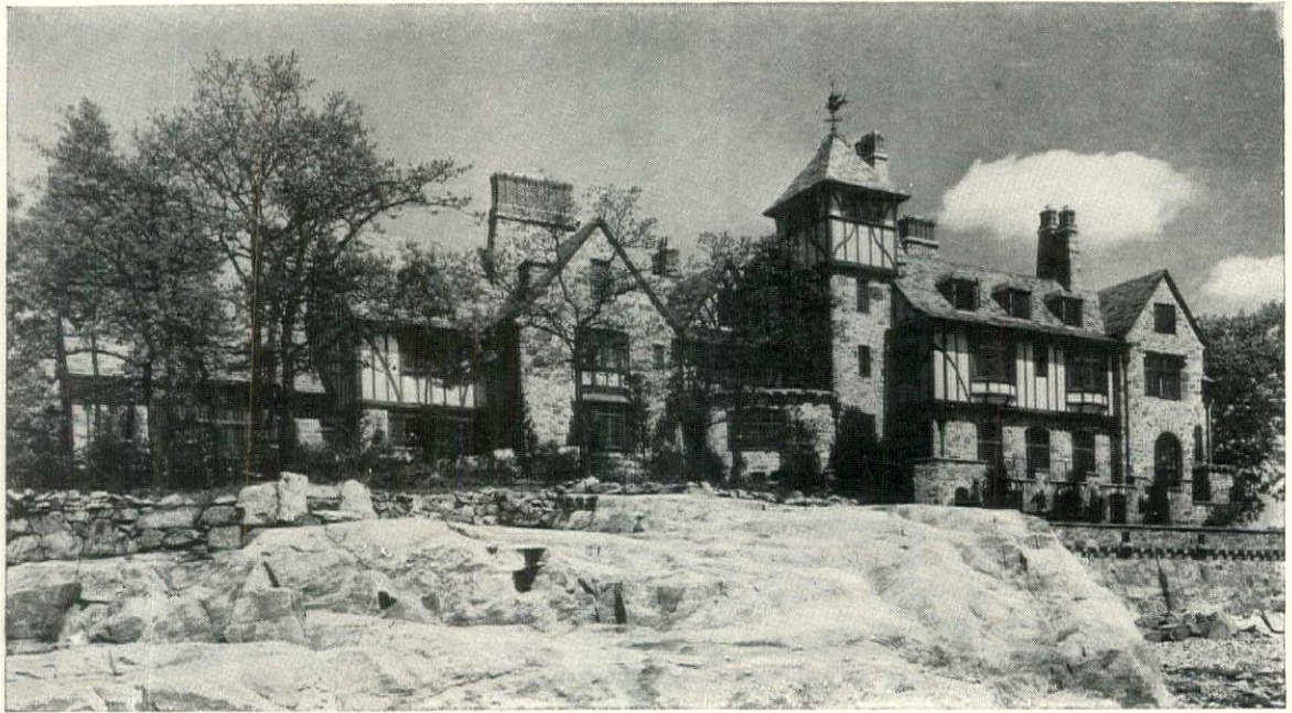
Residence at Greenwich, Conn. Frank P. Whiting, Architect
