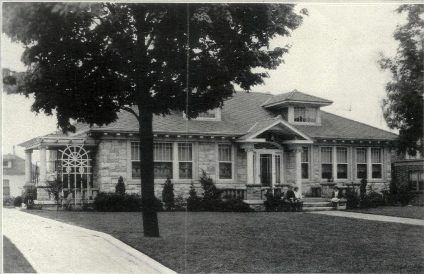
Design No. 401. Bungalow of seven rooms and bath. Faced with a veneer of Indiana Limestone having rough rock finish. A folder showing floor plans will be sent upon request.
