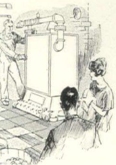
gas—replaces coal boiler or oil burner. New piping is almost never required.
