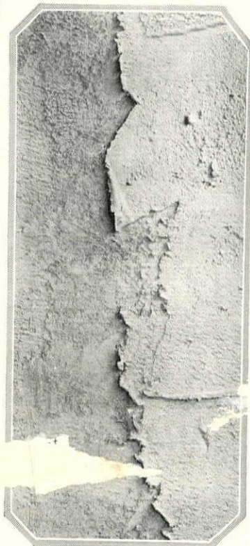
This texture at the right is known as Italian. It is suggested for use in surfacing houses which are simulations of the Italian villa. For such a house the stucco can be very colorful in tone as the Italian homes have colorful walls
