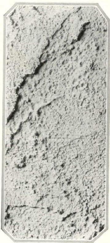
Different textures of stucco have been developed to harmonize the wall surface with the architecture of the house. The texture at the left is suggested for houses coming under the classification of modern Californian
