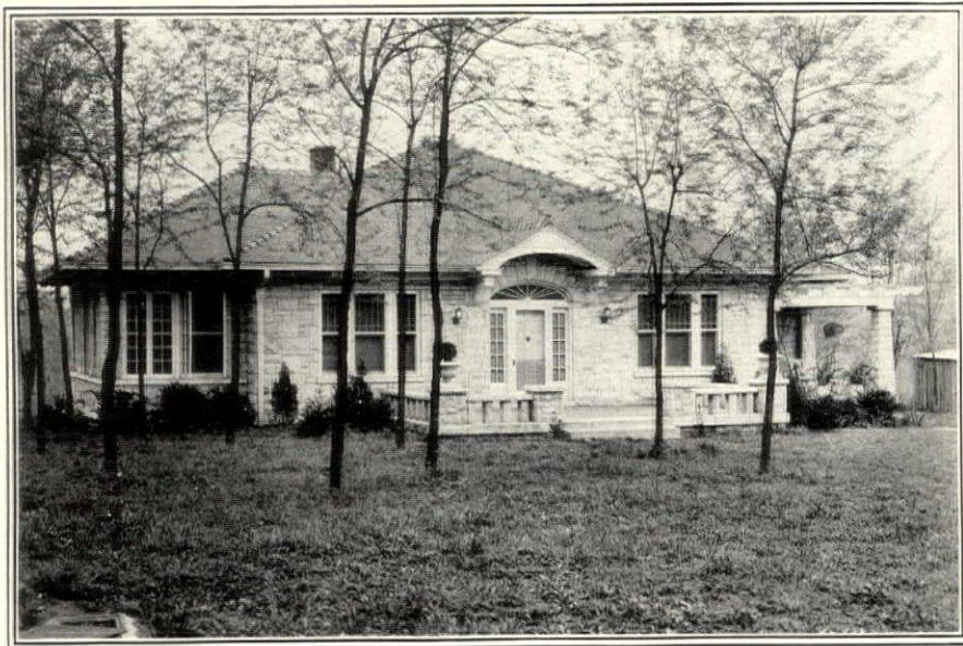
Design No. 403. Bungalow of eight rooms and bath, with both open and covered porches. Faced with a veneer of Indiana Limestone having rough rock finish
