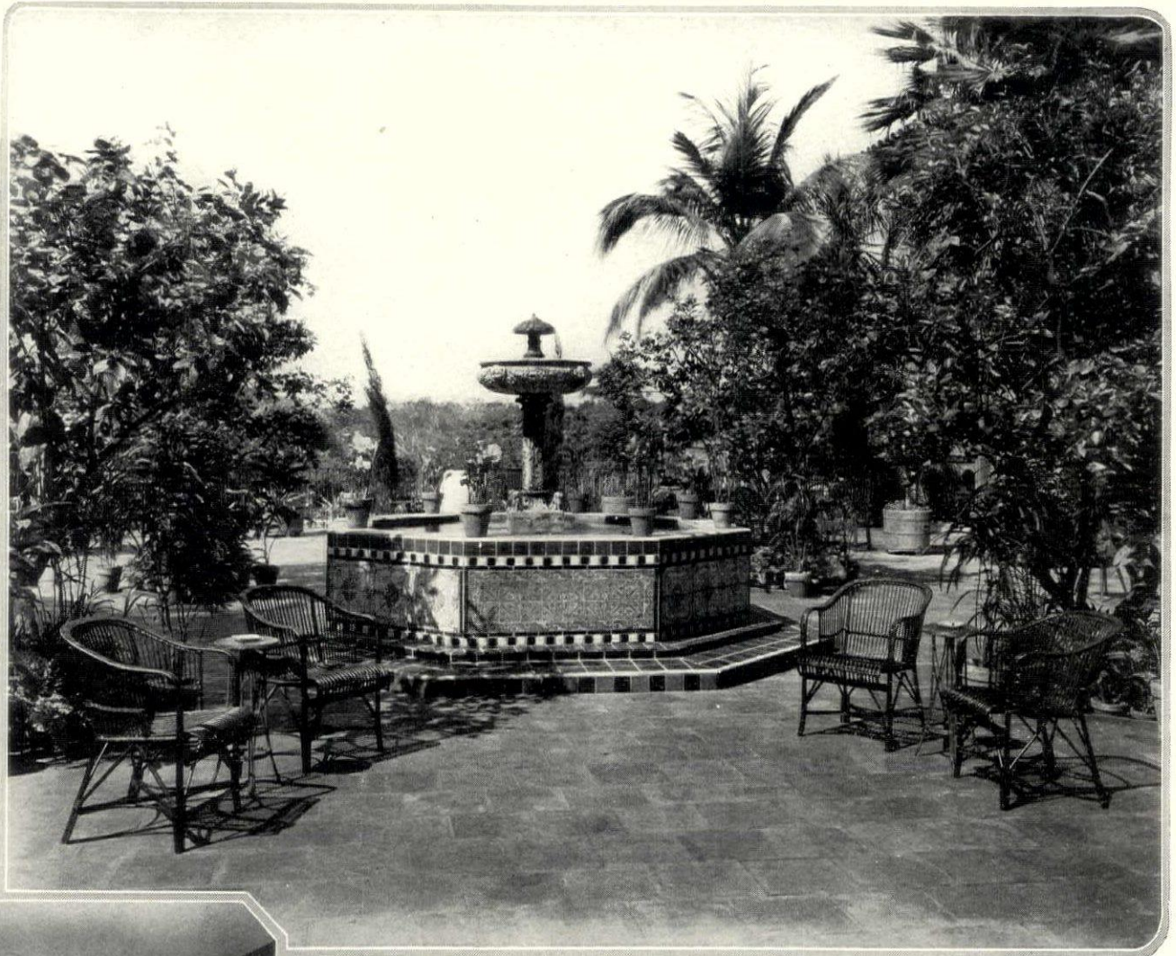
A newly completed garden fountain on the terrace of the Stotesbury house is covered with tiles from a collection Mrs. Stotesbury has been years assembling. Howard Major, Architect
