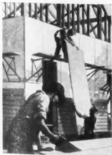
AS SHEATHING Celotex supplies the insulation needed back of brick, wood or stucco exteriors. Here it is nailed directly to the framework in place of the rough boards formerly used, gives greater strength to the house walls and makes building paper unnecessary.
