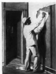
UNDER PLASTER On inside walls and ceilings, plaster is applied directly to the surface of Celotex. This eliminates the use of lath and gives stronger, insulated walls; less apt to crack and free from lath-marks. Plaster bonds with Celotex far tighter than it keys to lath.
