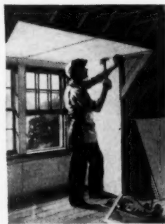
FOR OLD HOUSES In homes already built, a big measure of Celotex comfort and economy may be secured by lining attics and basements with it. In the attic an extra finished room can be made by nailing Celotex to the roof rafters. In the basement line the ceiling with Celotex.
