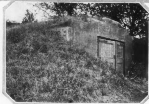
A root and fruit cellar should be built under the frost line
