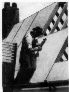
IN THE ROOF Most heat beats into houses through roofs in summer, causing hot attics. Most heat leaks out through roofs in winter, causing high fuel bills. Celotex applied over or under roof rafters gives the needed protection. For best results both uses are recommended.
