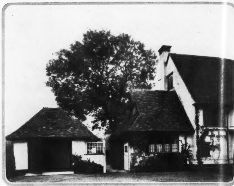
The forecourt of a house near Cambridge, England. The garage is separated from the kitchen by a short wall and gate, yet the garage is planned as an integral part of the design. Harry Redfern, architect
