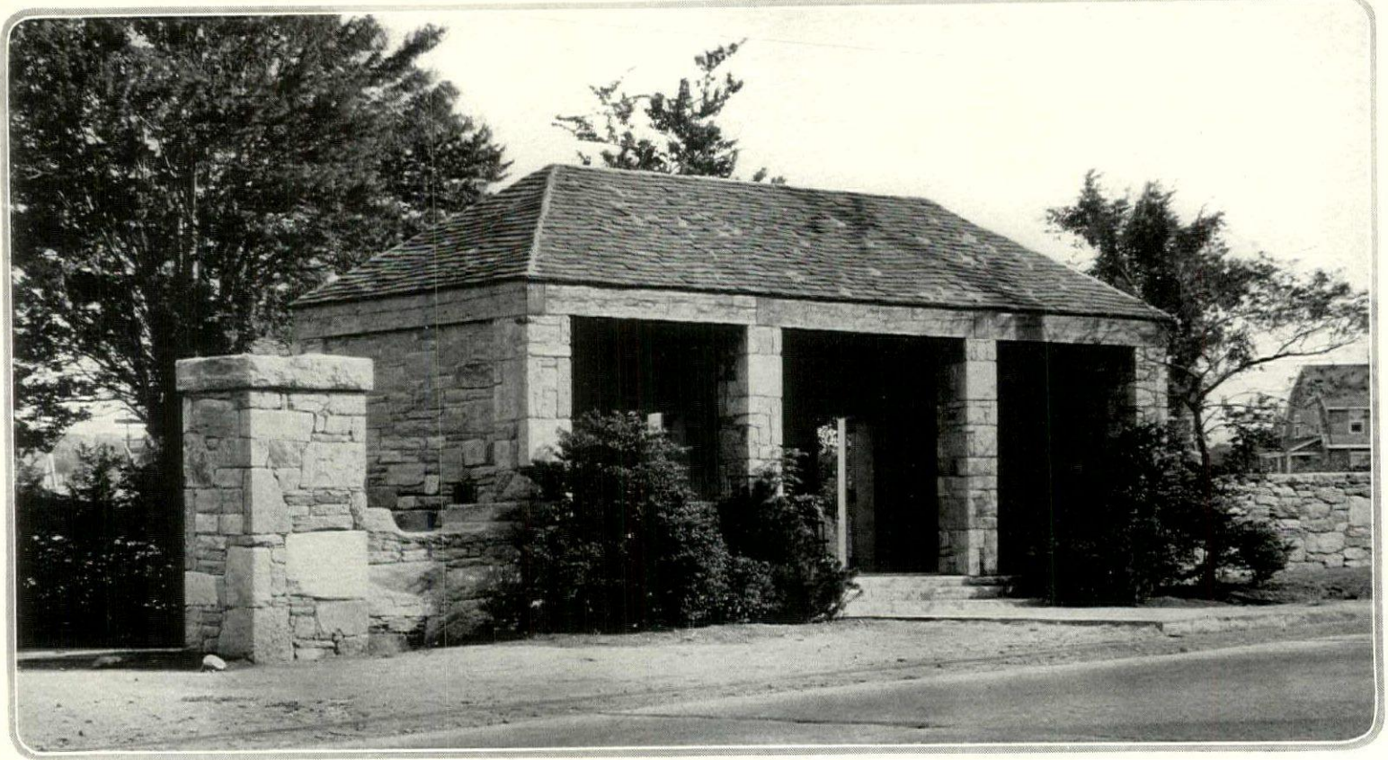
This trolley passenger shelter, at the Condé Nast Plant at Greenwich, Ct., is part of extensive developments being made by the publisher of House & Garden
