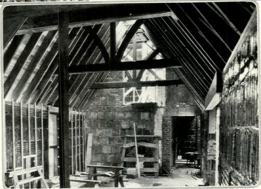
(Above) The second floor joists are being laid over the dining room. The photograph at the top of page 115 shows this section of the house after the roof sheathing has been laid
