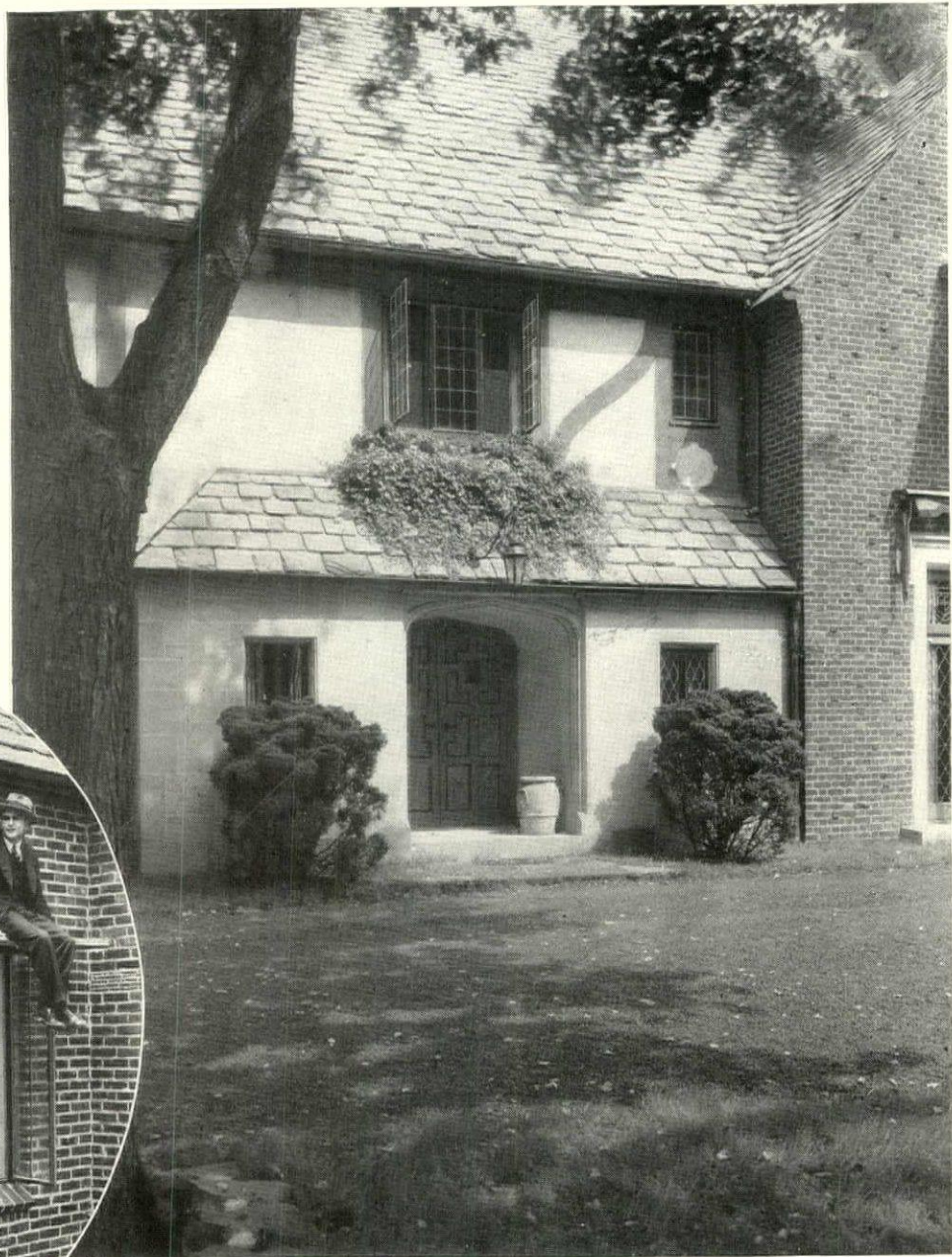
Residence Plainfield, N. J. Patterson-Wilcox Architects
