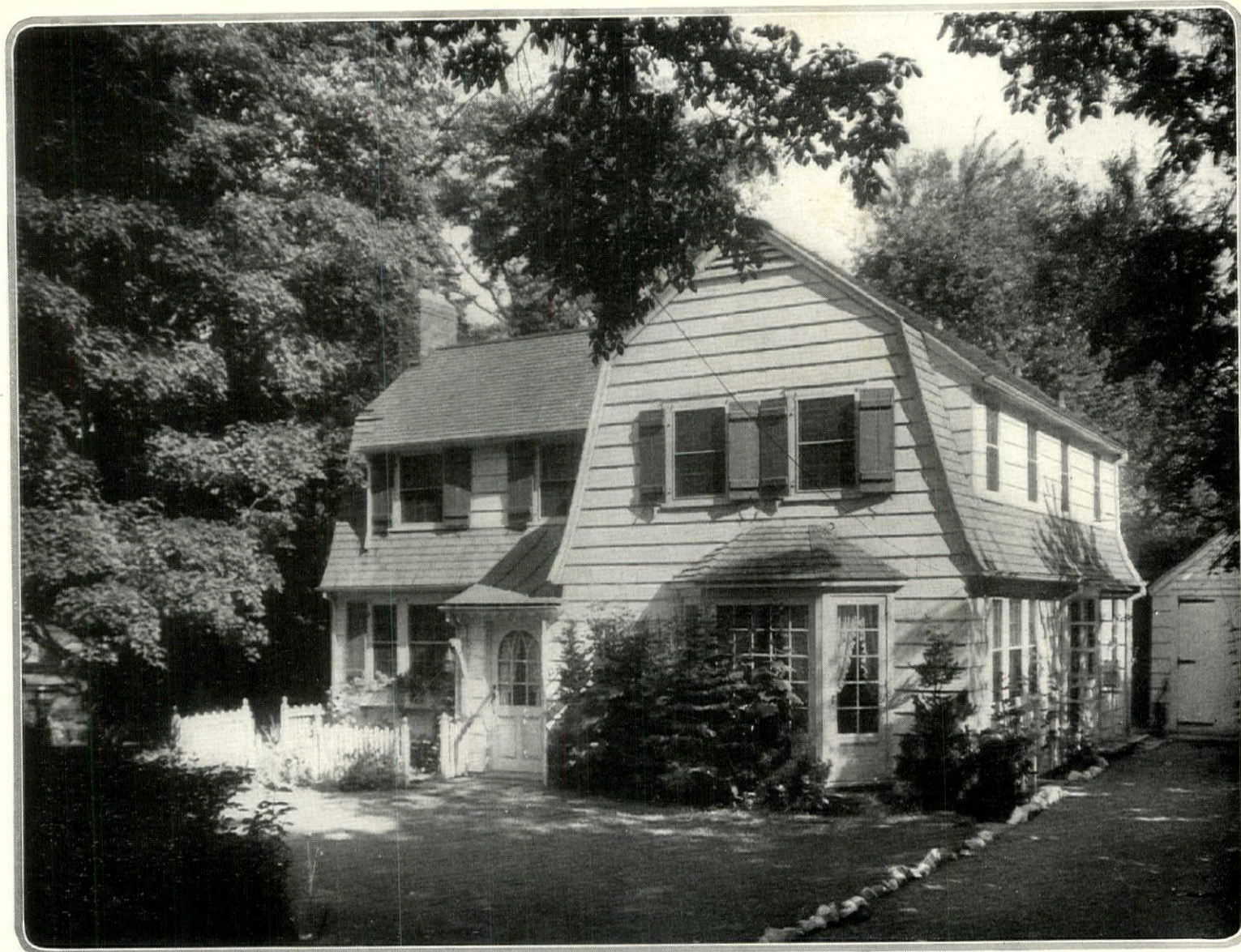
Although not a small house, the low-hanging eaves, the gambrel roof and the shingled exterior all combine to give this well designed residence a "cottage" atmosphere. A gambrel roof is not only picturesque but practical in that it allows maximum interior space on the second floor. The home of D. W. White, Douglas Manor, L. I. Alfred Scheffer, architect
