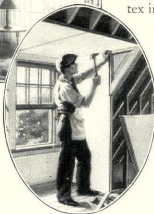
Anyone who can use a saw and hammer can finish off an attic room with Celotex in a few hours. You simply nail the broad, light boards to the studding and rafters. Celotex converts your old attic into a comfortable, livable room. Its golden-tan color and rough-textured surface make an attractive wall finish . . . or you can decorate it in many ways.
