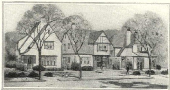
Sketch of a group of homes at Mt. Vernon, N. Y., built by L. Paulsen. A. J. Rogers, Architect.
