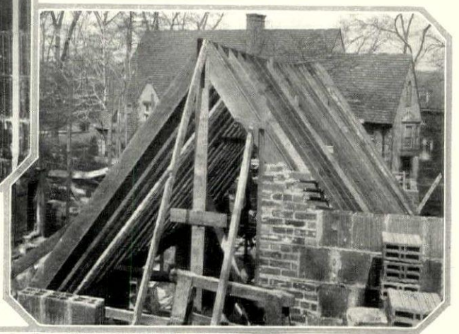
An aperture for a bay window. The lower portion of the opening is to be filled with brick and half-timber
