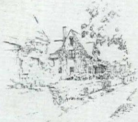
In Kohler Village The visitor to this beautiful "town-planned" community asks no further proof of the excellence of Kohler products —plumbing fixtures and private electric plants
