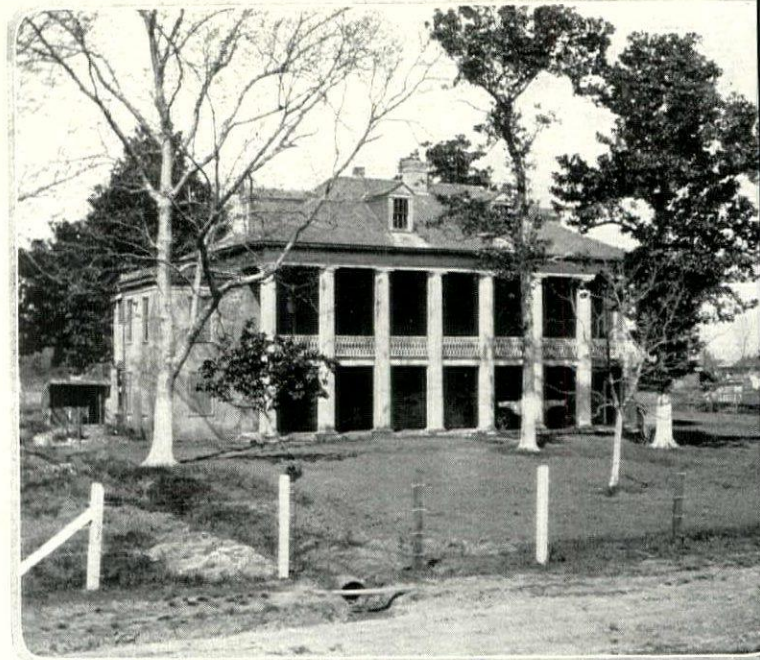
Another plantation home with two-story columns supporting a hipped roof. The columns are only across the front façade and support a second-story porch
