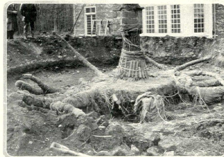
Showing how the roots of an Elm are spread out in the hole. The burlap wrapping is carefully unwound and the soil washed around the roots so that no fatal air pockets are formed.
