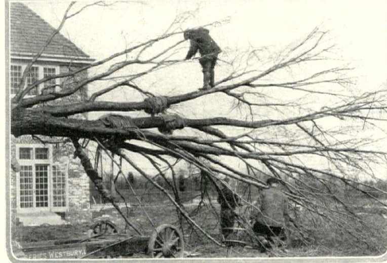
These two views show the wrapping of the roots and branches. From this position the tree is lifted and set in the hole with block and tackle. Broken limbs are cut off.
