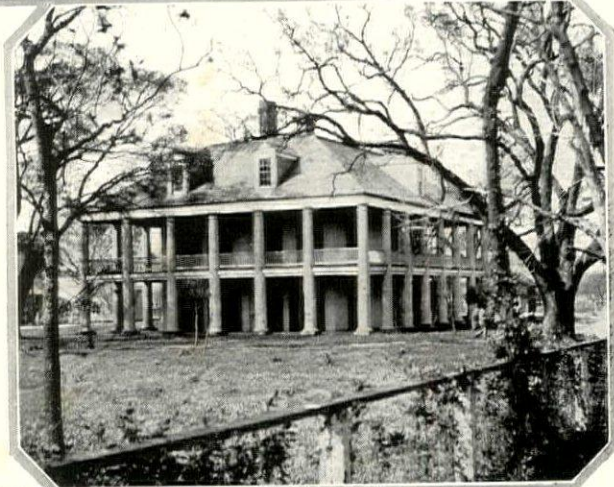
The hipped roof supported by two story columns makes some Southern homes appear low in height. Dormers break the barren appearance of the roof
