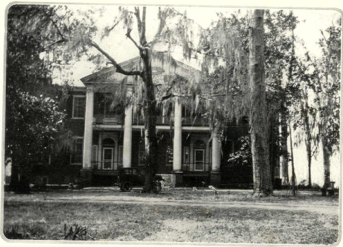
This typical plantation house near Natchez, Miss. has two-story Classic columns leading to a pediment. The second story porch also is found on many Southern plantation homes
