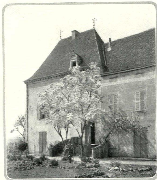
This steep roof is covered with small and somewhat irregularly-shaped mellow orange-red tiles which give a soft wavy texture. Château at Fleurville, Saône et Loire
