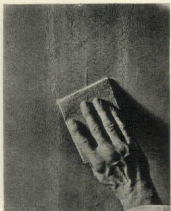
D. The cement is sandpapered, leaving a smooth surface for your decoration. U. S. Gypsum
