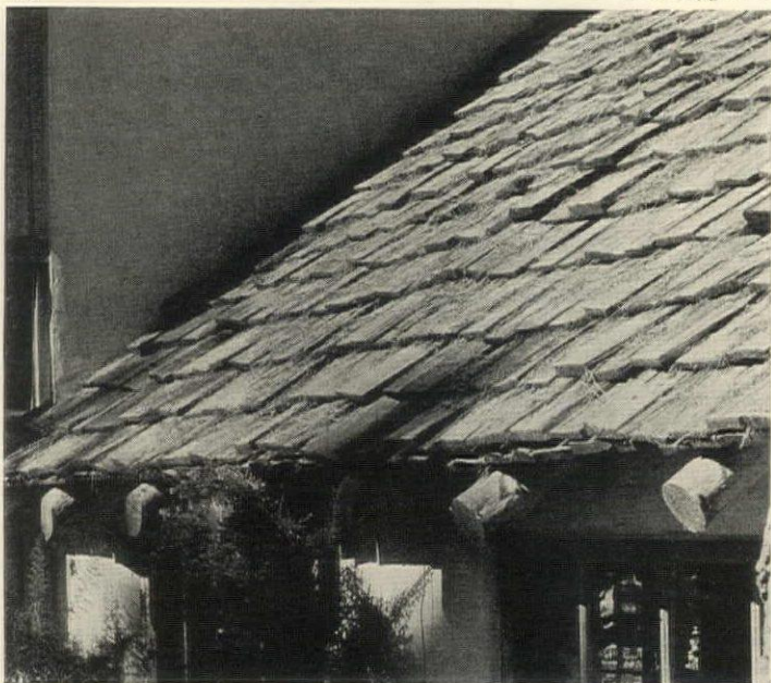
Thick, hand-split redwood shakes possess all the character of a traditional material used in traditional fashion. They are particularly suitable for a country home, such as this at Del Monte, Cal.
