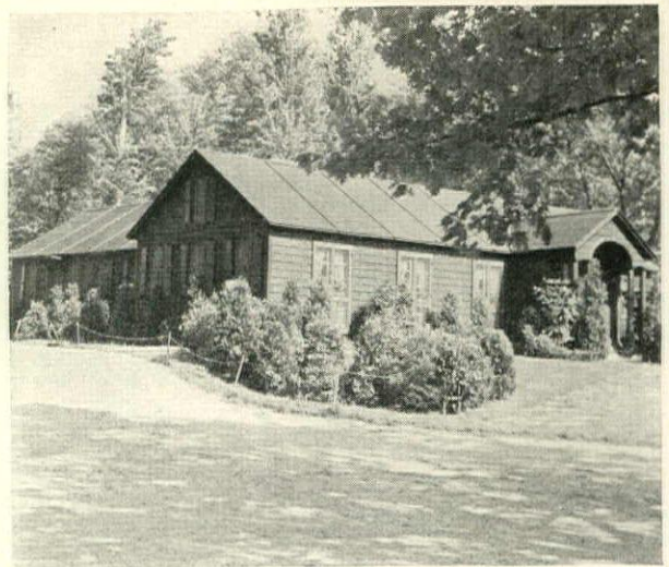
ALL the houses illustrated on this page are built of prefabricated sections manufactured by the Hodgson Co. Principles of construction originally applied to camps and sheds 40 years ago are now extended to the building of completely fitted houses
