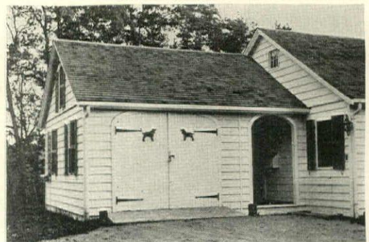
THE price of a completed house can be estimated in advance, by adding up the prices of the units from which it is built. Allowance must then be made for the cost of foundations, heating and plumbing fixtures, and labor needed for erection
