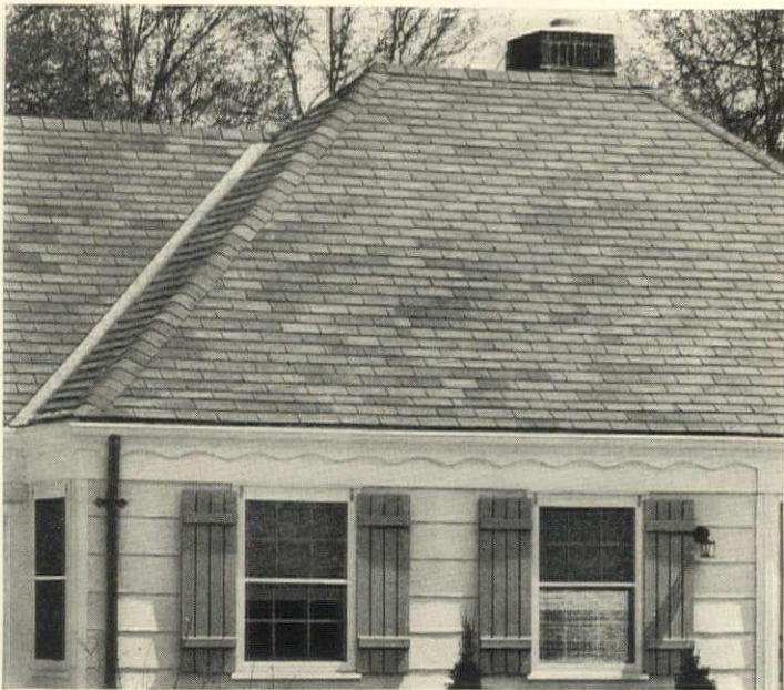
These shingles are made of mineral granules cemented with waterproof asphalt to a felt base. They are available in various types to fit either traditional or modern architecture. U. S. Gypsum
