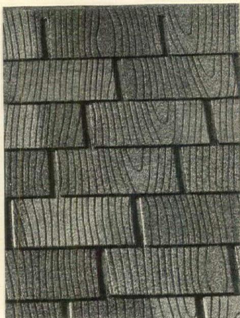
A layer of these asphalt shingles applied over a dilapidated roof will serve to improve its insulation value noticeably. Ruberoid
