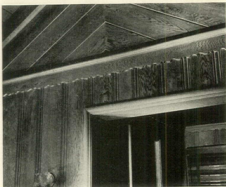
To preserve the wood and bring out its full richness of grain, an oil finish is very satisfactory. The rose-brown color of redwood responds particularly well to such treatment. California Redwood Association
