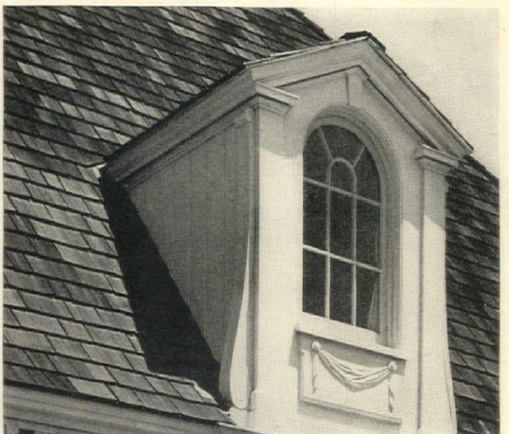
For long life and distinguished appearance good-quality sawed wood shingles are among the best materials. Exposure to the weather serves to improve their soft coloring. Van Pelt & Lind, architects
