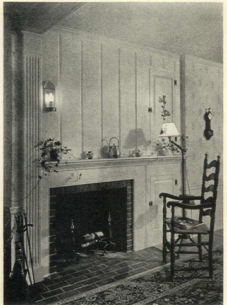
In all rooms the design of fireplace and trim should be in complete harmony. Often, as here, the mantel moulding will be a modified version of that on the cornice. D. J. Abrahams, architect
