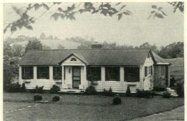
CEDAR is used for roof and walls. The roof is green, the walls stained or painted white according to taste. There is a good choice of different door and window designs, porches, etc. And the house may be ready for occupation inside of three weeks
