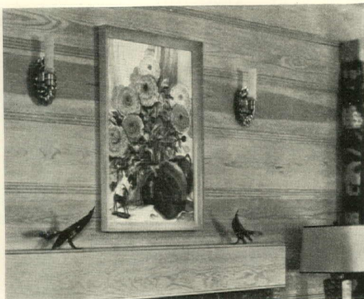
Pine paneling laid horizontally gives a spacious and sturdy effect, especially when wide boards and shallow beading are used. It is an excellent soft-toned background for works of art. Arkansas Soft Pine
