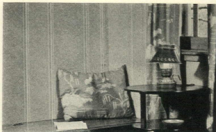
Wood fiber board is now made to simulate random-width wood paneling. It has good sound absorption, fine insulation value, and beadings which disguise joints between the boards. Wood Conversion Co.
