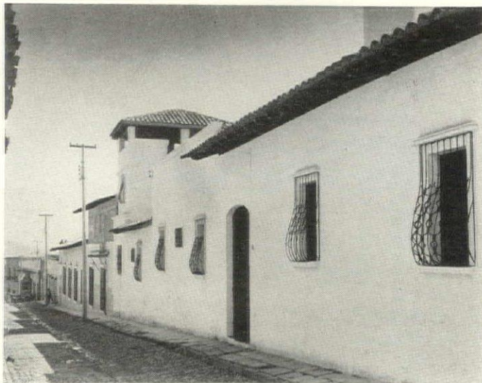
The exterior of Casa Mañana was remodeled from several little whitewashed adobe houses along the street in Cuernavaca, Mexico. A Spanish mirador was built above the farther bedroom wing
