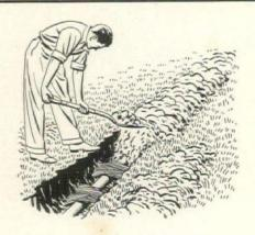
Fill in the trench after all tile has been laid and the joints covered. Don't loosen the tile by carelessly throwing in the soil. Don't pack the soil down but allow it to settle naturally. Put all of the soil back in the trench.
