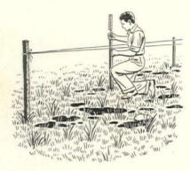
Mark proper grade on each stake. If you have the twine 2' above ground at first stake and it is in lowest part of wet area then at second stake put mark 2" below the line. If next stake is 20' away drop the line 4" and so on.
