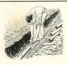
Lay 4" agricultural tile in the trench using a handful of soil on either side to keep it in position. Do not allow any space between the tiles. Be sure to check the trench to make sure the bottom is firm and the pitch okay.
