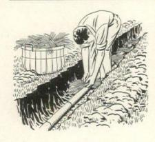
Cover joints in tile with a handful of hay. These cracks should never be cemented, as through them the water enters the tile to be drained off. Hay keeps the loose soil from washing into the tile before the earth has settled.
