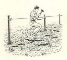
Place stakes every 10′ along the route after location of trench is laid out. Route should be where pitch is or can be made at least 20″ to every 100′. Set these stakes back 2′ from spot to be dug to facilitate digging the trench.
