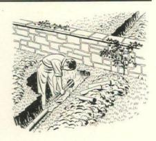
When passing under a wall, don't make the trench up to the wall itself for you are apt to disturb the foundation and cause the wall to settle. Dig up to within 2' of wall on either side and cut under it with a post hole digger.
