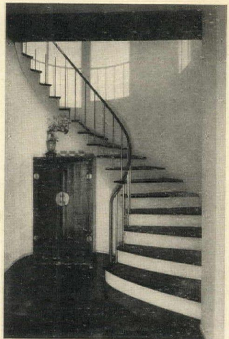
A curve of chromium posts and wooden rail
