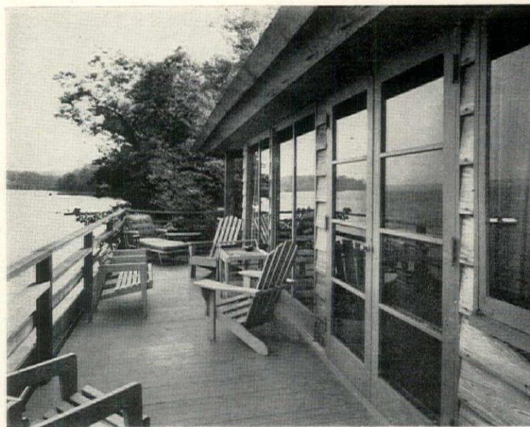
A DECK OVER THE WATER opens from the big, second-floor living room, overhangs a stone-flagged walkway below. Wide eaves offer partial shelter. Sturdy furniture can be left out in any weather. This side of house is nearly continuous glass doors and windows.
