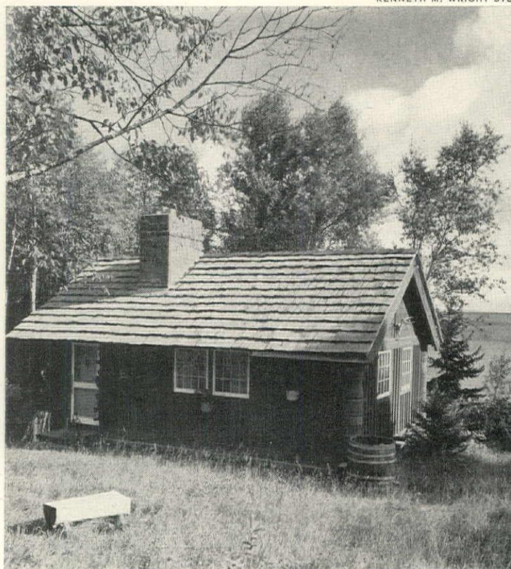
STEEPLY PITCHED ROOF suits northern landscape, is made of hand-riven cedar shakes. As in peasant cottages, the massive chimney is the heart of the house.
