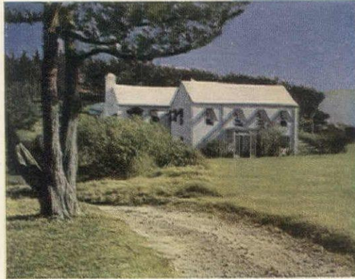
THIS OLD HOUSE in Tucker's Town illustrates the charm of Bermuda's typical architectural features: wings, gables, shutters and whitewashed stone roofs.
