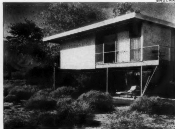
A PATIO is tucked under the living room. The thin metal columns help support the upper story, while the diagonal one braces the balcony.
