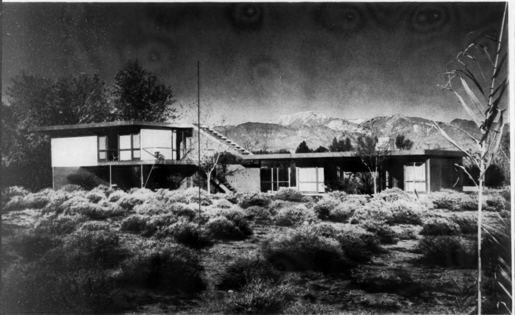
RIGHT OF THE RED LINE IS THE NEW PART OF THE HOUSE: TWO BEDROOMS, TERRACE AND CAR SHELTER
