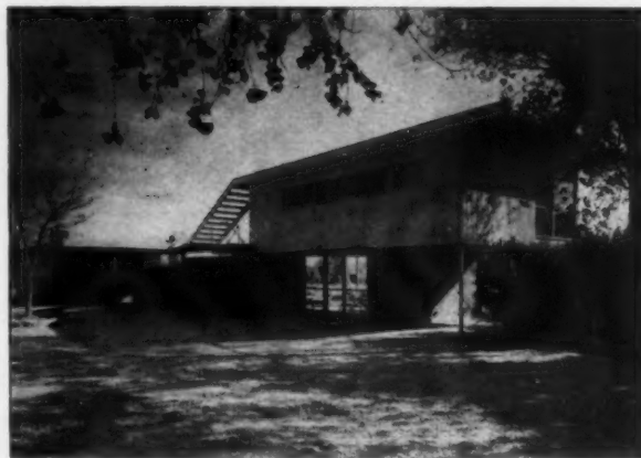
TWO SHELTERS keep the hot sun off guests' cars: one under the old house (foreground), another formed by overhang of new wing.
