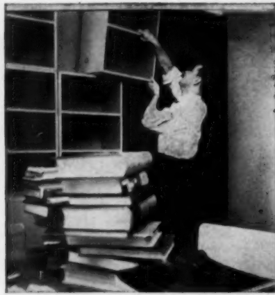
ASSEMBLY ON THE SPOT was managed by Mr. Landman, who had only to bolt the units together to create storage wall.
