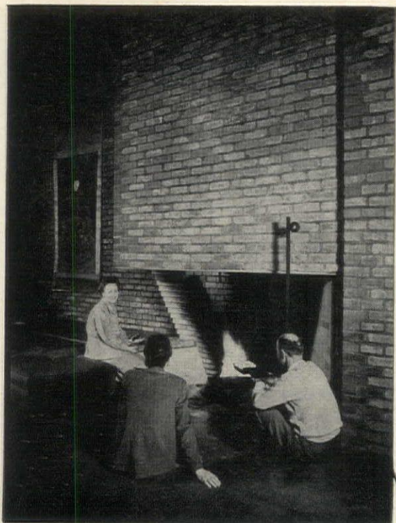
LIVING ROOM CHIMNEY of old rosy bricks interspersed with hard-fired purplish ones. This part of the core of the house shares the chimney with the adjoining kitchen.
