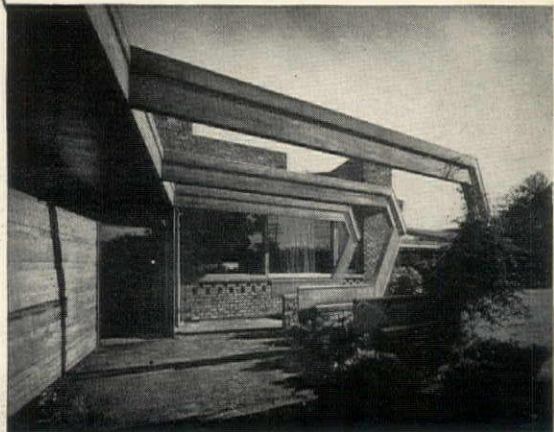
KITCHEN WINDOW VIEW is of a modern arbor, which repeats the materials and colors of the interior of the kitchen.
