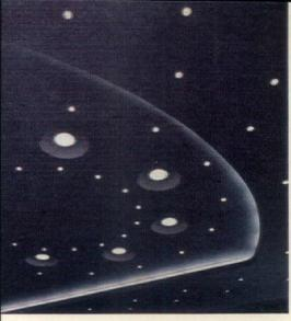
CEILING LIGHTS in Security Council Chamber give diffused illumination from large, recessed domes, varied by small, direct spotlights arranged in a circular design.
