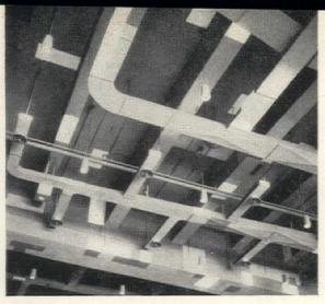
PARTLY EXPOSED CEILING saves plastering, forms network of unusual design. Air conditioning ducts, pipes, light conduits are painted a harmonious gray. Ceiling detail, Economic and Social Council Chamber.
