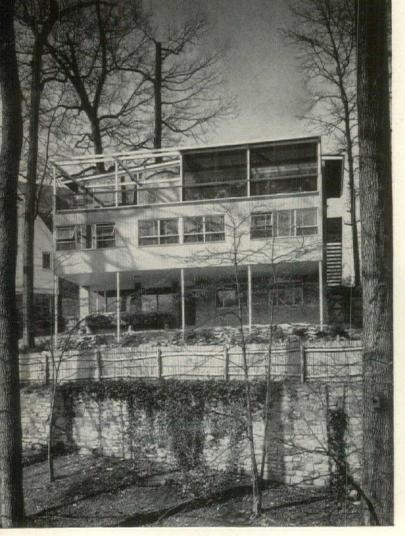
You enter the ground floor from the back garden, where the children have a fenced play area. Because site slopes so steeply, the center (bedroom) floor rests on a series of steel columns.
