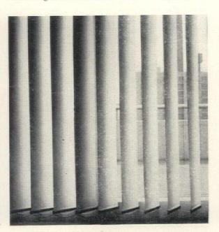
VERTICAL LOUVERS of fireproofed, opaque window shade material control light along window walls of the South Lounge. A central pull cord permits panels to be arranged in overlapping screen or open to sun.
