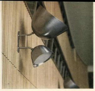
LIGHTING FIXTURES in Trusteeship Council Chamber are set in wall of ashwood slats backed by Fiberglas matting to absorb sound. Larger unit throws light on unusual pattern of ceiling shown on the right.
