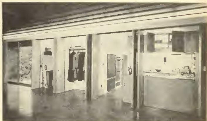
FOLDING DOORS OPEN KITCHEN TO LIVING ROOM
