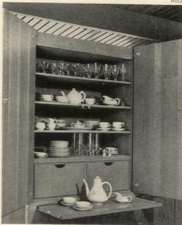
▲ Party cabinet built into family room is finished with ash-grain plastic laminate, includes deep drawers for linens and a pull-out serving counter.
