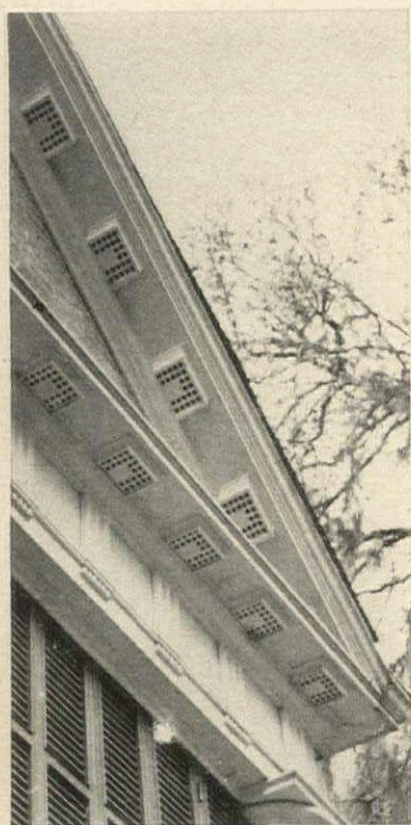
PERFORATED WOOD BLOCKS ORNAMENT THE UNDEREAVES LIKE SQUARE HONEYCOMBS
