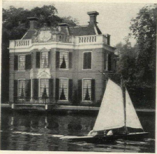
On the bank of the Vecht River: a stately house of brick (a favorite Dutch building material) with a typically steep hip roof and four square-capped chimneys. Baroque cornices over center windows and a lavish baroque medallion set into a roof-line balustrade dress up façade exposed to river traffic.
