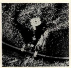
7. Types of head fittings vary according to system purchased. Lawn heads are sunk flush with sod surface, are all but invisible.
