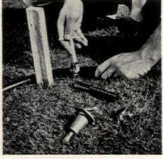
5. Once pipe lines are laid out on the surface, taps are quickly made at required locations to receive branch T's of sprinkler heads.
