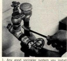
1. Any good sprinkler system you install yourself begins with the proper valve assembly that is attached at the source of supply.
