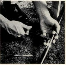
3. All pipe lines should be measured and cut, and all fittings, metal or plastic, inserted according to manufacturer's rules.
