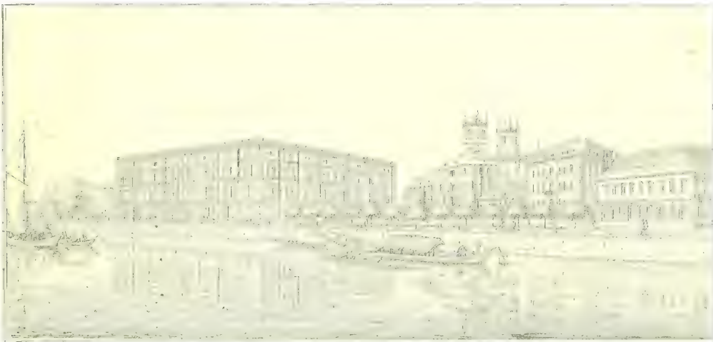
In Berlin, Schinkel's Bauakademie, left, and Neo-Gothic Friedrich-Werder Church, right
