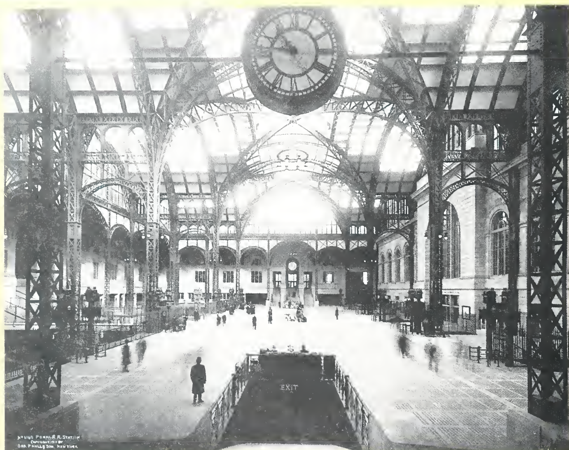
Pennsylvania Station, McKim, Mead & White, 1904–1910
