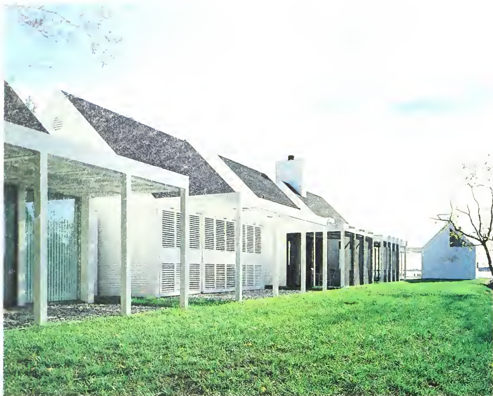
With the shutters raised, preceding pages , the living room is shaded from the sun. Pool house is a fifth and separate “Monopoly” structure. Right : The long axis of the house parallels the allée and road, the latter extended by a long pier. From the water is seen only a small house and its outbuilding. Above : At far left, the master suite pavilion; at far right, the pool house.
