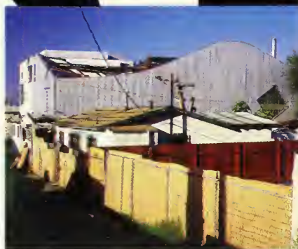
Brian Murphy's house for Dennis Hopper in Venice, California. Page 178. Photograph by Tim Street-Parter.
