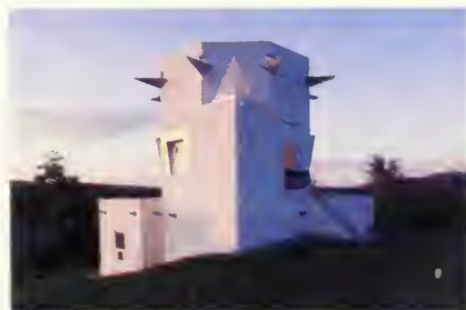
At rear: pointed skylight, kitchen entrance
