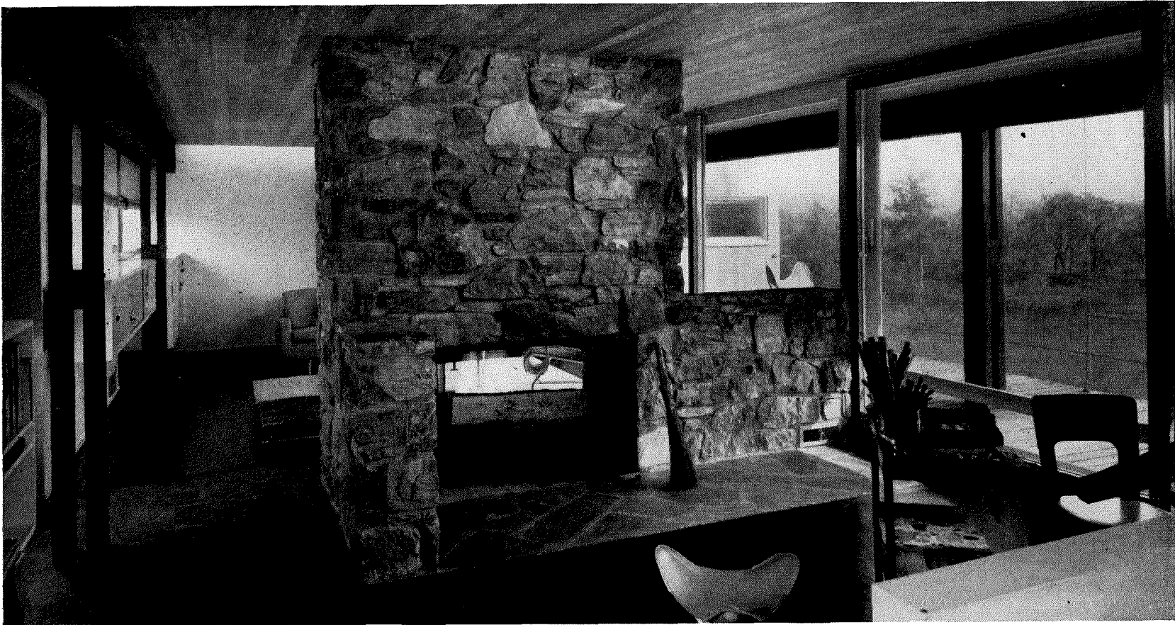
Upper floor is divided into living area and studio by free-standing, two-way fireplace. Note double posts on both sides of structure. They hold bolted steel girders between them. Clerestories are at left.
