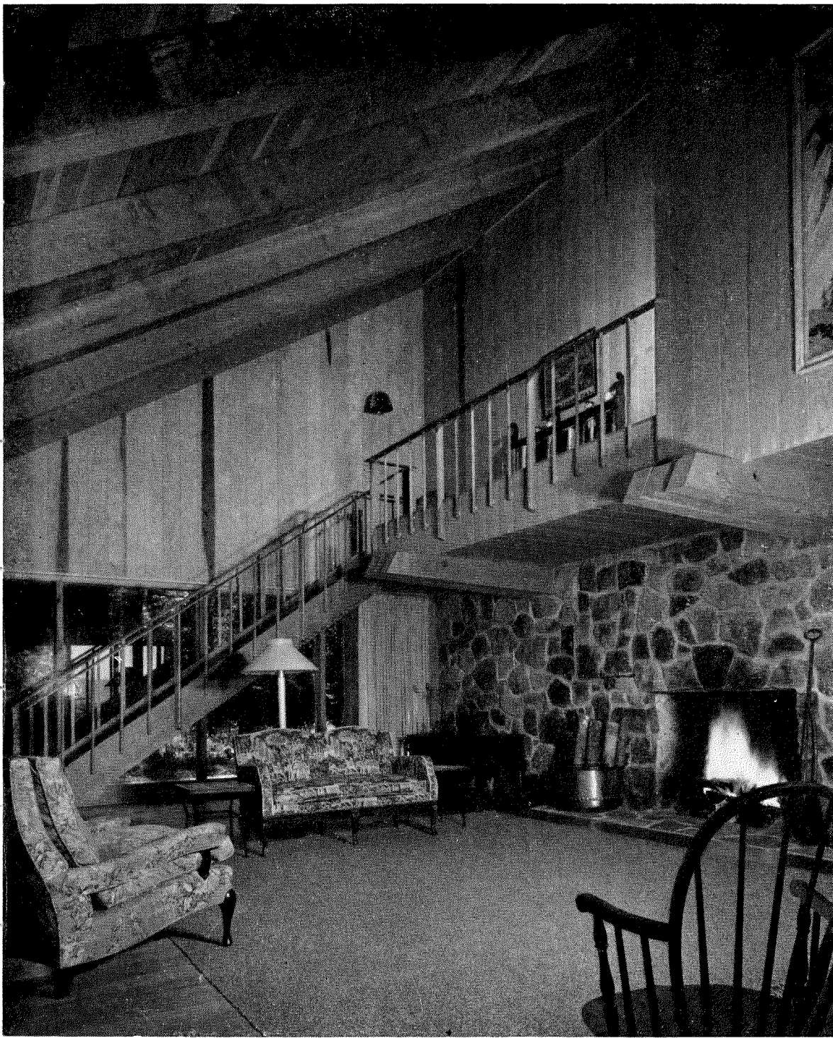
INSIDE THE LODGE (see above and right) this same structural idea is repeated: rough, flat timbers placed side by side to form cantilevered girders, supported on a massive base (the stone wall, in this case) and a crisp, neat form on top.
