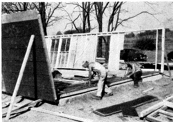
Many builders fabricate their framing and put siding on while frame is horizontal, but few tip up the entire wall of one side at a time. Everything possible is precut at Place's shop. Drawing at left shows construction details.
