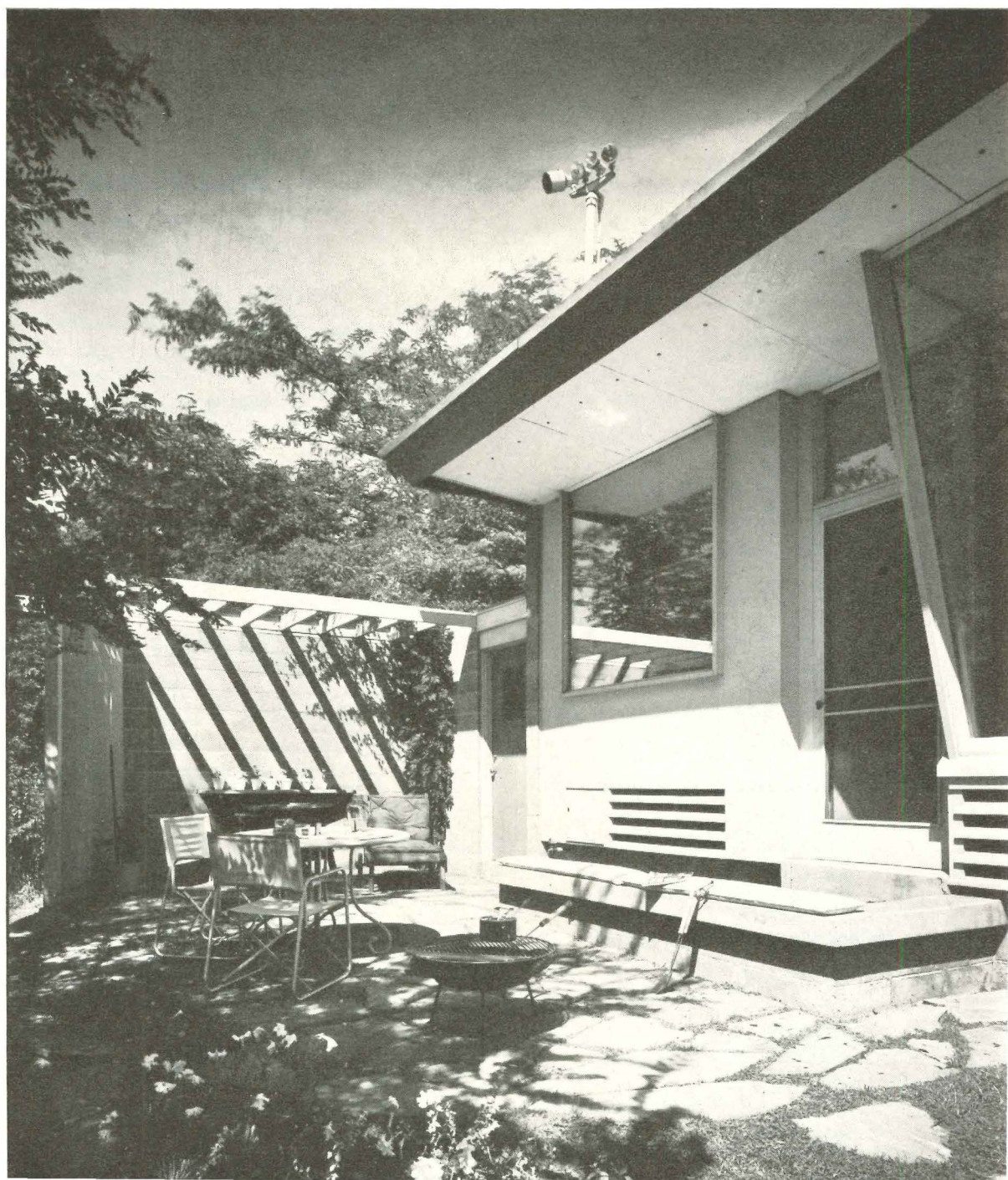
ce is shielded from low western and highway traffic by a covered block wall. Adjustable vertical s toward prevailing southwesterly can be closed to form a solar or sunbathing in the morning, and tered area for outdoor cooking and g in the early evening. Small door e louvers in wall of house opens to e a pass-through from kitchen.
