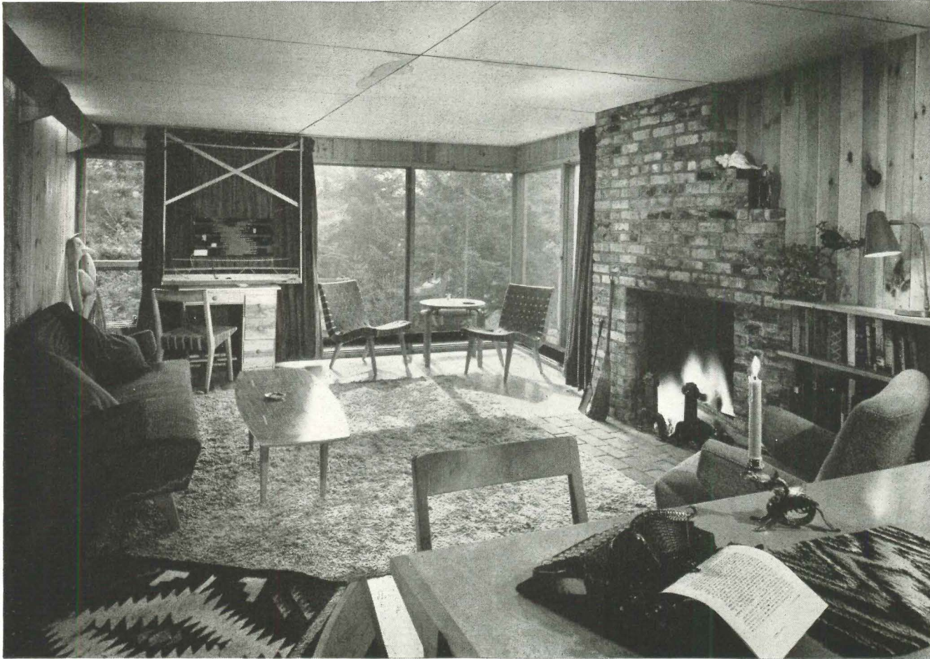
All-glass corner makes only break in 2' framing rhythm. Finned pipe in front of glass provides heat, 7' ceiling height conserves it.
