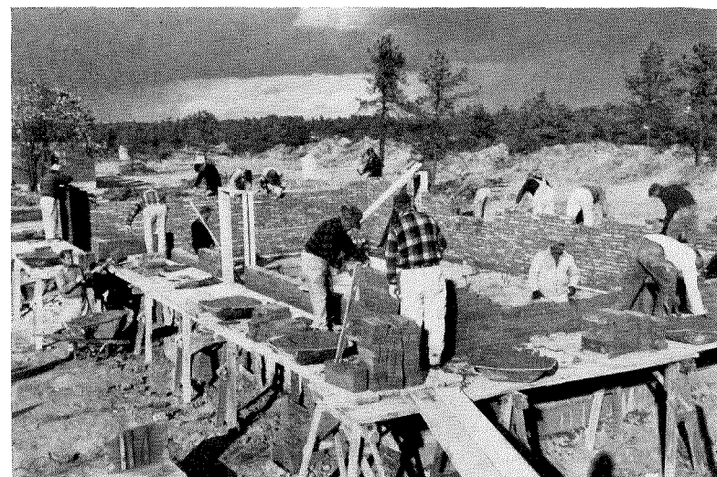
Masonry labor on each of first six houses cost $421 including block partitions. Masonry materials cost $379. Each man lays approximately 350 bricks in a seven-hour day, which is considerably less than on some jobs in the Middle West where men frequently lay as many as 500 to 700 bricks in an eight-hour day.
