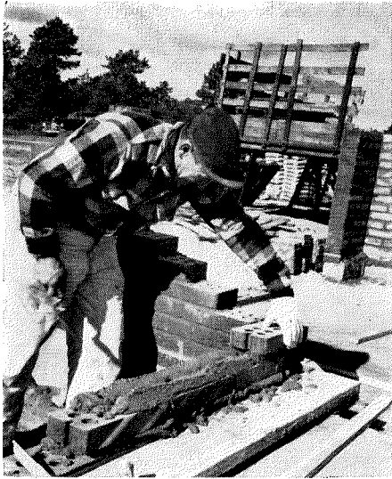
Labor unions encourage SCR bricks because through their use more bricklayers will be employed on residential jobs. Holes (as in bowling ball) make brick easy to pick up.
