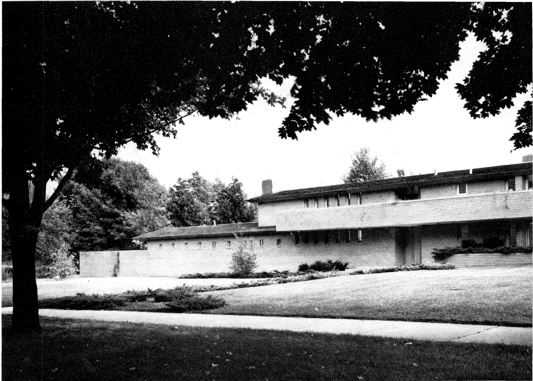
Photos: © Ezra Stoller
