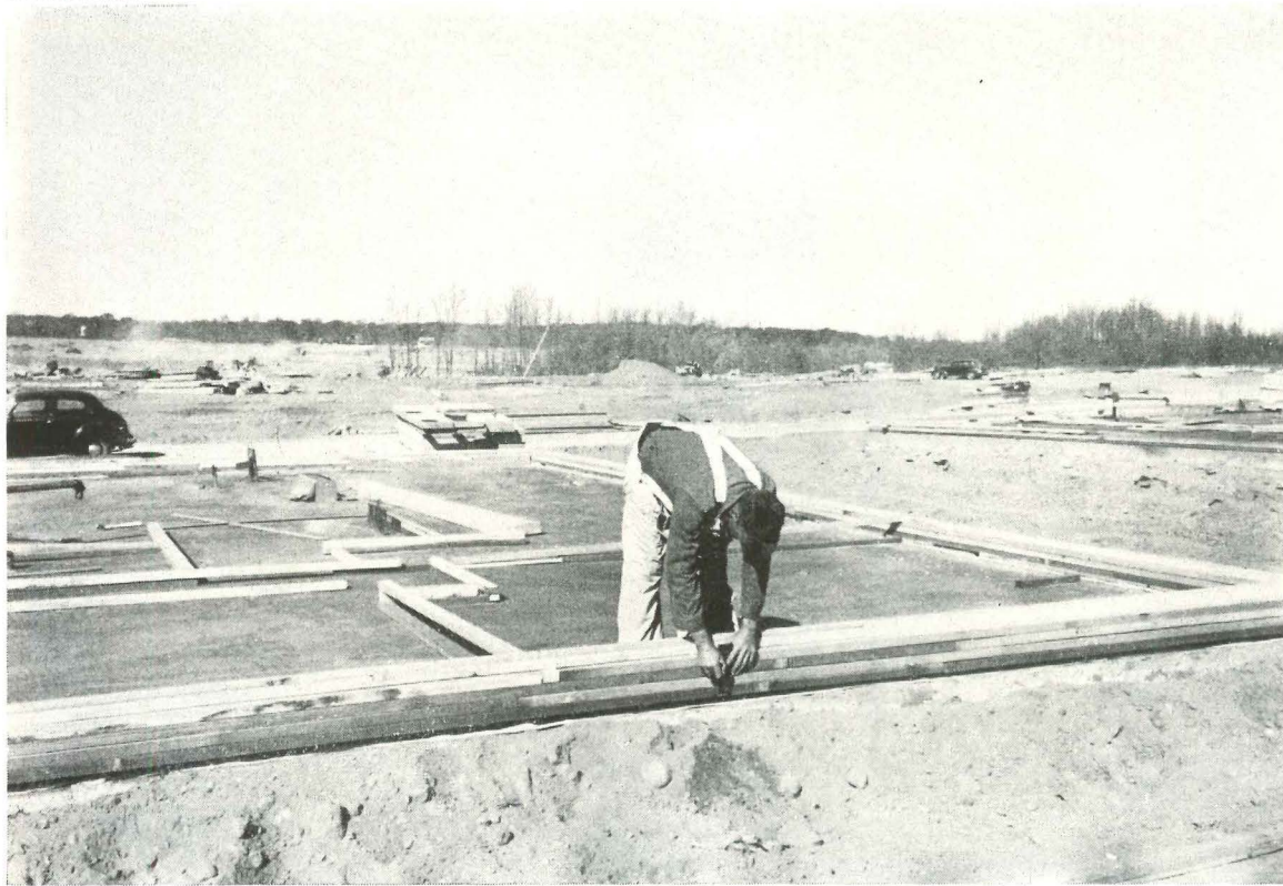
Layout man is key figure. He installs sills for exterior wall and partitions and marks position of every stud, window and door. He lays out four or five houses per day. His speed is due to fact that except for window locations, every house is approximately the same.
