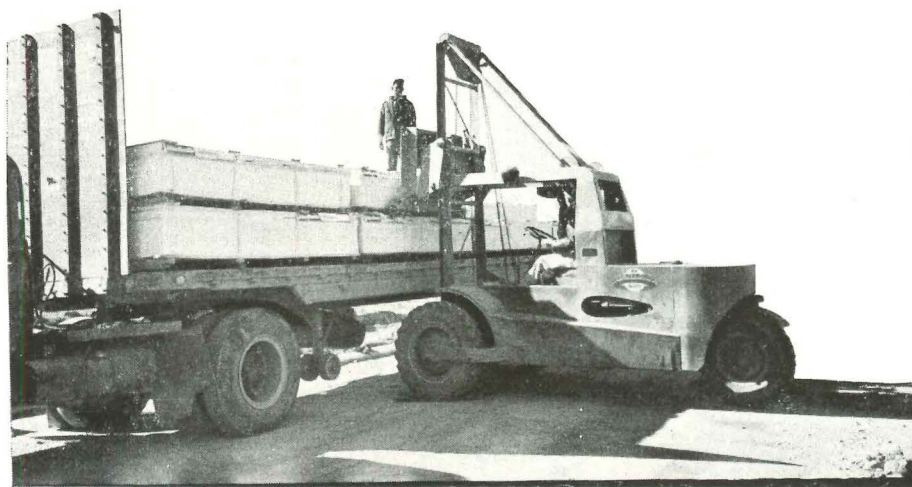
Asbestos siding , packaged with right color, is fork-lifted to each house
