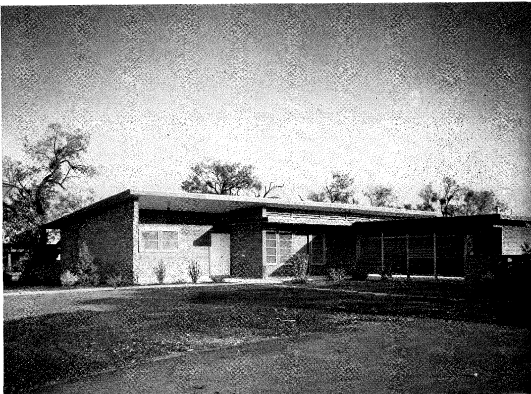
One of five demonstration models, this house has T-plan, clerestory louver vents, fence shielding carport
