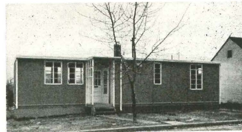
PHA TEMPORARY has painted pressed board and batten siding, casement windows, two bedrooms and an alcove usable as a third, same equipment and foundation as PHMI unit. The shell was erected in 6½ hrs.
