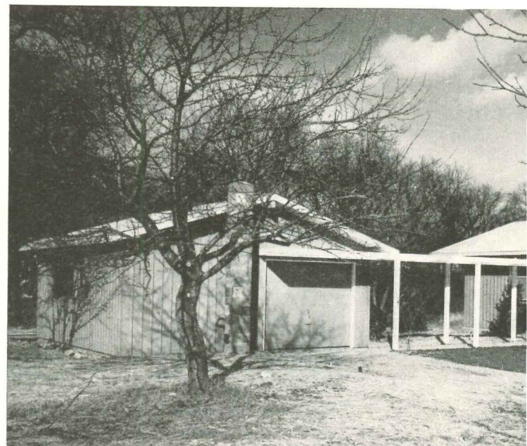
★ Link to house under low-cost translucent paneling. Garage can be reached under cover in rainy weather. Detached as it is, noise from power machinery won't keep the children awake—sales point that could be made by a sign.
