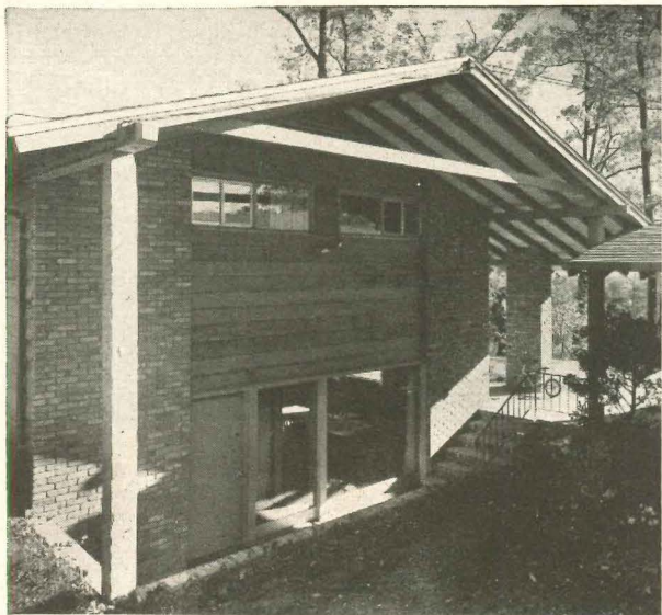
Porch , off kitchen and dining room, at south end of house, has brick-paved floor 4' below grade level. Porch is one of five outdoor living areas and is particularly suited for small children whom mother can watch through wide windows and glass doors. Top soil of sloping lawn above is laid on gravel base, thus on even the rainiest days soaks up water before it reaches porch. Crossbeam under roof would seem to obstruct view from upper windows.
