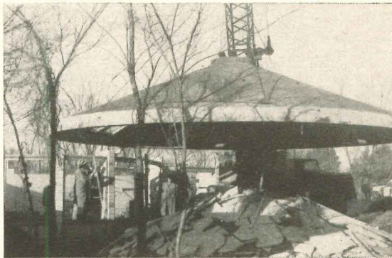
Experiment in structure includes concrete cone, poured on the ground and lifted into place (see p. 168).
