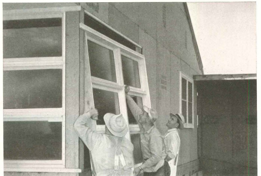
Ease of installation is shown here as men work 6-sash Flexivent group quickly into place in window opening. Groups might just as easily be assembled in shop and trucked to site.
