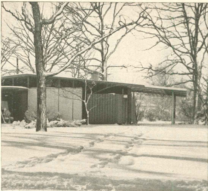
Before. Driveway of USG house by Architect Quincy Jones (see p. 112) is 60 ft. long. Boiler capacity for heating house is 90,000 Btuh.
