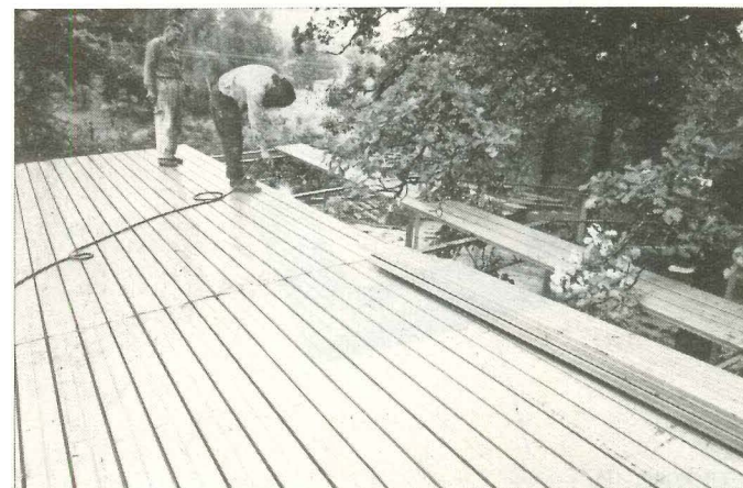
Rigid insulation, built-up roof, top decking
