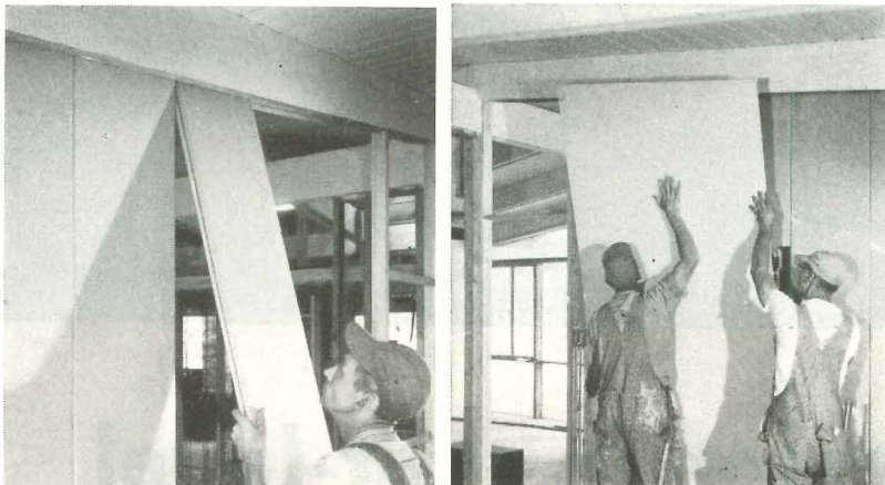
Core fits into joist . . . is faced with wall board
