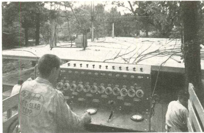
One hundred tons being lifted hydraulically
