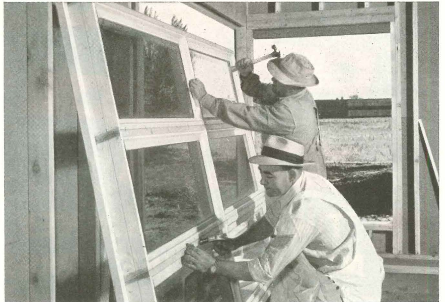
Ease of assembly is evident as workmen at the Spande 50-home Westwood Gardens project assemble 6-sash Flexivent group on the site. Units come completely packaged ready for assembly.
