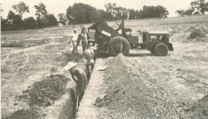
Mobile trencher can easily make 90° turn (above), speeds off to next foundation job when finished.
