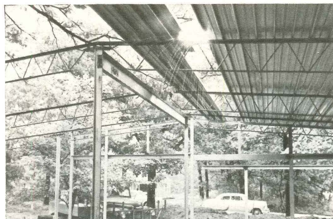
Welding replaces nails
