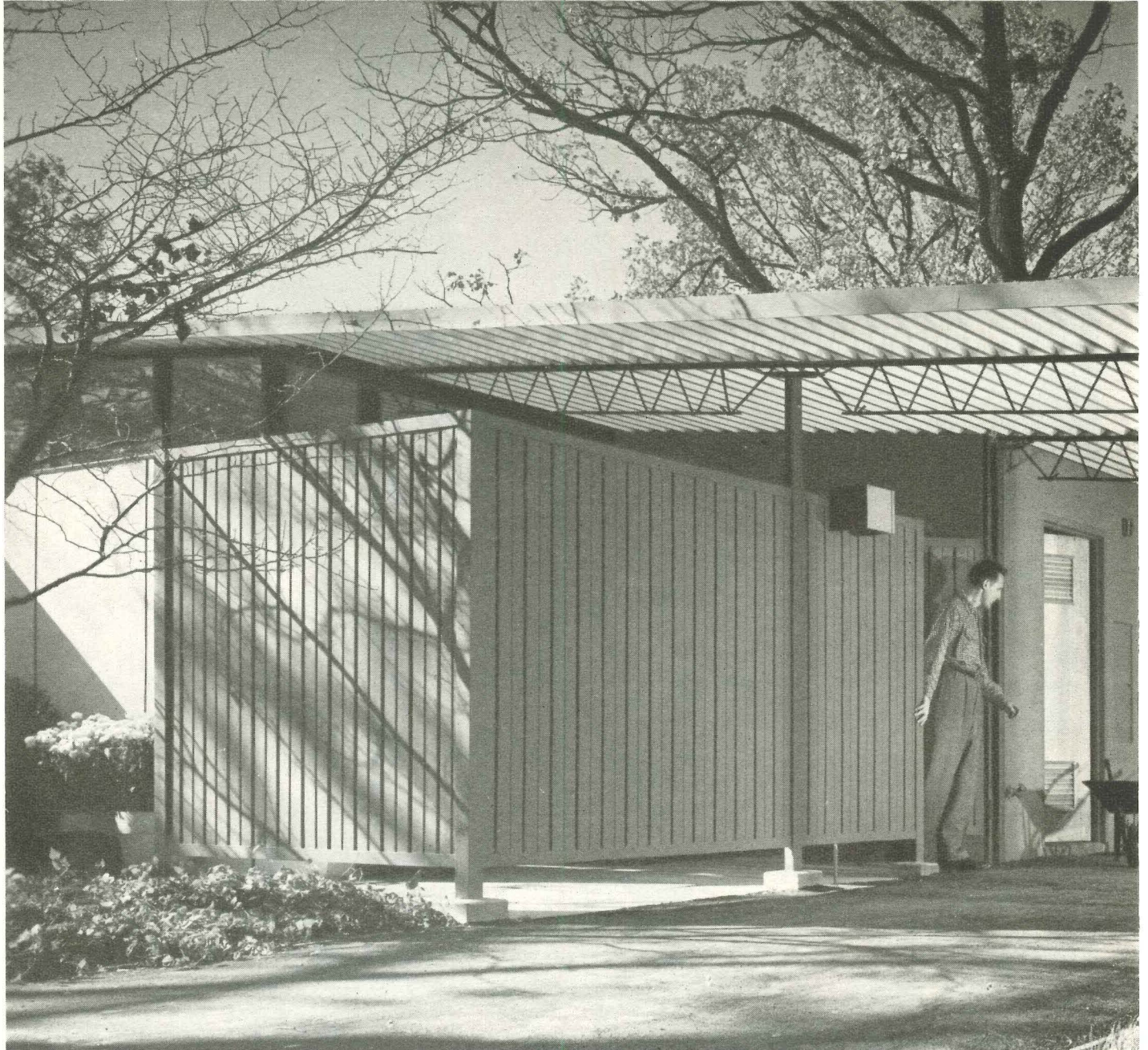
Steel predominates in the entrance area. Roof decking turns vertically for garden wall; open web beams are supported by steel T posts. Entire roof weighs only 1½ tons, requires little maintenance.
