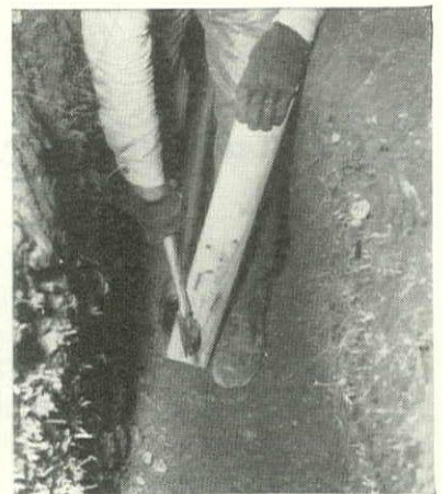
Connector is tapped onto tapered end
