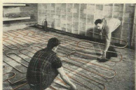
HEAT FOR THIS basement game room will be provided by 1/2" PG's embedded in concrete. For floor or ceiling installations the pre-formed Anaconda Panel Grid offers many economies.
