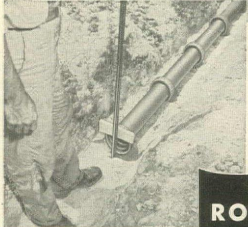
Push the pipe together . . . the joint is complete!
