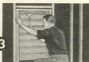
3 Ready-made attic louvers can be installed quickly by one man. Sizes for each of various-sized fans.
