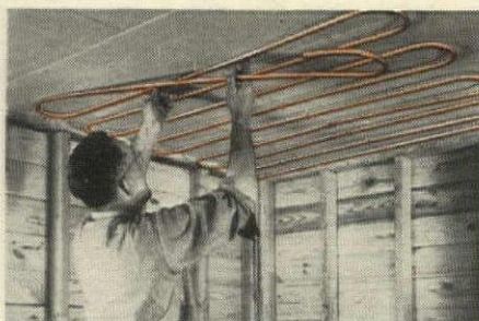
A HOOK TYPE FASTENER offers another easy, quick installation method. Fasteners are partially set in joists, PG's are positioned, and fasteners driven home.
