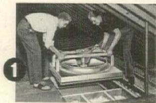
1 Fan and shutter arrive set up. Simply place fan over framed ceiling opening. Rubber cushion makes it self-sealing!
