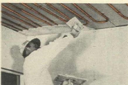
NO SAGS OR DIPS in the tube lines permits a uniform plaster thickness, which means savings in time and materials.
