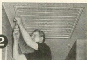
2 Complete automatic shutter unit screws to ceiling opening frame; flange forms trim. No finishing needed.
