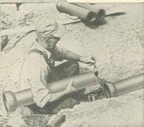
Paint the spigot joint the same way . . .
