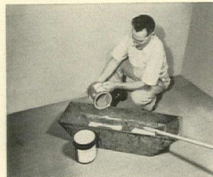
Powder and liquid are mixed here to form chemically-fusing, below-grade adhesive.
