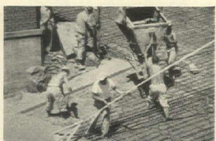
SNOW MELTING SYSTEMS are installed easier and quicker with 1/2" PG's embedded in concrete. 5411
