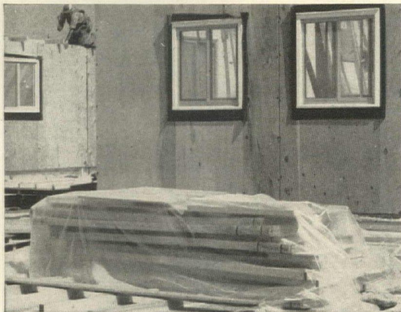
No water can reach materials or tools that are protected by VISQUEEN film
