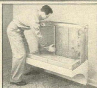
2 Hearth & firebox are formed of interlocking ceramic sections.
