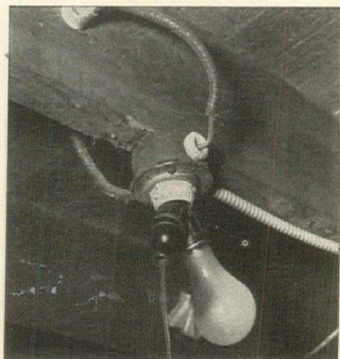
Personal selling put over Kansas City rewiring drive.
