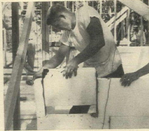
STYROFOAM IS SAWED OR CUT WITH A KNIFE, WEDGED INTO PLACE WITH WATERPROOFING AND GIVEN A 1" COAT OF SPRAYED CEMENT
