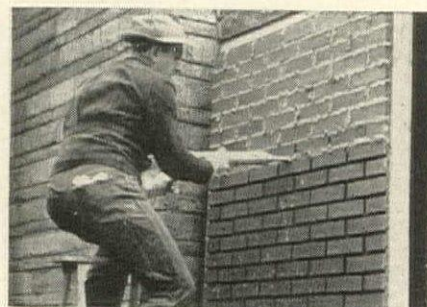
Calking gun fills joints fast, but requires tooling for finished appearance.
