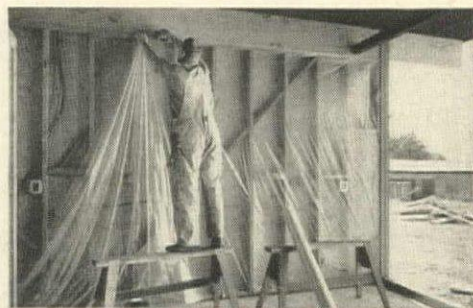
VISQUEEN film locks moisture out of studwall, prevents damage to insulation, paint peeling, rot.
