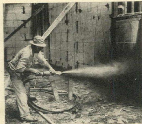
STYROFOAM IS SAWED OR CUT WITH A KNIFE, WEDGED INTO PLACE WITH WATERPROOFING AND GIVEN A 1" COAT OF SPRAYED CEMENT
