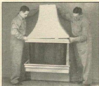
4 Fireplace hood sets on hood support channel—fits tight to wall.
