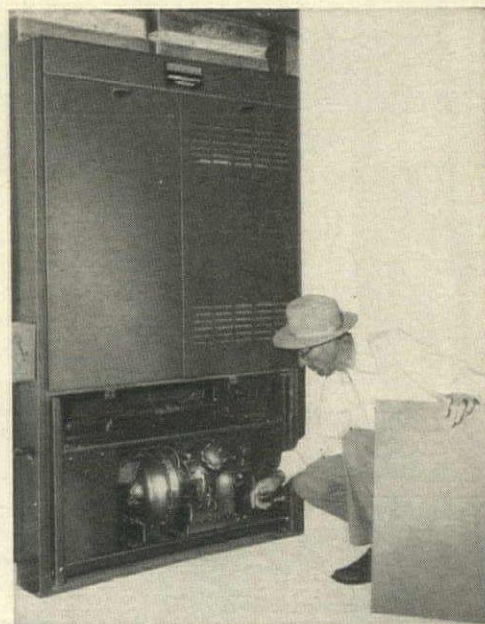
Builder Pooley likes the optional feature of Worthington's Year-Round Air Conditioner. Cooling section can be added at any time—it rolls into cabinet like a drawer.
