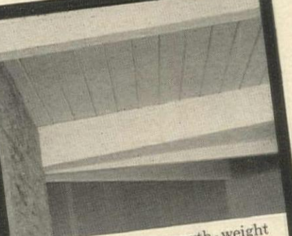
Dryness, great strength-weight ratio makes hemlock ideal for exposed plank and beam ceilings.
