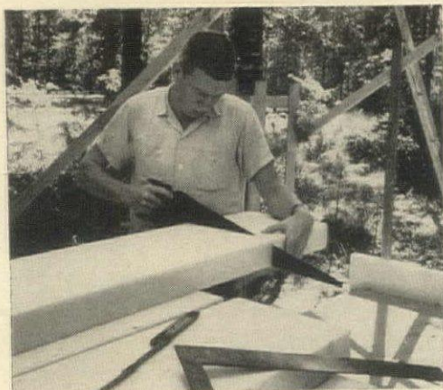
STYROFOAM IS SAWED OR CUT WITH A KNIFE, WEDGED INTO PLACE WITH WATERPROOFING AND GIVEN A 1" COAT OF SPRAYED CEMENT
