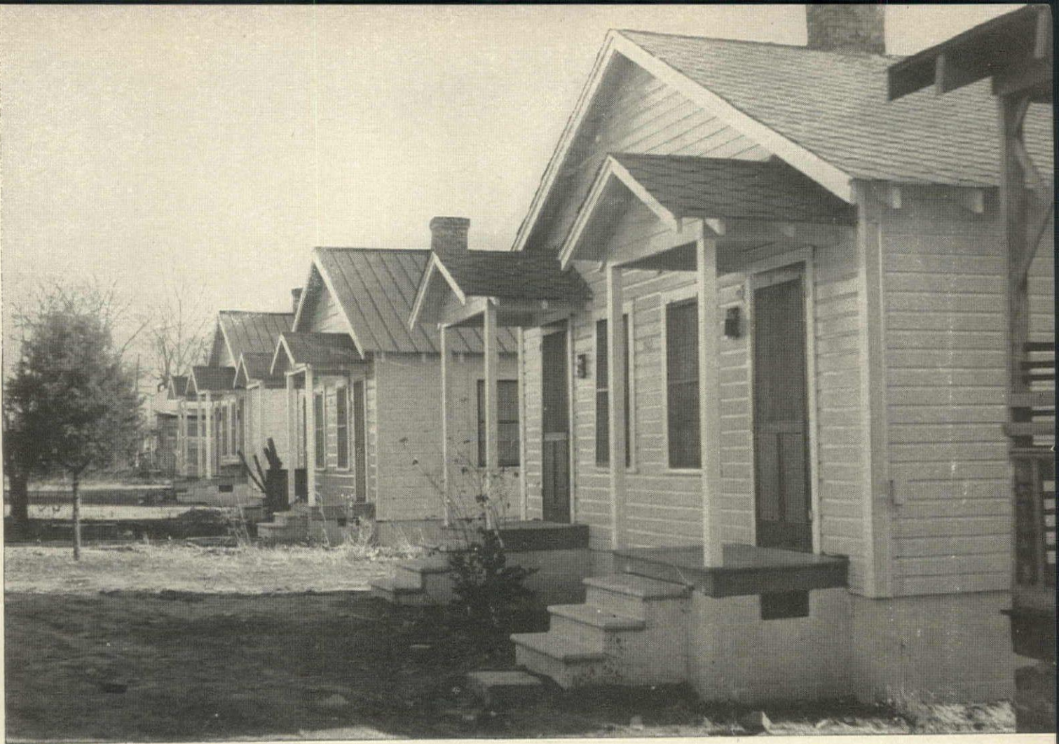
New siding, roofing, porches, steps, paint jobs, etc. turned dreary shacks (opposite) into rows of neat bungalows (above)
