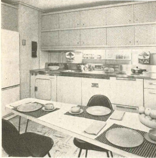
Sliding kitchen cabinet doors are hung from wall over built-in kitchen appliances, work surface.
