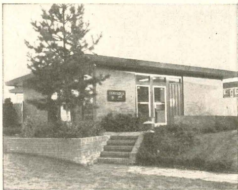
Sales office (above) is located to the immediate left of model houses shown in center spread. An important part of Sampson-Miller's merchandising plan, sales office looks substantial and professional, lends dignity to the sales force. Formerly, when sales offices were in basement of model house business was concentrated in week-end period. Now, buyers come in every day and salesmen can make better use of their time. Right: one of main entrances to the Garden City property.
