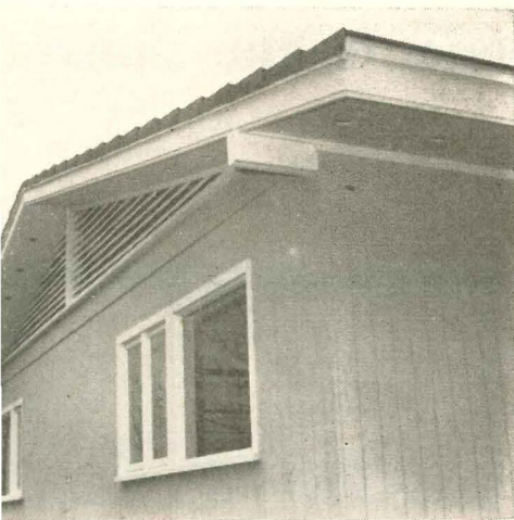
Gable end ($45) is built in lumber yard
