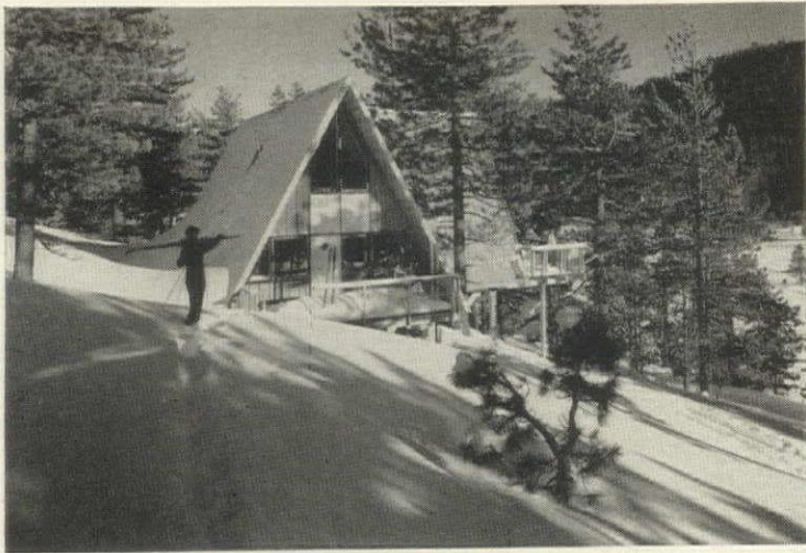
High Sierra house has steep roof designed to direct snow away from major windows, decks and entrances. Interior has 1,425 sq. ft.
