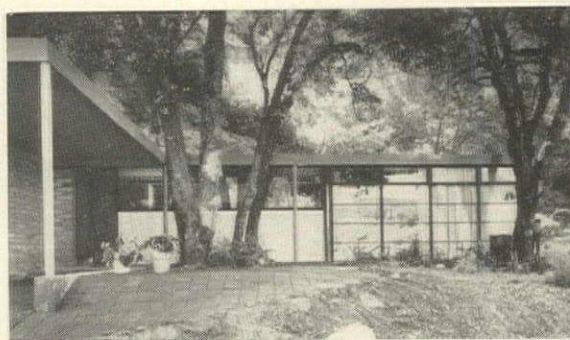
Steel frame house in Los Angeles, Calif., Pierre Koenig, designer. Basic structure consists of lally columns and light steel girders, topped with steel decking. Exterior walls are "curtains" of glass, steel and stucco.
