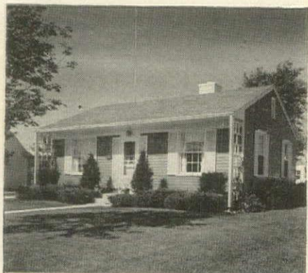
Relative inexpensiveness permits generous use of double hung wood windows with metal weatherstripping, even in the most modern homes.
