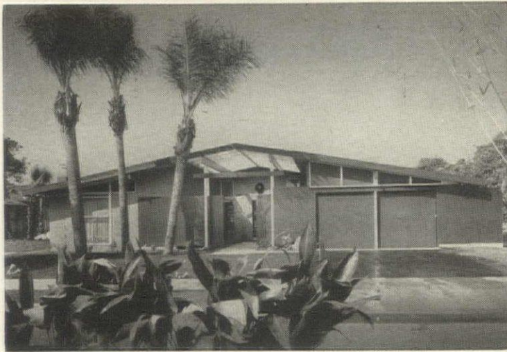
This is a "Sherwood Forest" model, reported in H&H, February, 1956. Because of double garage and long, low roof, house looks enormous.
