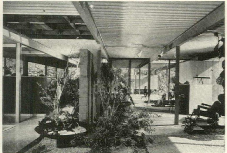
Steel frame (painted red) and metal roof decking are exposed inside house. This is Architect Quincy Jones' own house built last year.
