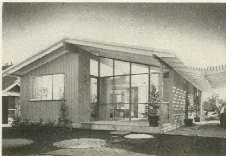
This 1953 design won praise from AIA judges for good plan, good appearance. Big windows are protected by unusually large overhang.
