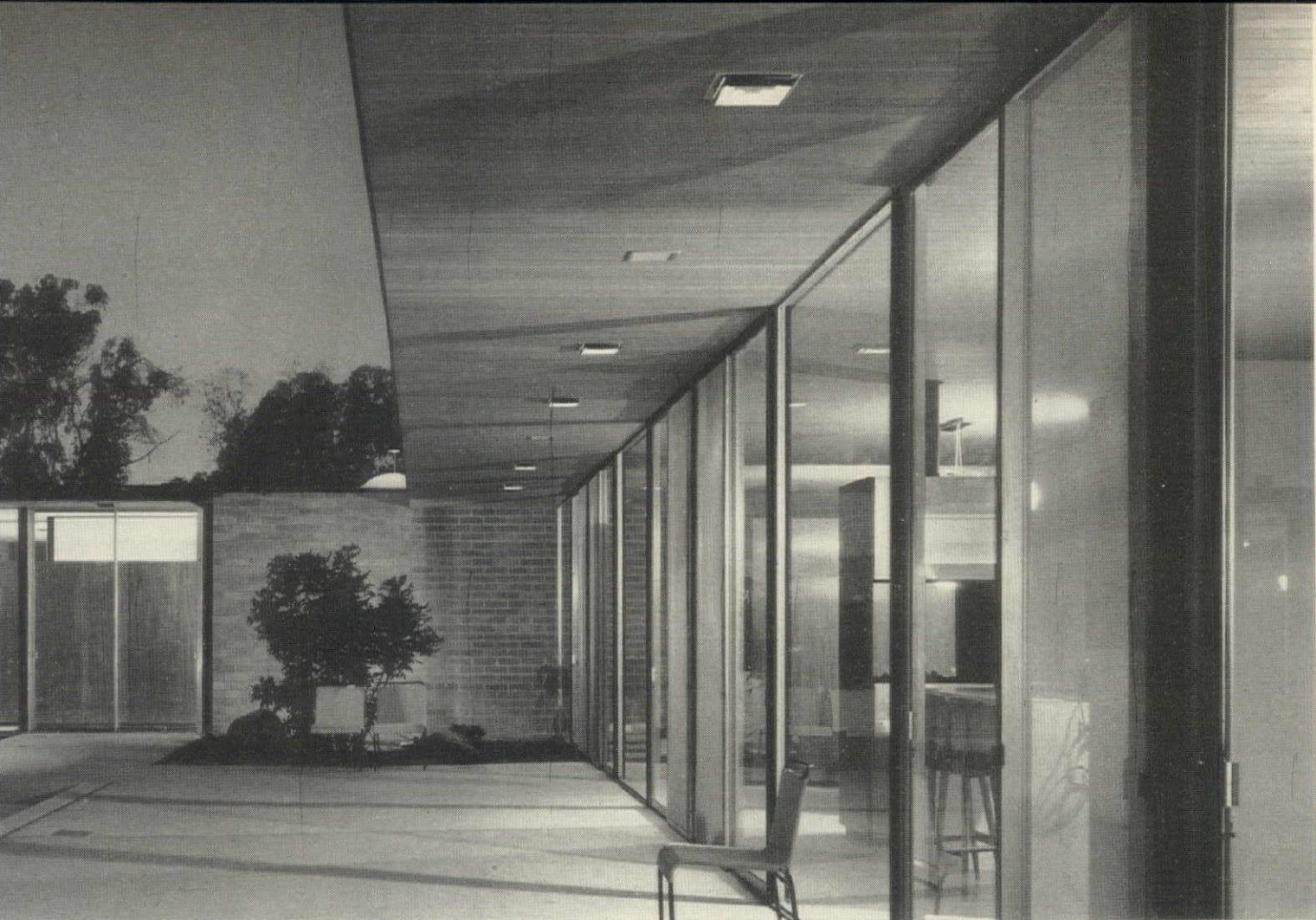
Window walls, framed in aluminum and set between 4" steel columns, line the open sides of living area, right, and bedrooms, left
