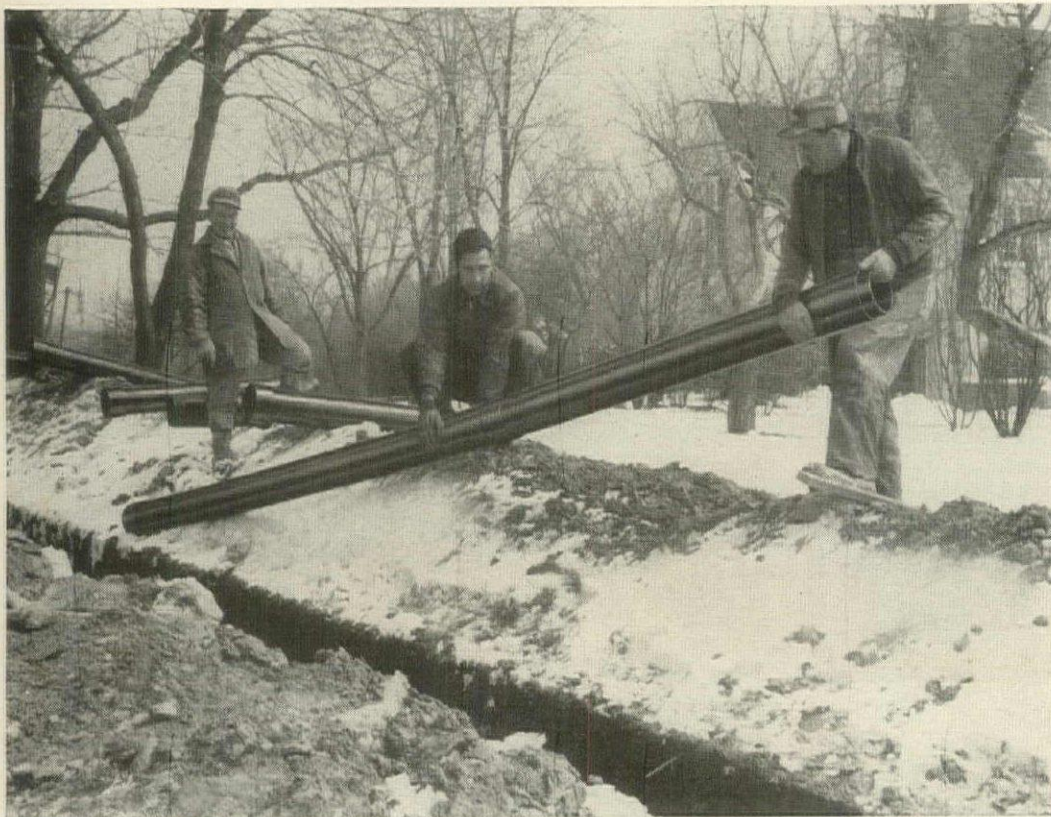
LONG LENGTHS are assembled on the ground, lowered into trench, and tapped into position to make a root-proof, watertight joint. Easy to handle, quickly installed. Only Perma-Line is available in 5, 8, and 10-foot lengths.
