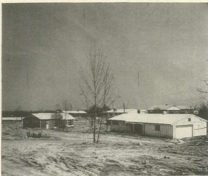
Houses are turned on site to get maximum privacy, and each house is placed on the lot that suits it best, as the site plan at the top of the page and the photo above indicate. Trees are saved whenever possible.
