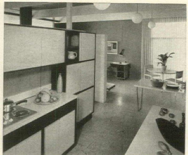
Kitchen cabinets have sliding Masonite doors sprayed with various shades of two-tone washable paint.
