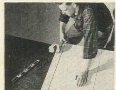
Irregular surfaces or out of plumb walls are no problem at all. Fillers are furnished which can be quickly and easily scribed. Fillers can be cut on the job with tin snips.
