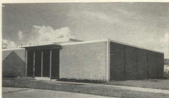
Steel frame house in Houston Parade of Homes, 1955. Burdett Keeland, architect. Buck King, builder. Brick walls are treated as large panel inserts set between exposed steel columns.
