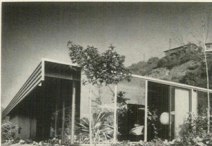
Glass-walled house has vertical eave which shades glass from west sun until 5 p.m. House on 4-acre site has fine view of mountains.
