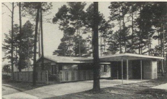
Conventional house by J&B Builders, Houston, is actually built around a new stud-like steel framing system.
