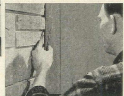
The photo above illustrates how easily a GENEVA cabinet can be fitted to even a brick wall. Filler can be accurately scribed to give tailored appearance.
