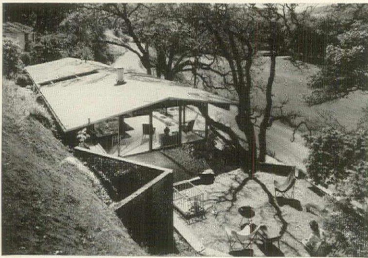
Nestling on hillside, this 1,100 sq. ft. house is protected from possible earth slide by 6' concrete wall covered by redwood fence.
