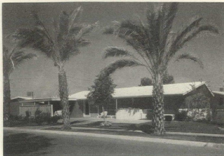
Carport has fenced side to street which helps hide unsightly objects. Sun-bouncing white roofs are Phoenix standard.
