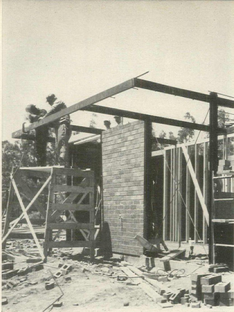
Steel frame takes inserts of block, wood or glass just like panels
