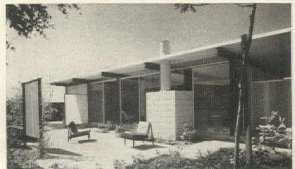
Metal and glass house by builder Joe Eichler openly capitalizes on its exposed steel roof deck and framing.
