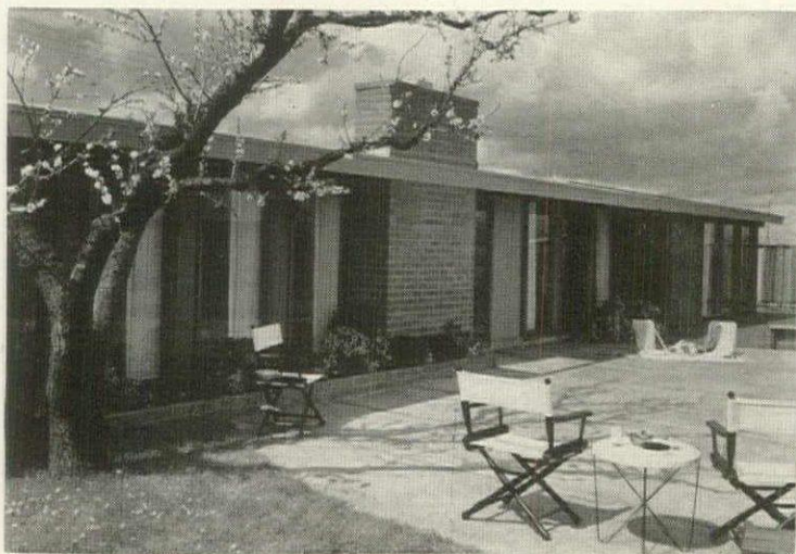
Trees in this old cherry and apricot orchard were saved whenever possible. Wide overhang (on all four sides) makes house seem larger.
